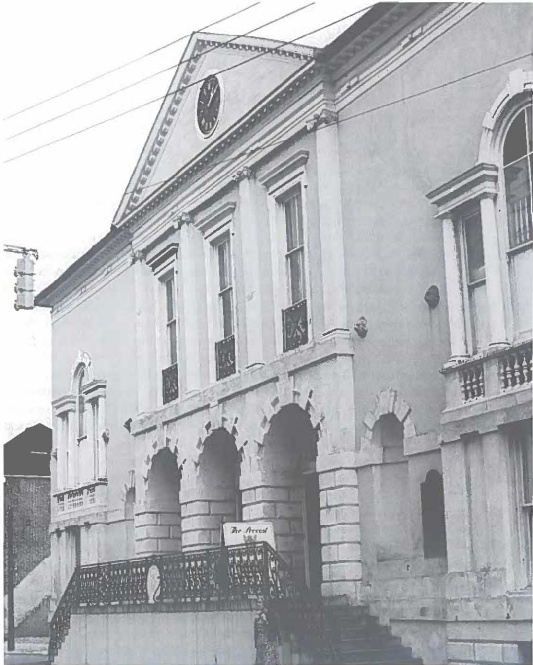
Exchange Building, Charleston. Built between 1767 and 1771, the Exchange was the site of an anti-tea mass meeting on 3 December 1773. British troops were quartered here after the fall of Charlestown, and Colonel Isaac Hayne was imprisoned in the dungeon before being hanged as a traitor on 4 August 1781. In 1780 the convention to ratify the Constitution met here, and in 1791 President George Washington viewed a parade in his honor from its western porch. State Historic Preservation Office. SCDAH.
