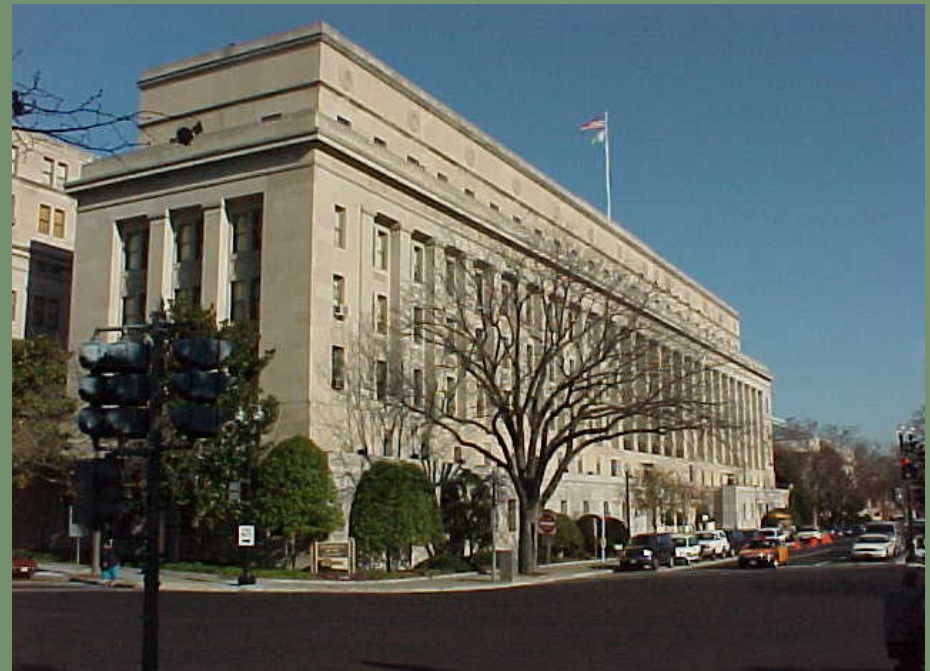
1849 C Street, NW Washington DC; Silver LEED EB
