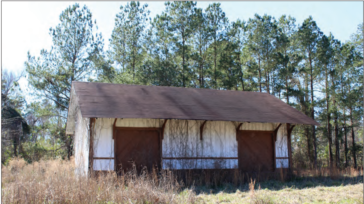
A. Train Depot, East Elevation
