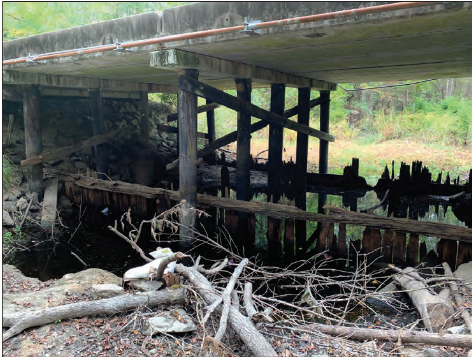
A. Oblique View, Facing Northwest
