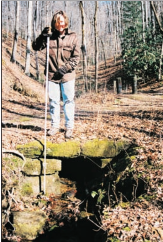
A. Stone Culvert. Looking North.
