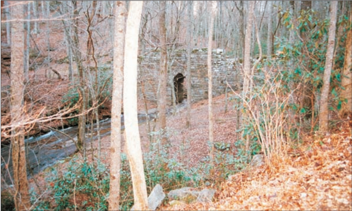
A Setting of Poinsett Bridge showing the narrow valley and steep valley walls. Looking upstream (east).
