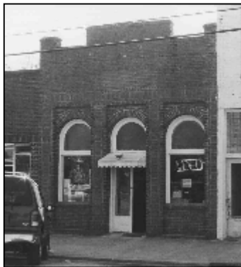
Figure 46. Old Bank Building (Site 0377)
