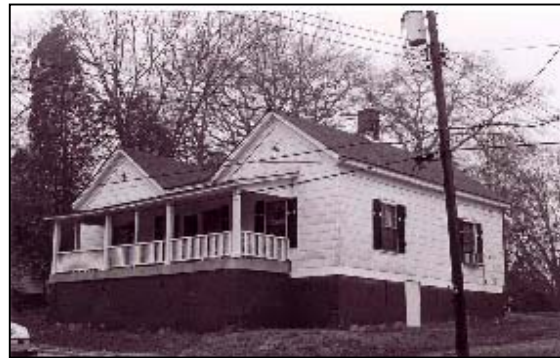
Figure 76. Laurens Cotton Mill Employee Housing Style 4 (Site 0733)
