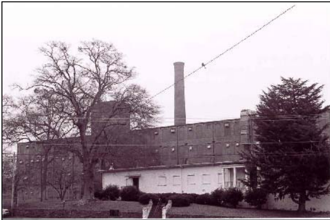
Figure 78. Laurens Cotton Mill-view showing the western facade.
