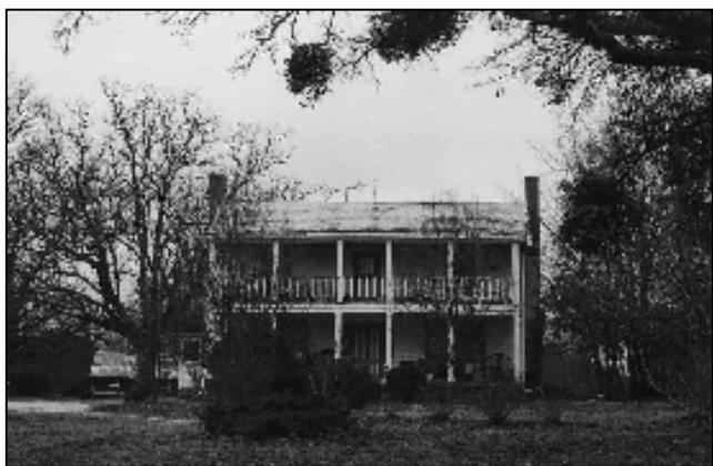
Figure 18. Hellams House (Site 0210)
