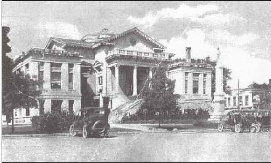
Figure 58. Laurens County Courthouse ca. 1920
