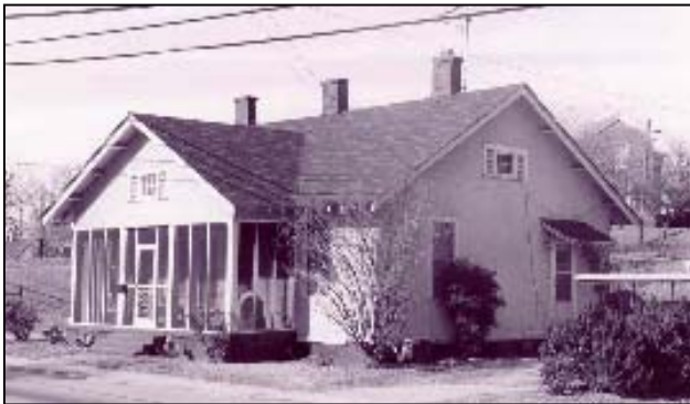
Figure 75. Laurens Cotton Mill Employee Housing Style 3 (Site 1477)
