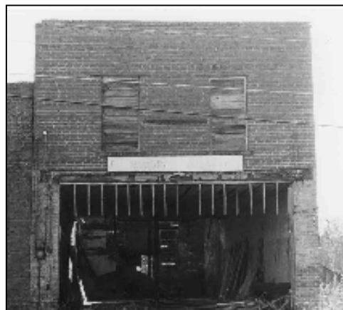
Figure 38. E.F. Golding General Merchandise Store (Site 0342)
