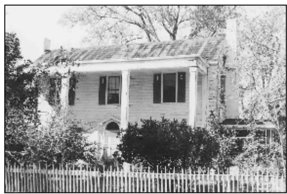
Figure 17. L. Blakely House (Site 0314)
