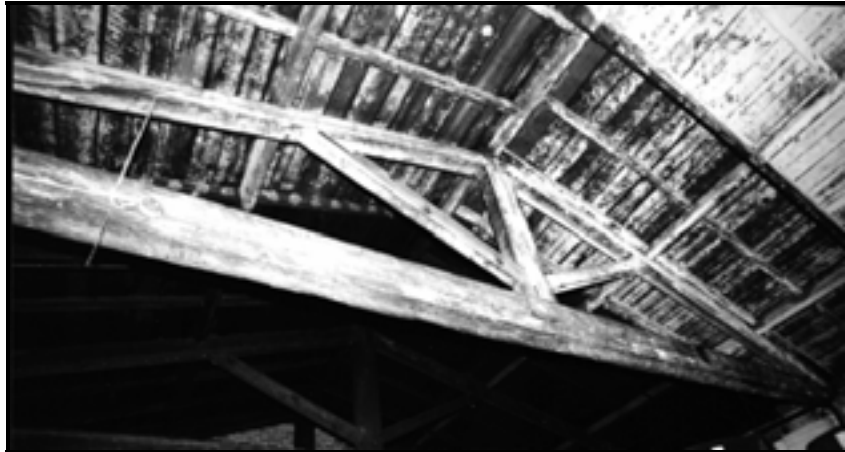
Figure 8. Inside view of Southern Railway Freight Depot, Site 093 0259.
