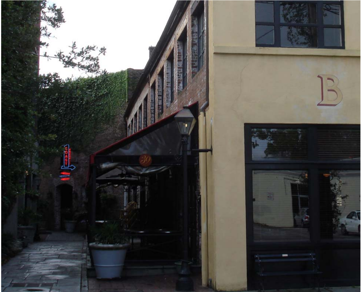
Alley adjacent to 39 John Street
