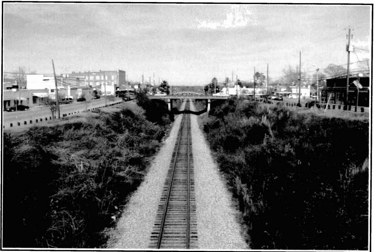
Figure 2 - Present View of St. Matthews Railroad Cut
