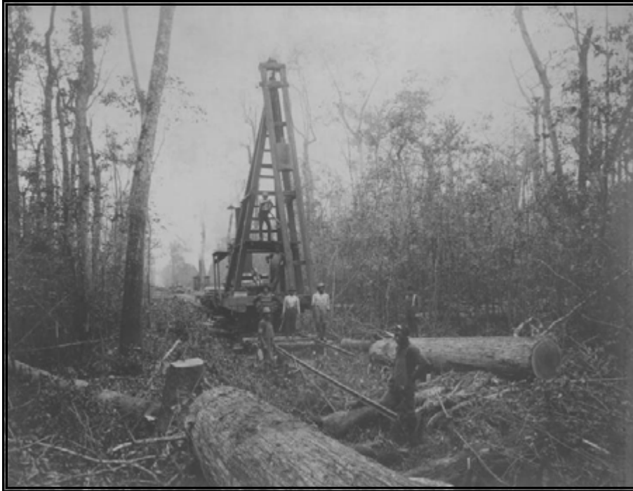
Figure 76. Crew laying track for the tram line (GCDL).
