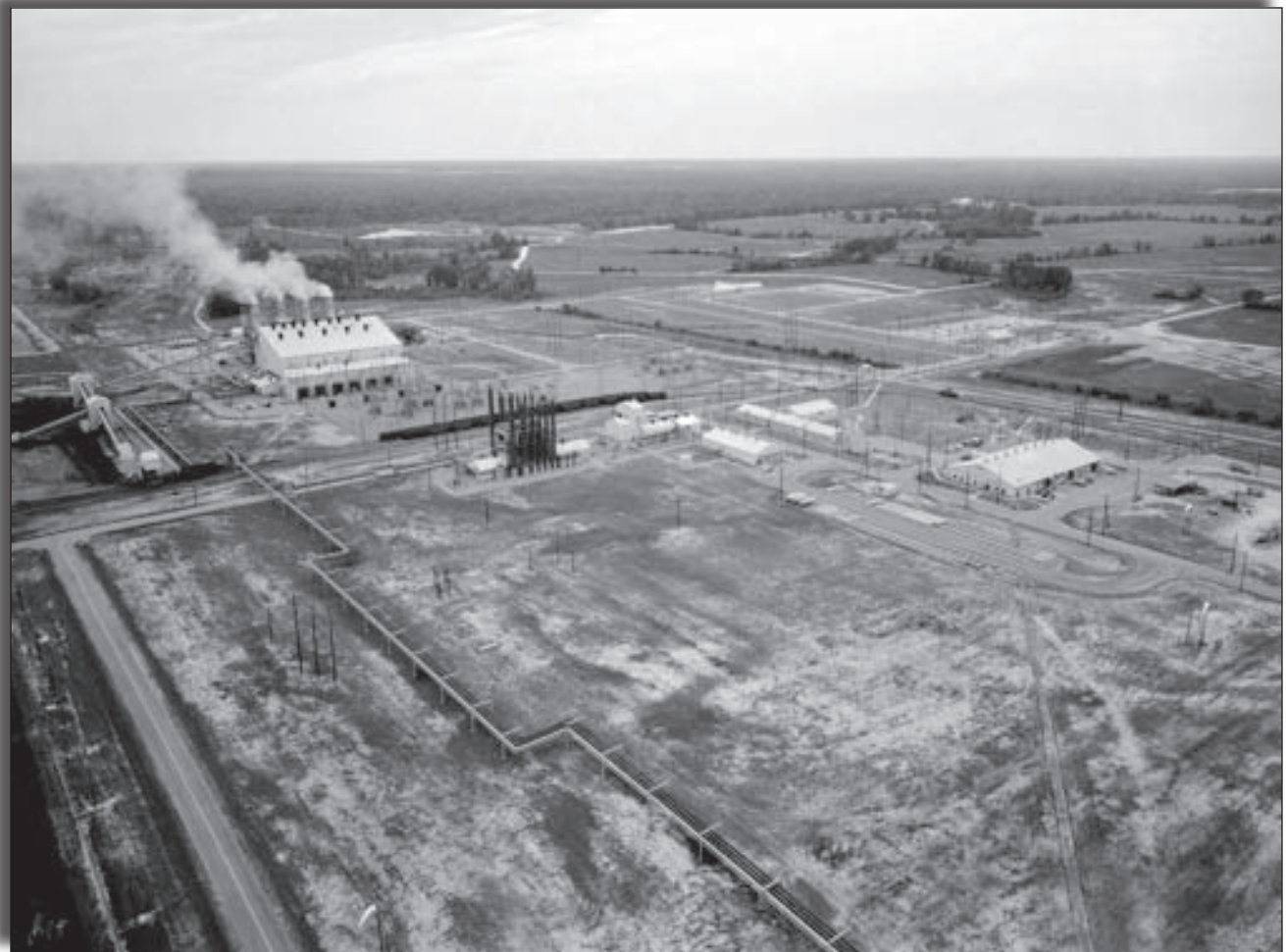
Aerial View of 484-D Powerhouse, April 16, 1956, SRS Negative 3410-29
