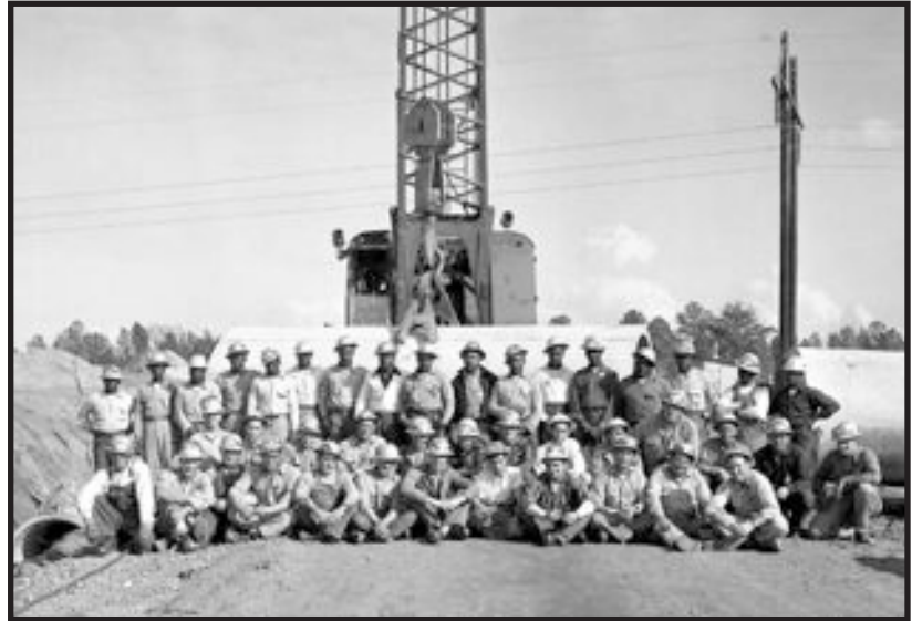
Pipe Laying Crew, January 15, 1953, SRS Negative M-1830-02
