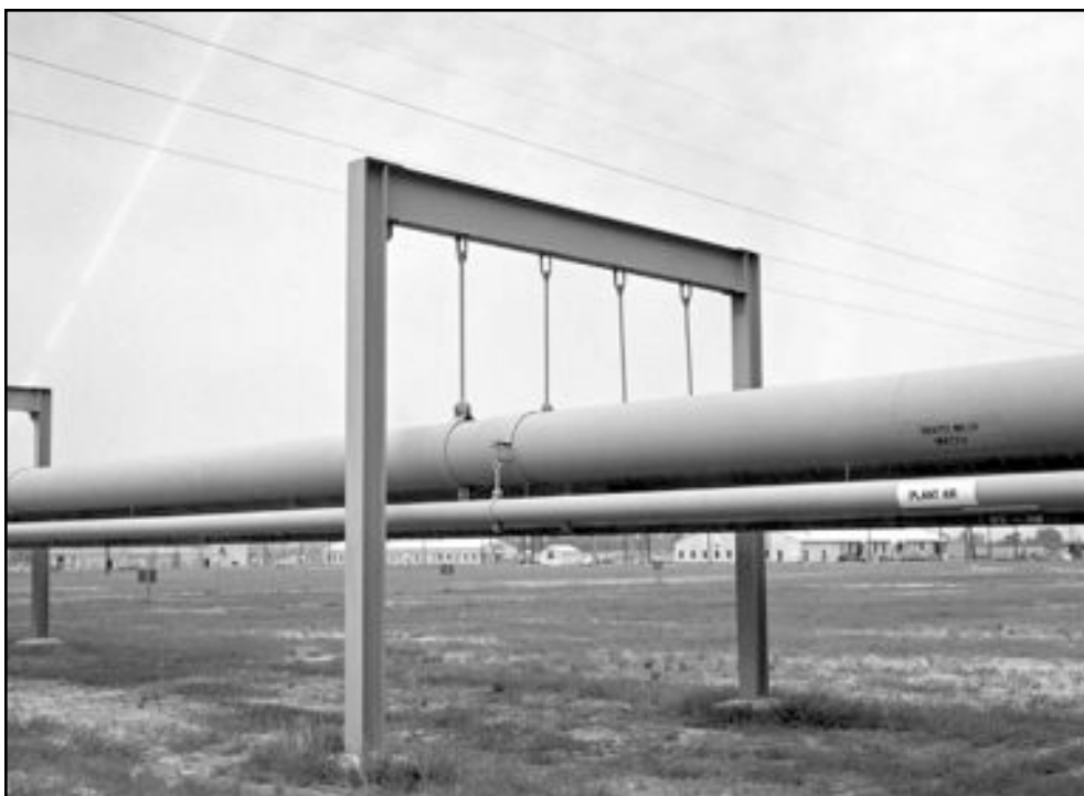
Pipe Supports in D-Area, August 13, 1953, SRS Negative 4-515-04
