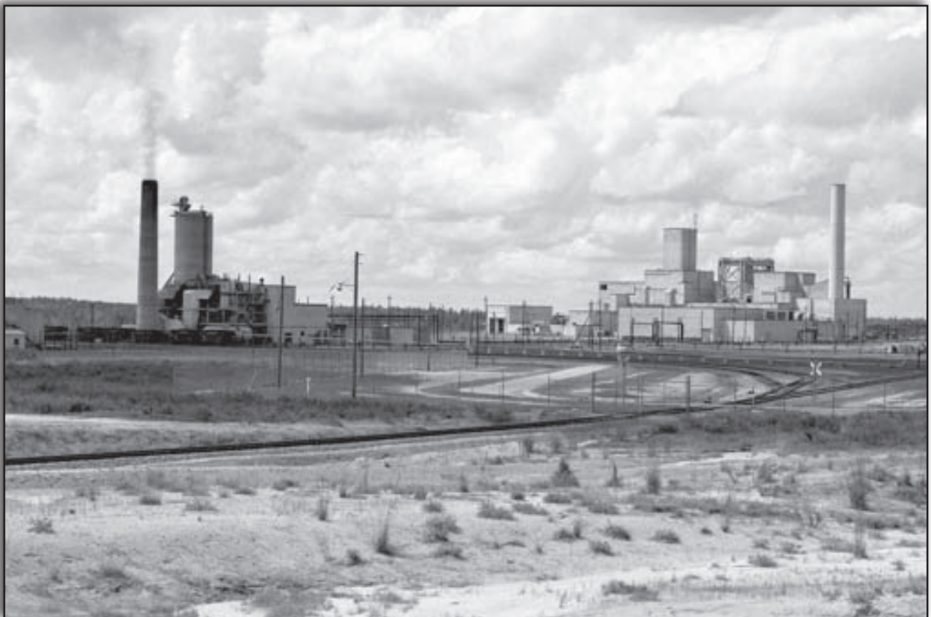
184-C Boiler House (left) and C-Area Reactor (right), July 27, 1959, SRS Negative DPSPF-6098-15
