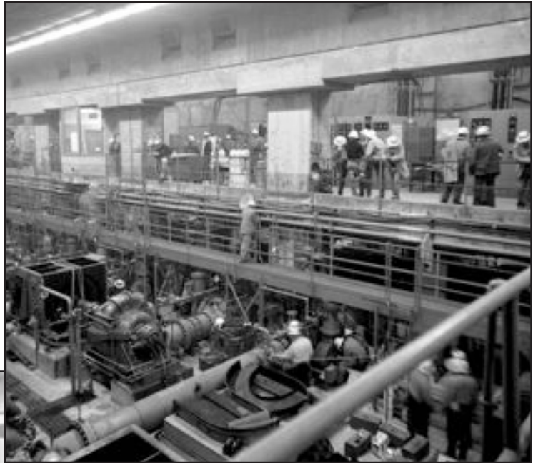
INTERIOR VIEW OF PUMP HOUSE, CLEAN-UP OPERATION SHOWING BOTTOM LEVEL, DECEMBER 15, 1954
