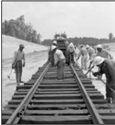
Railroad Construction Near Dunbarton, May 31, 1951, SRS Negative M-132-2
