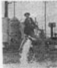
John Fahn, one of a group of water engineers, is shown making a periodic performance test on a deep well pump.
