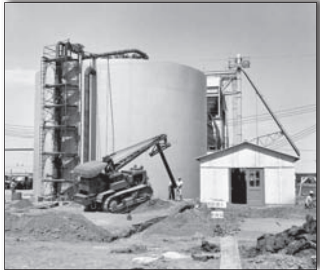
782-A Reservoir Construction, August 28, 1952, SRS Negative 7-417
