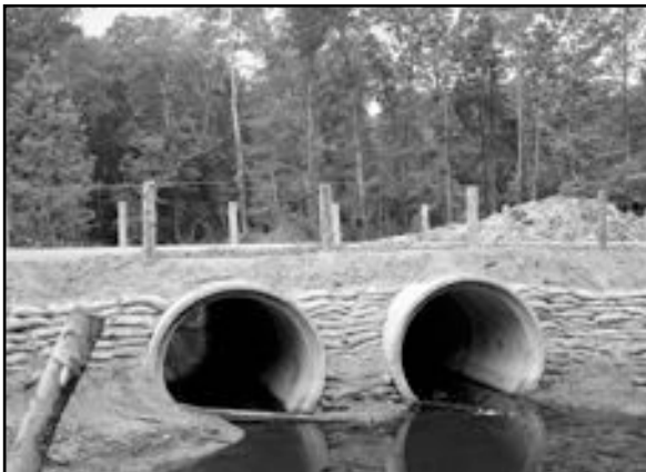
Bridge and Culvert at Four Mile Creek, May 31, 1951, SRS Negative M-146
