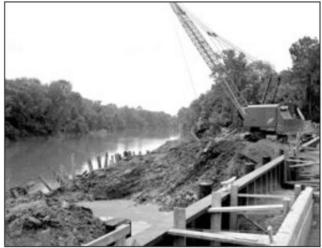
Construction of Savannah River Boat Landing, May 31, 1952, SRS Negative M-931-01
