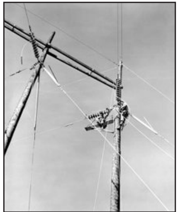
Electrical Linemen in 300/700 Area, March 7, 1952, SRS Negative M-609
