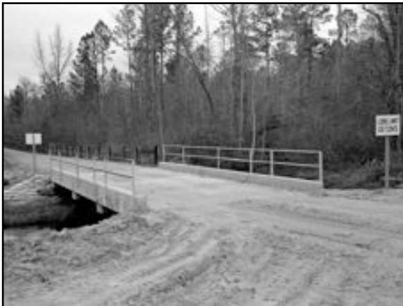
Example of Pre-fab Bridge at SRP, January 4, 1957, SRS Negative 4022-02
