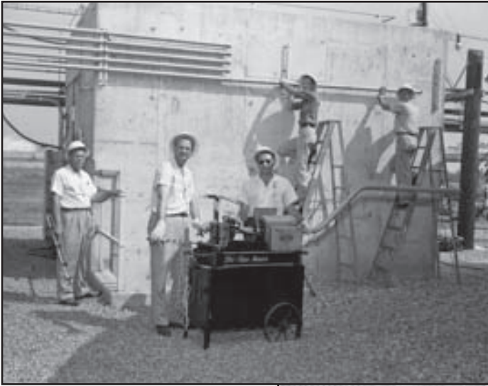
Electrical Crew in C-Area, June 6, 1958, SRS Negative DPSPF-5230-1
