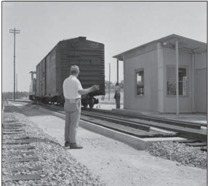
Building 608-G (Track Scale House), East Elevation, September 10, 1954, SRS Negative DPSPF-1785-5
