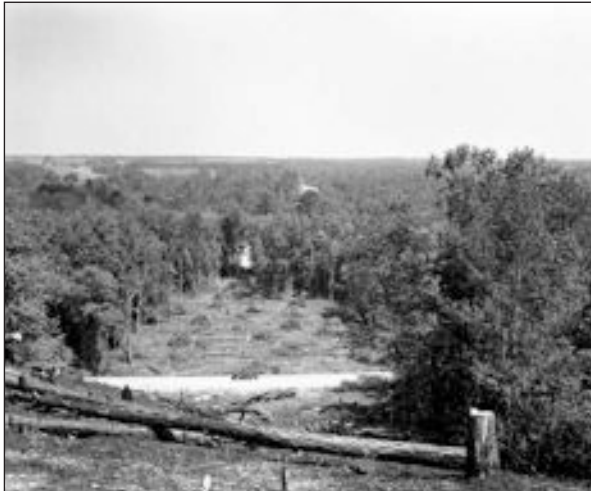
New Road Cut at Three Runs Bridge, View Looking West, July 9, 1951, SRS Negative M-187
