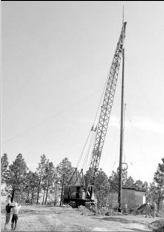
Radio Pole Erection, March 28, 1957, SRS Negative 4334-09
