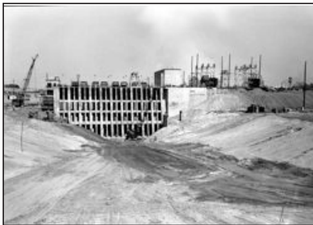
681-3G Pump House Intake, March 28, 1953, SRS Negative 6-249-02
