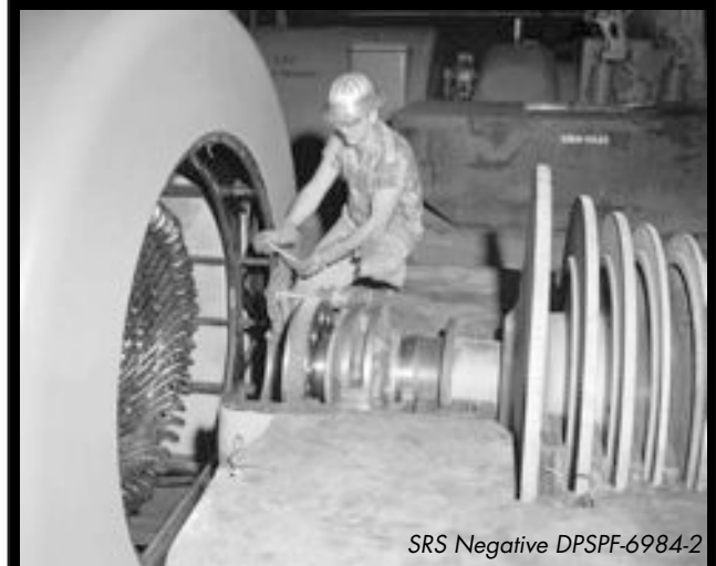
TURNING DEVICE FOR #3 TURBINE IN 484-D POWERHOUSE, OCTOBER 4, 1960
