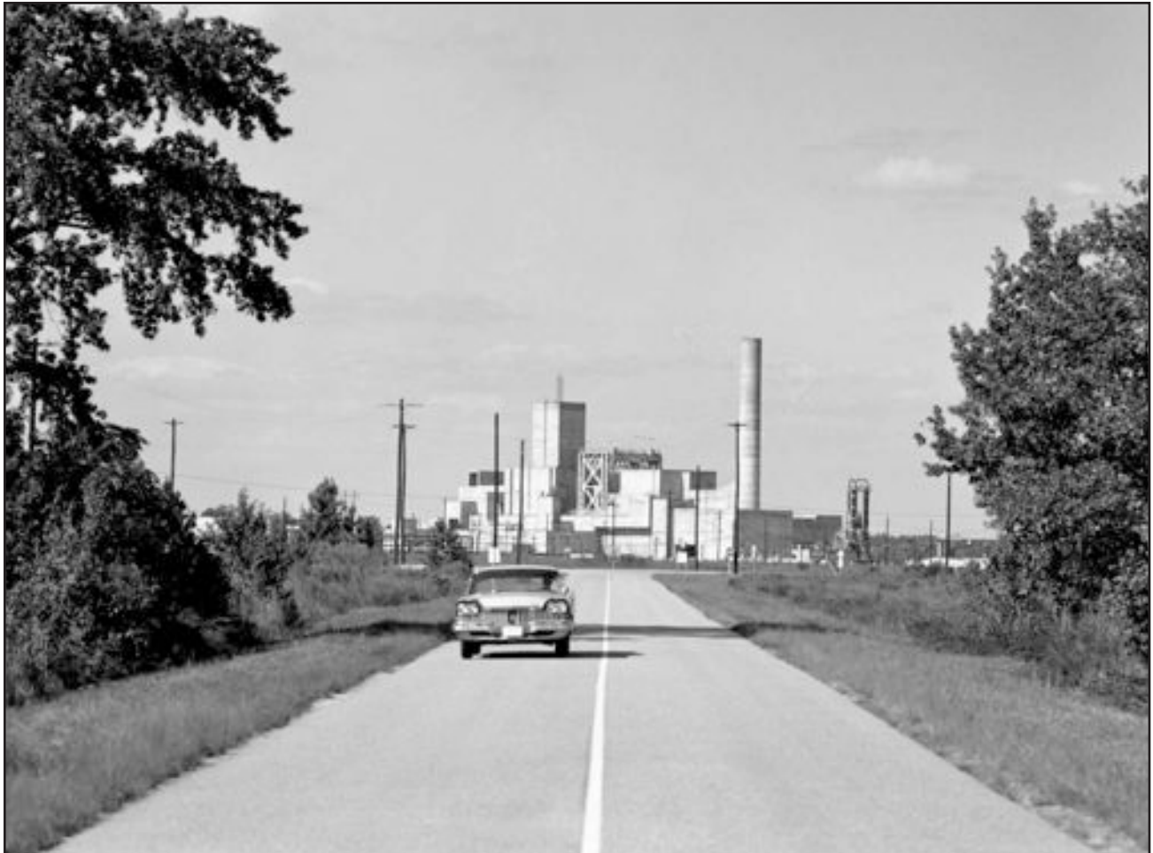
Example of Primary Road Near R Reactor, September 23, 1959, SRS Negative DPSPF-6240-3
