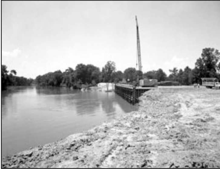
Construction of Savannah River Boat Dock, June 25, 1952, SRS Negative M-1045-01
