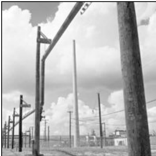
Steamlines and Pipe Supports, July 11, 1955, SRS Negative DPSPF-2731-4
