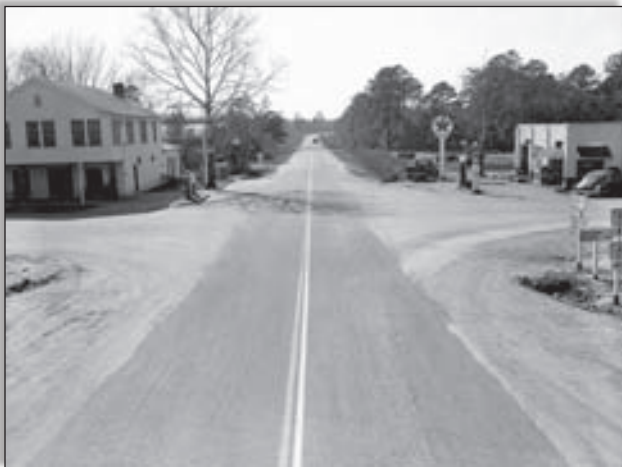
Highway 64 at Dunbarton, View Looking Northwest, February 15, 1952, SRS Negative M-565
