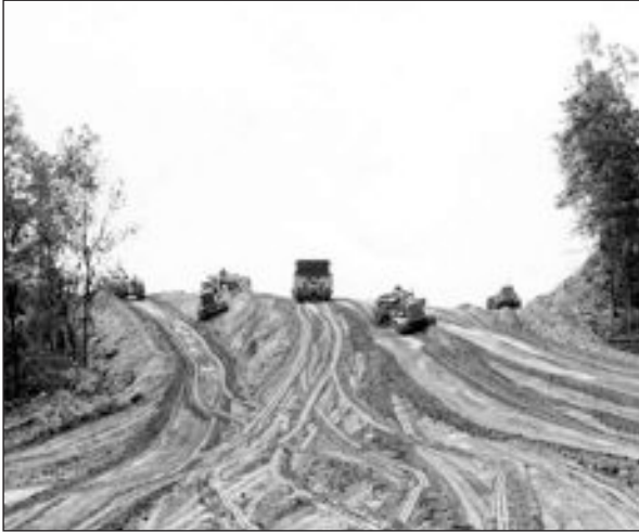
New Road Cut, Three Runs Bridge, July 26, 1951, SRS Negative M-213-4
