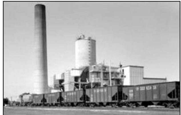
Railcars in Front of Powerhouse, February 24, 1959, SRS Negative DPSPF-5773-2
