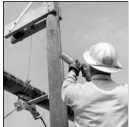
Insect Spraying Under Steam Pipe Supports, August 28, 1957, SRS Negative DPSPF-4597-5
