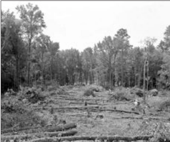
Initial Road Survey, New Road (Road C) to Three Runs Bridge, June 28, 1951, SRS Negative M-168
