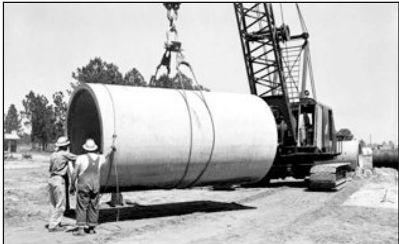
84" Pipeline Segment, April 3, 1952, SRS Negative DPESF-712-09
