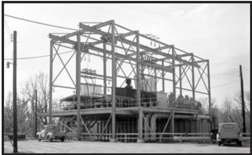
681-5G Under Construction, January 14, 1953, SRS Negative 6-237
