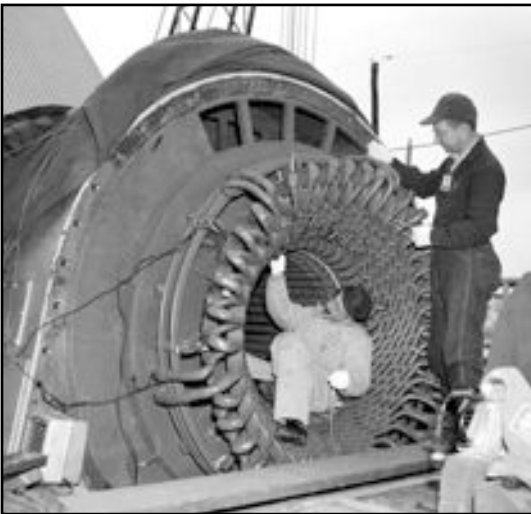
Generator Repairs, January 14, 1958, SRS Negative 4934-4
