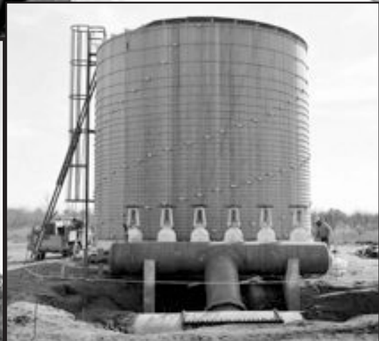
(TOP) Testing for Water Hammer on the 901 Large River Water Pipelines (Underground Water Pipes), December 1953, SRS Negative M-3193-10
