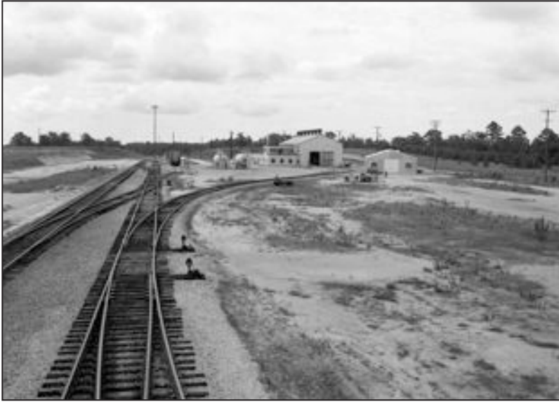
Railroad Classification Yard, View Looking South, July 8, 1956, SRS Negative DPSPF-5218-10
