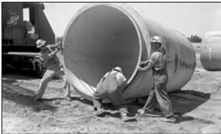
Laying Water Lines, April 3, 1952, SRS Negative DPESF-712-08
