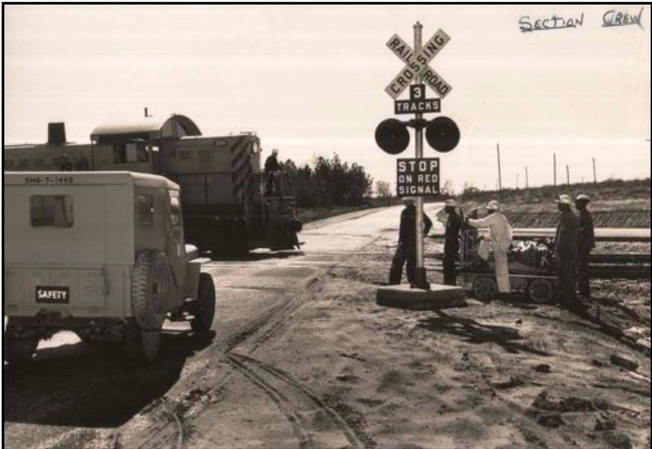
Section Crew Performing Maintenance on Intersection Signal, March 3, 1952, Photograph Courtesy William Hinson
