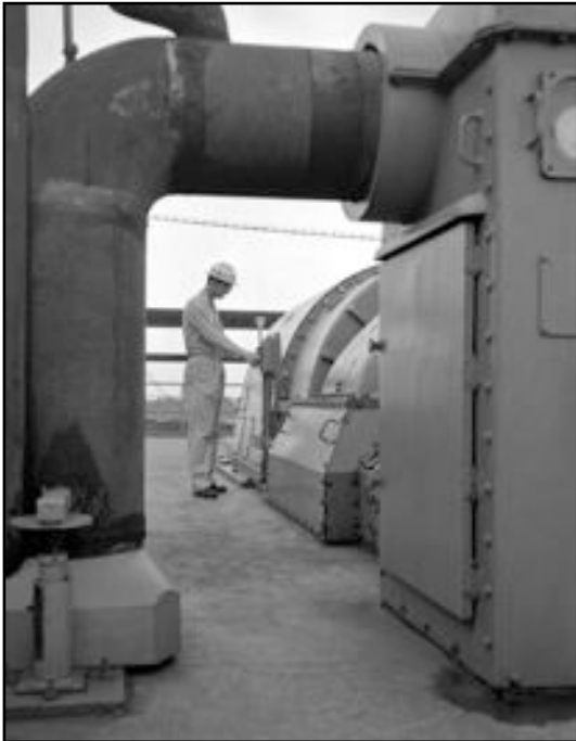
Generator Housing in 184-K Powerhouse, December 10, 1956, SRS Negative 3943-20
