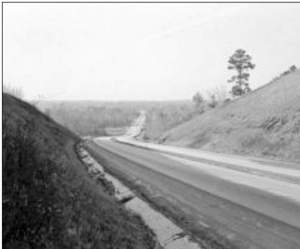
Four Lane Road After Completion, January 27, 1958, SRS Negative 4967-32
