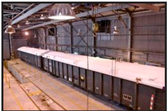
Interior View of Building 618-G, July 2009, SRS Negative 0901190020
