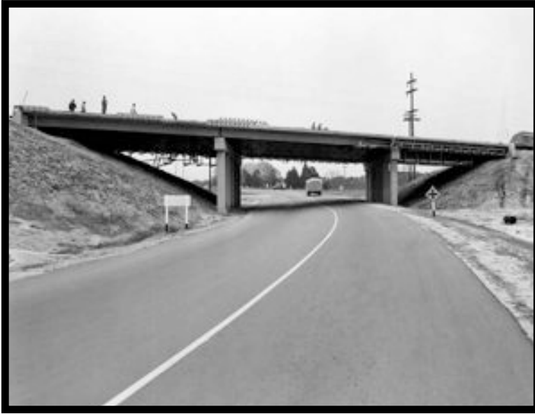
781 Beech Island Overpass, March 28, 1952, SRS Negative M-687B
