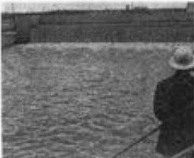
Process raw water pumps take their suction from this reservoir for supplying D Area needs. Water comes from the river pumping stations.
