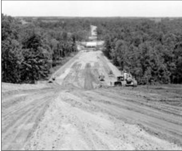
New Road Cut, Three Runs Bridge, July 26, 1951, SRS Negative M-213-03
