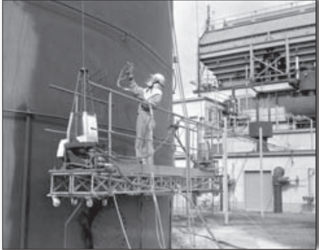
Finishing the Exterior of 782-A Reservoir, date unknown, SRS Negative DPSPF-6513-1
