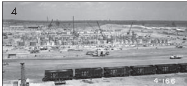
TOWER CONSTRUCTION VIEWS: 1. Building Sign; 2. Constructing a reinforced concrete foundation for tower platforms; 3. Construction of concrete pedestals for tower units; 4. GS Unit area showing pedestals in various stages of completion, train in forefront; 5. Stiff legged derek lifting first tower; 6. Derek completing tower row; 7. Tower being elevated; 8. Tower in place; 9. Units in place.
