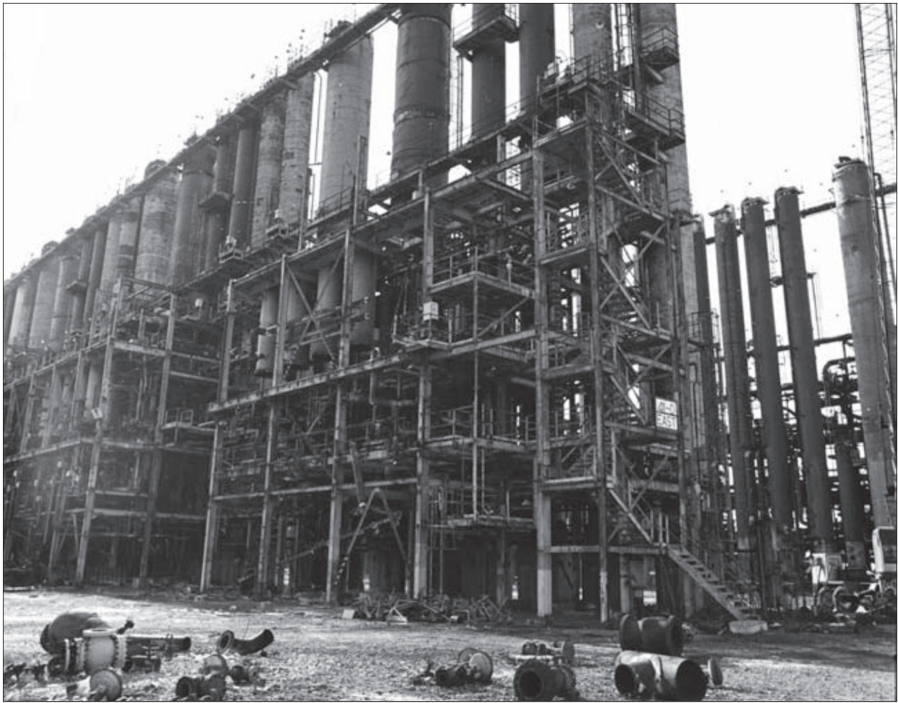
(Above and Below) Details showing early dismantlement and aerial view of 400/D Area with 411-D, 412-D removed. Courtesy of SRS Archives, negatives 16597-14 and 34268-18.
