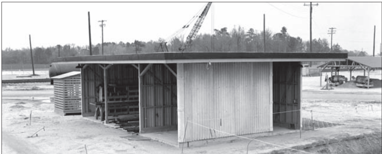
Building 711-D, Pipe Storage. Historic view, 1952. Courtesy of SRS Archives, negative 4-346-9.
