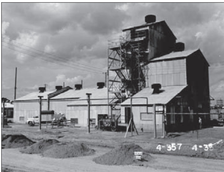
Building 421-D, Finishing Building. Courtesy of SRS Archives, negative 4-357-2.
