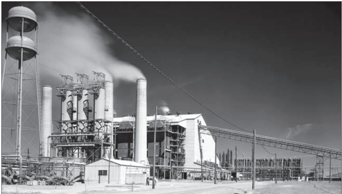
Power House after Completion. Courtesy of SRS Archives, Negative No. 3142-004.
