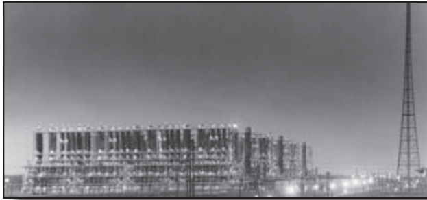
411-413 GS Units and Flare Tower
