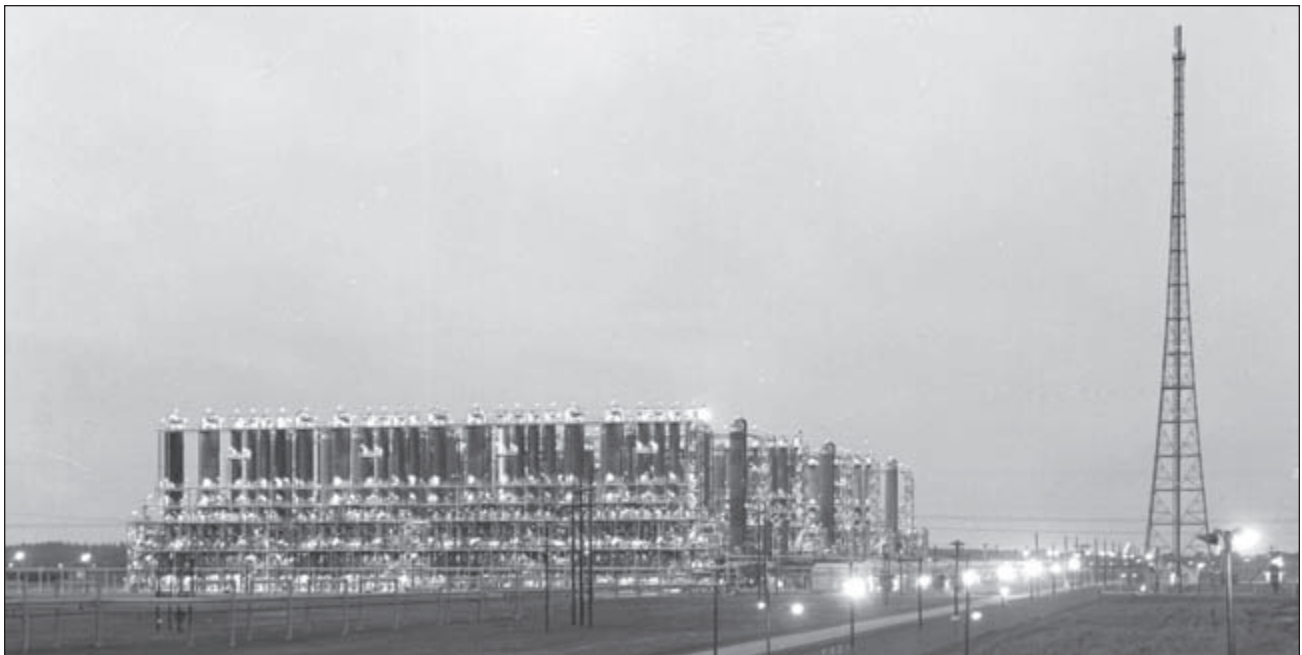
Night time view of 400/D Area , circa 1953. Courtesy of SRS Archives, negative 3391-003.
