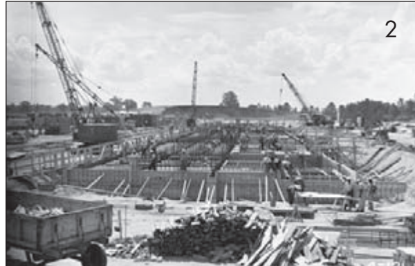
TOWER CONSTRUCTION VIEWS: 1. Building Sign; 2. Constructing a reinforced concrete foundation for tower platforms; 3. Construction of concrete pedestals for tower units; 4. GS Unit area showing pedestals in various stages of completion, train in forefront; 5. Stiff legged derek lifting first tower; 6. Derek completing tower row; 7. Tower being elevated; 8. Tower in place; 9. Units in place.
