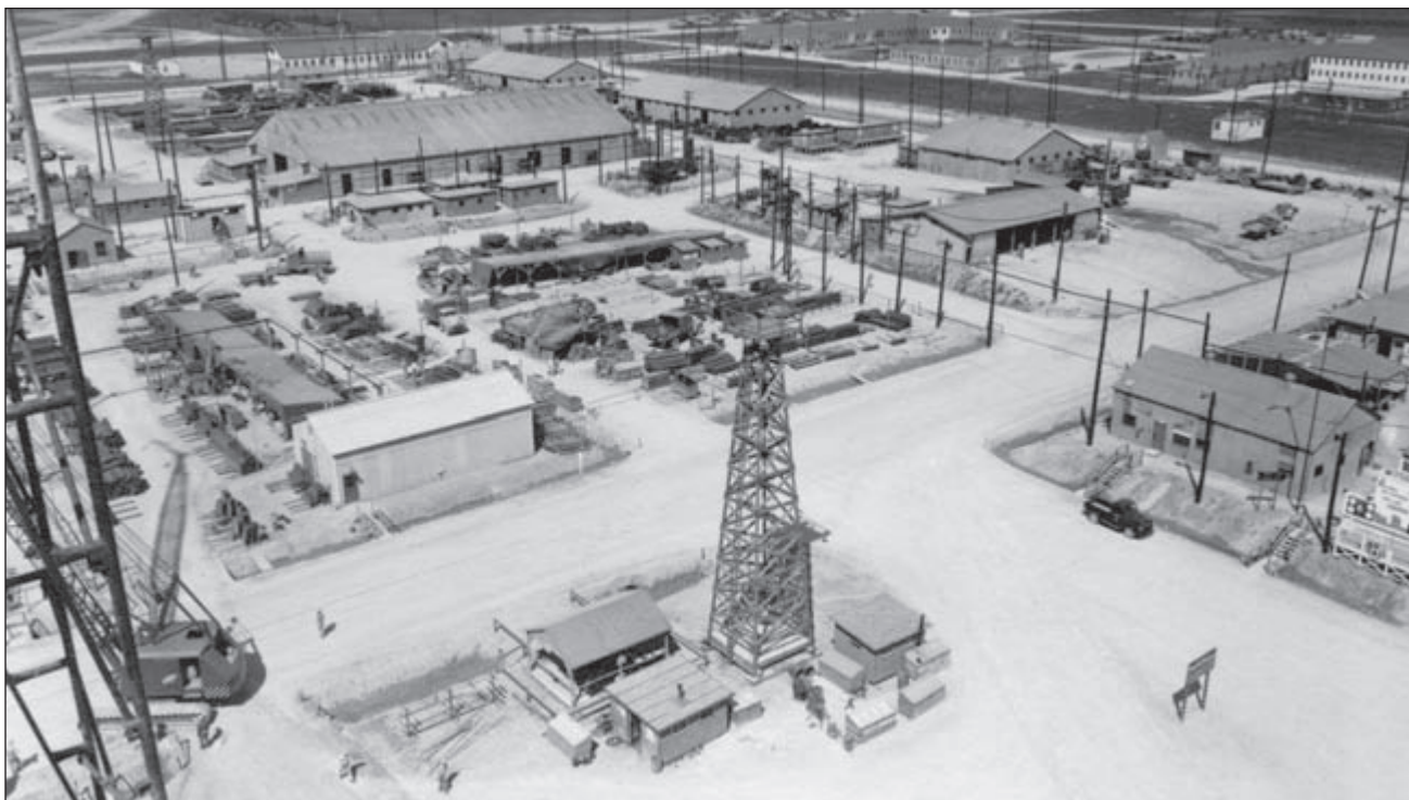
Aerial of Dana Plant.
