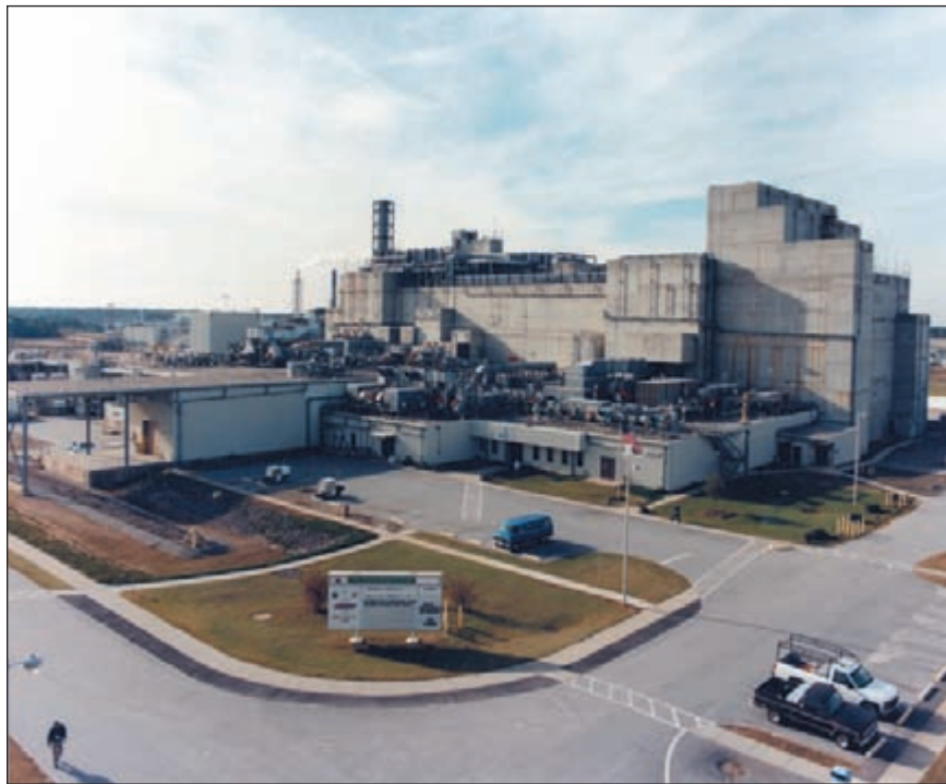
Aerial View of DWPF Building 1977. Courtesy of SRS Archives, Negative 97-1527-1.
