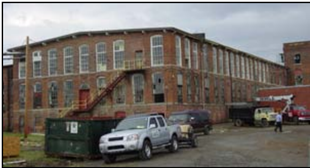
Highland Park Mill (NR 1992), renovations in 2004
