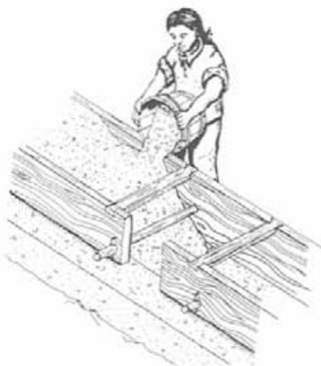
Tabby boxes--little more than planks held together with wooden pins and pegs--served as molds for the poured tabby mixture. A 19th-century expert on tabby found that a slave could mix and mold 120 cubic feet of tabby per week.
