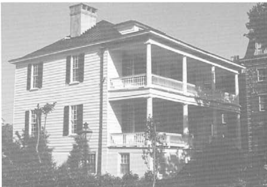
A piece of old Dorchester in Charleston? That's what the author of a letter to the Charleston News and Courier claimed in 1959. The house was said to have been built in Dorchester and then dismantled and rebuilt at its present location in Charleston on the corner of Smith and Wentworth streets. The double porch is a later addition.
