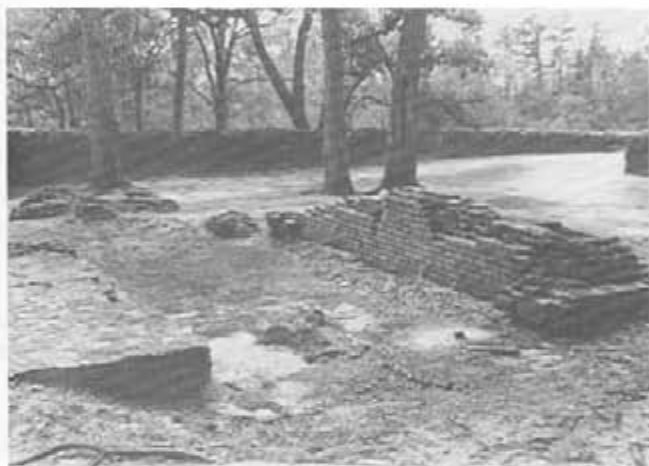
Nineteenth-century scavengers removed bricks from the powder magazine for use in the construction of the Presbyterian parsonage in Summerville. The remnants of the magazine were uncovered by archaeologists in the summer of 1973.
