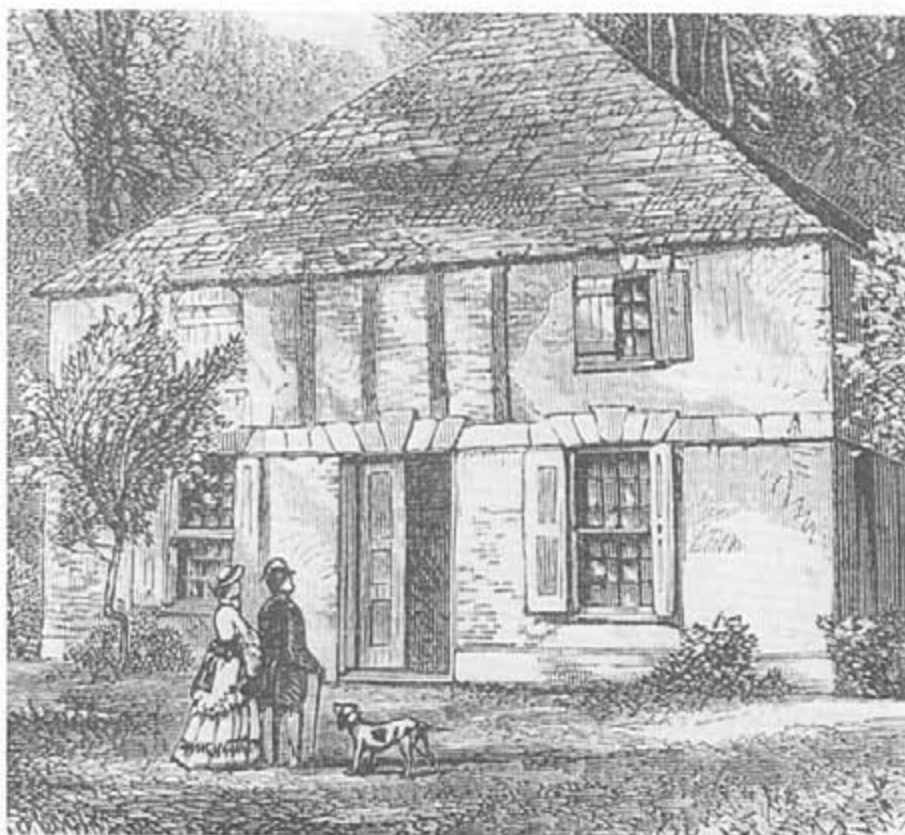
Pictured here in 1875, the Congregational meeting house served Dorchester's Puritan settlers for over 50 years. A new congregation renovated the old building in 1794 and used it off and on into the next century. An earthquake in 1886 left the structure a ruined shell.
