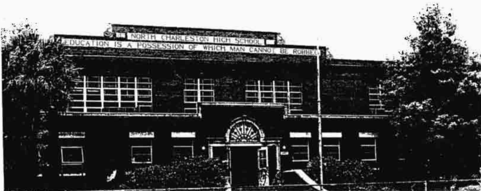
North Charleston High School Just Before Demolition (1983) File Photo, Courtesy of Post-Courier Newspaper
