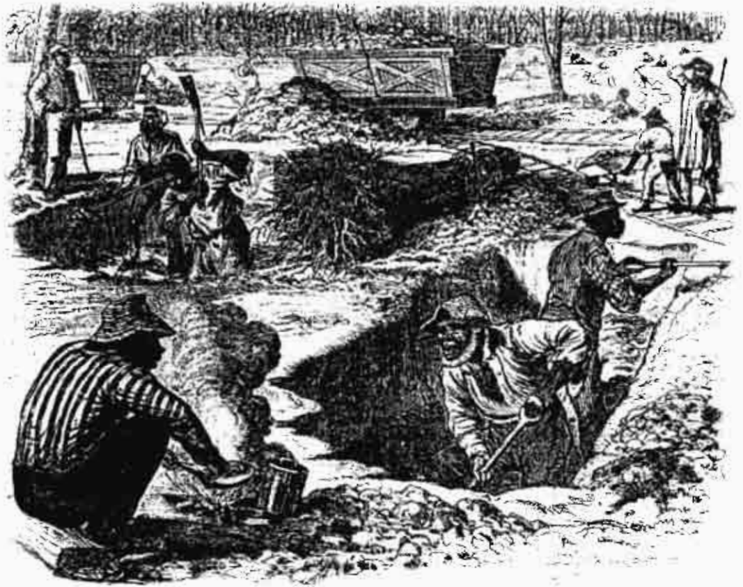
Digging in the phosphate pits.
