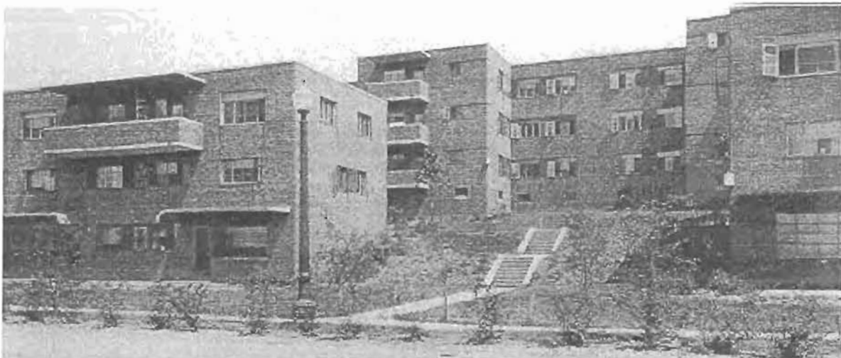
Figure 7 - Representative buildings at Lakeview Terrace featuring brick construction, flat roofs, casement windows, and stripped architectural details. (Short and Brown, Public Buildings , 1939)
