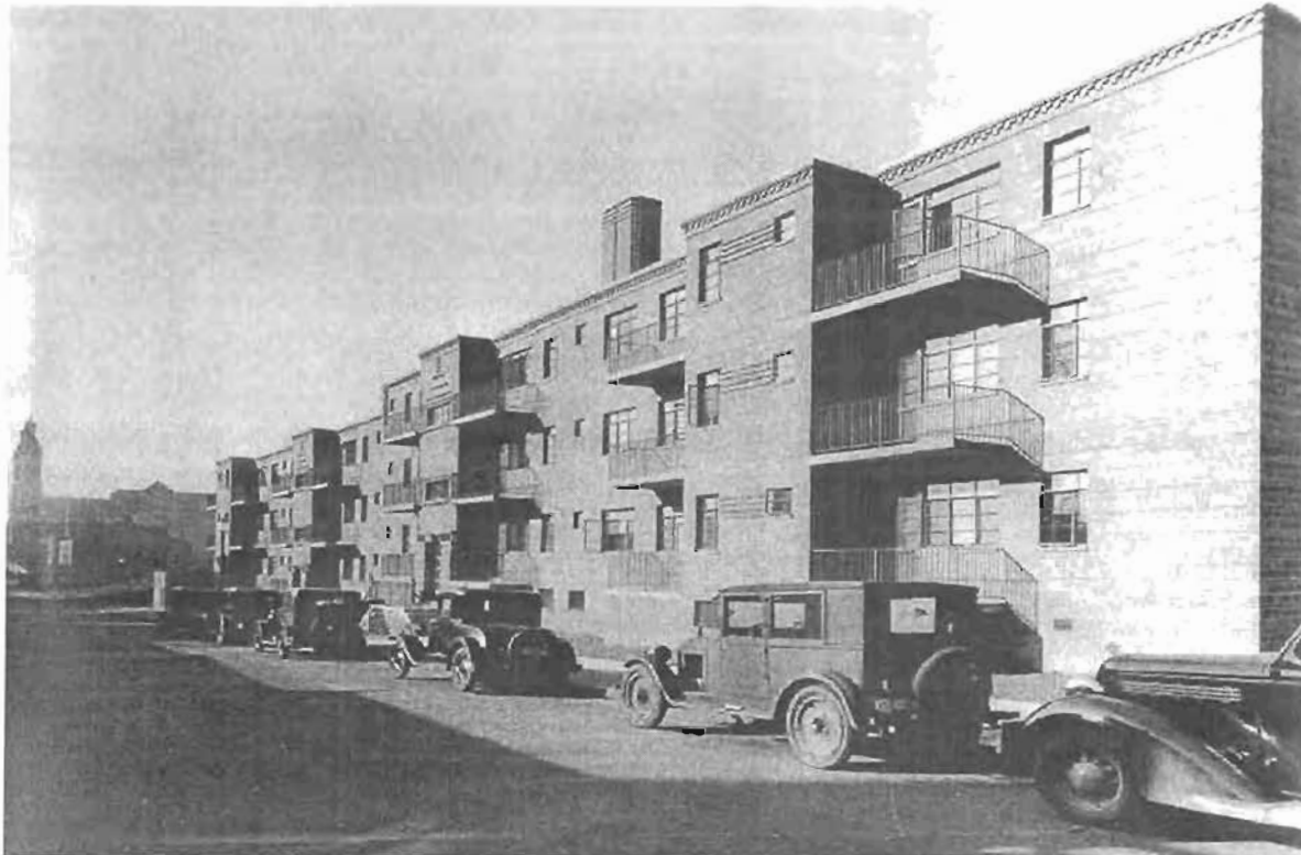
Figure 2 - A representative building at Neighborhood Gardens in St. Louis, Missouri, a PWA limited-dividend public housing project completed in 1935. The 252-unit complex's three-story brick and concrete buildings featured flat roofs and International Style architectural details, common characteristics of the era's early public housing. (National Register of Historic Places Nomination, 1985)
