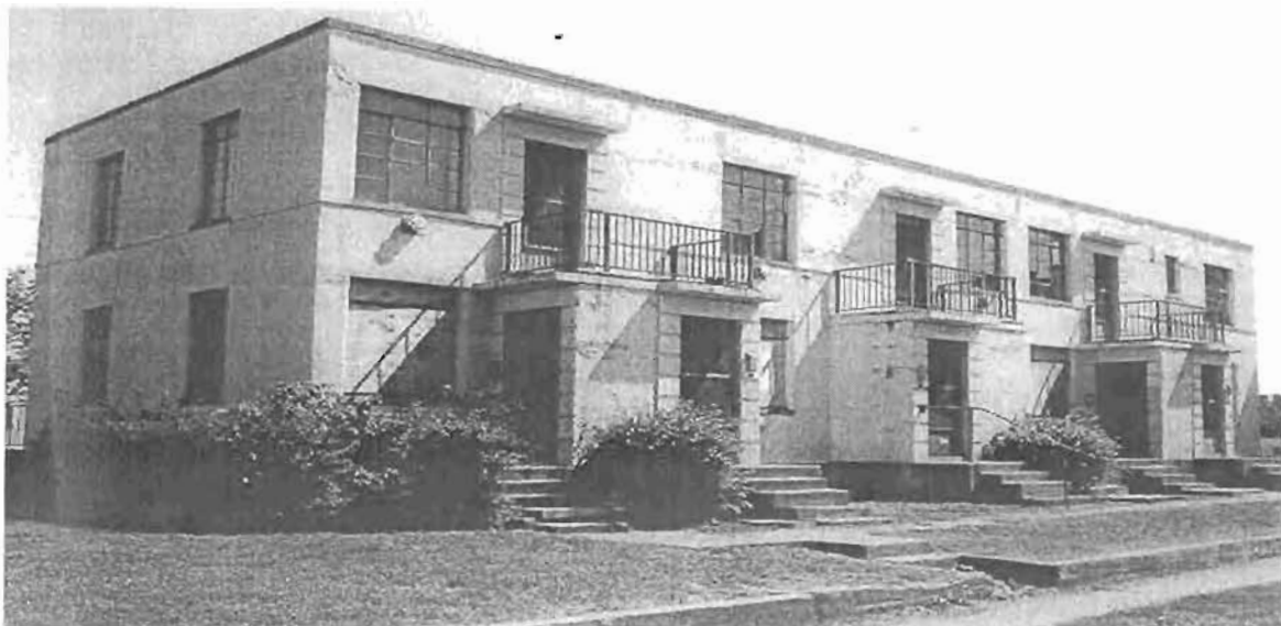
Figure 16 - A contemporary view of an individual building in Cedar Springs showing subsequent deterioration. (National Register of Historic Places Nomination, 1991)
