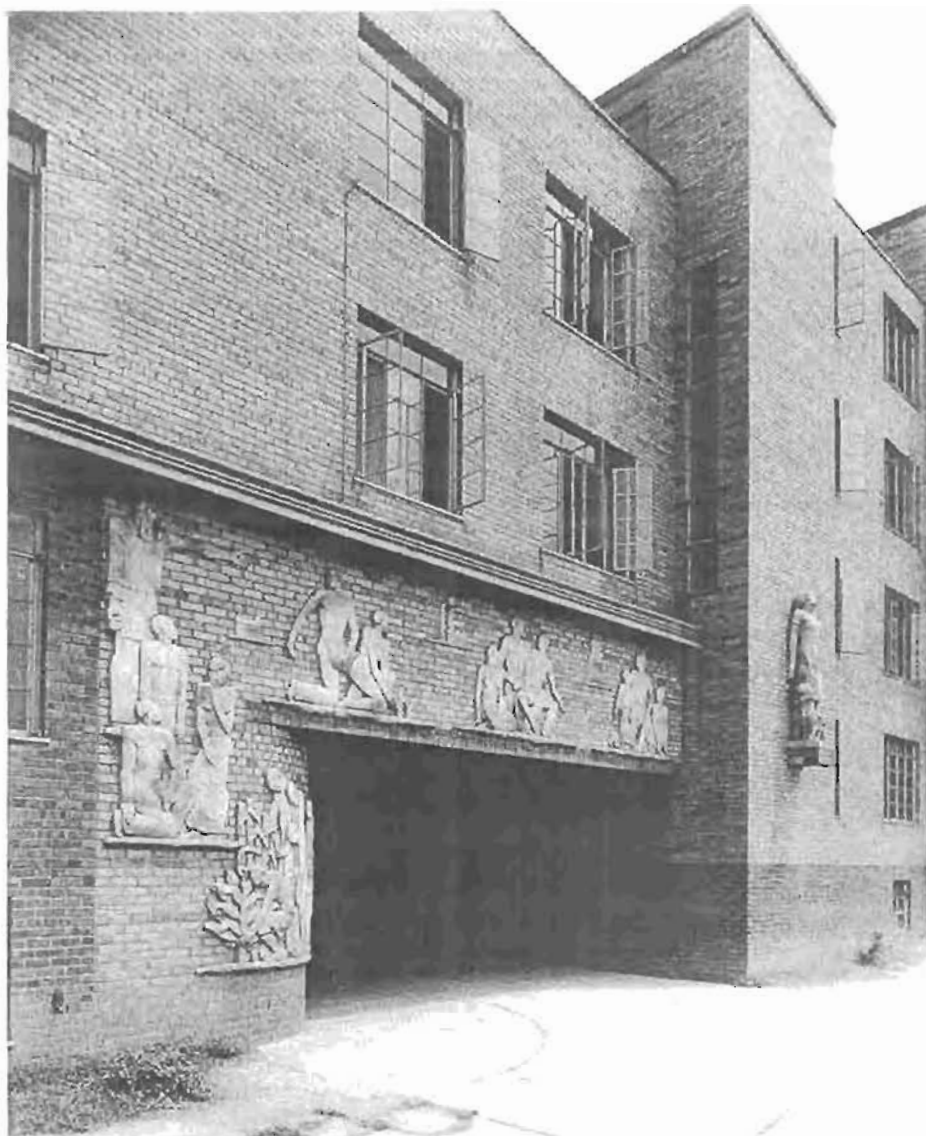
Figure 8 - Detail of building at Langston Terrace in Washington, D.C., a PWA direct-built public housing project completed in 1938, showing typical PWA-era details, including stripped, modern design, brick construction, and casement windows. This complex also featured a significant public art component, a terracotta frieze entitled "The Progress of the Negro Race." (National Register of Historic Places Nomination, 1986)
