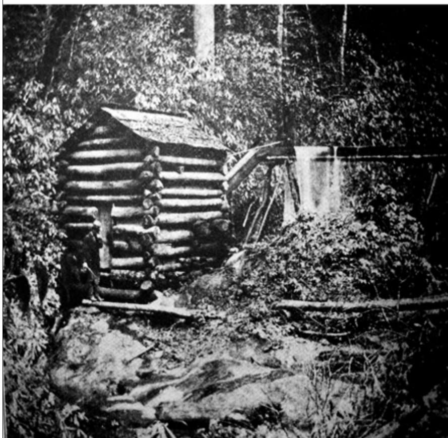
Figure 2. Grist Mills at their Simplest. Top: woman using a hand mill (quern). Bottom: a tub mill in the Appalachians (Hunter 1979).
