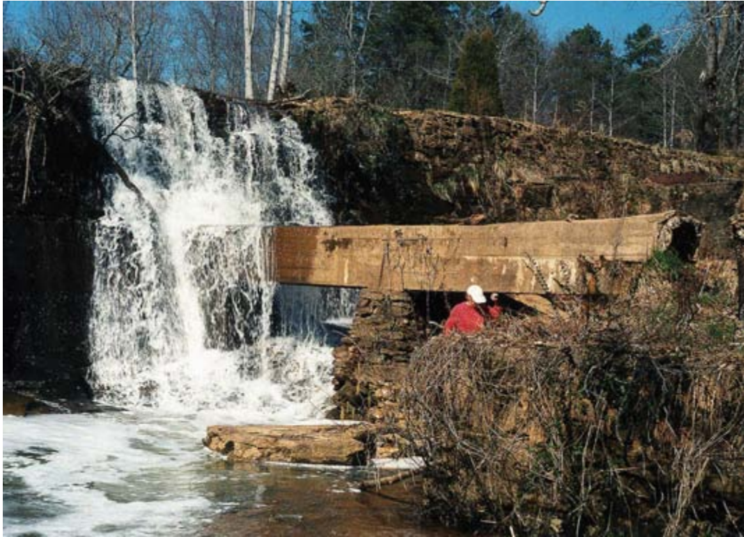
Figure 25. Photograph of Concrete Flume and Rock Pier.
