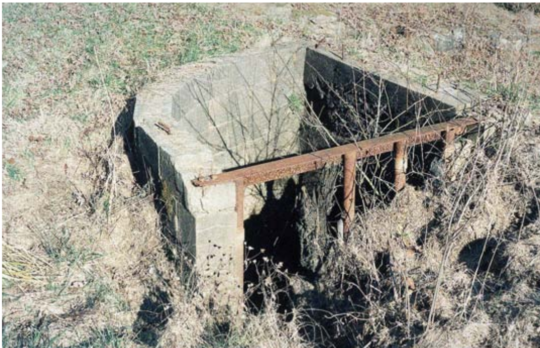
Figure 26. Photograph of Intake to Second Flume. View to the north.
