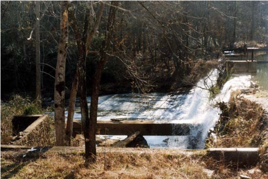
Figure 24. Photograph Showing Concrete Flume (center). View to the southwest.
