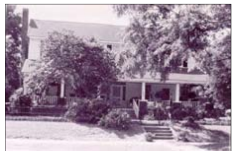
Figure 12. Dominick House (Site 304 0105)
