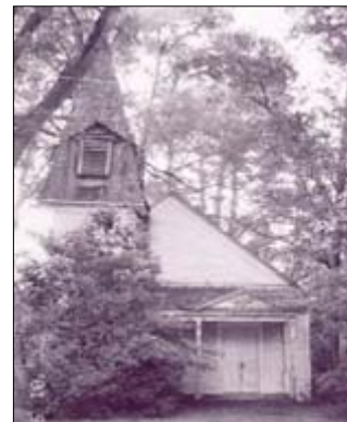
Figure 37. Old Methodist Church (Site 407 0150)
