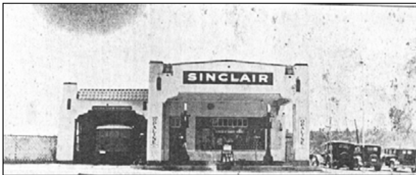
Figure 10. G. Russell Shealy Service Station ca. 1940 (Site 304 0125)
