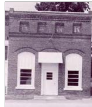
Figure 33. Bank of Pomaria (Site 407 0137)
