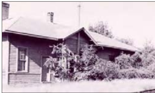
Figure 55. Prosperity Southern Railroad Depot (Site 414 0177)
