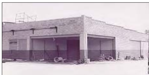
Figure 34. The Setzler Company Building (Site 407 0130)
