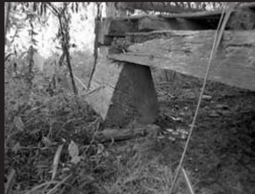
House, Detail of Wood Pier
