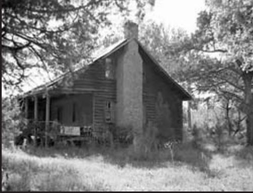
House, Oblique View
