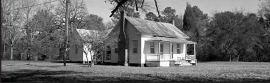
Oblique View of House
