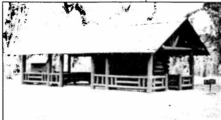
Huger Picnic Shelter
