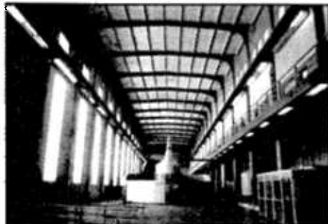
Jefferies Hydroelectric Plant, Interior
