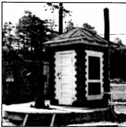
Edisto River-Goose Creek Tunnel Shaft Head Structure
