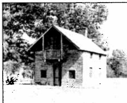
North Chachan Plantation, South Pavilion
