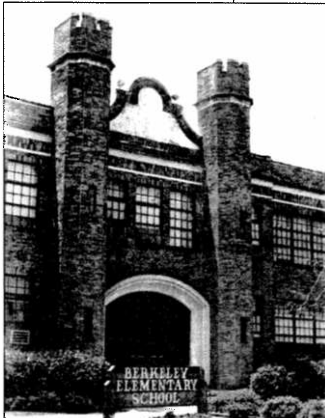
Berkeley County High School (Berkeley County Elementary), Main Street (SC Highway 6), Moncks Corner
