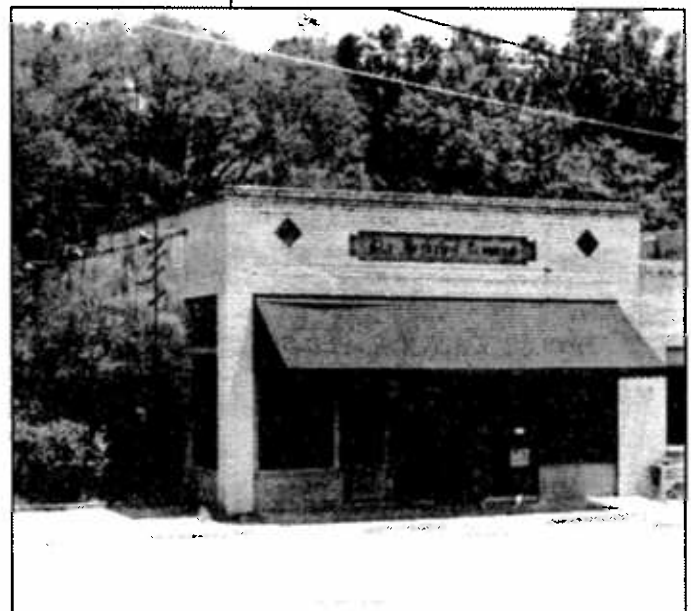
Berkeley Democrat Building , South Railroad Avenue, Moncks Corner
