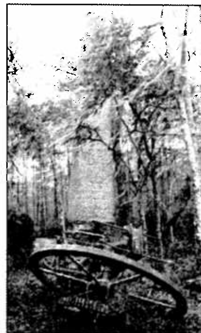
Rice Mill Chimney at Cherry Hill Plantation
