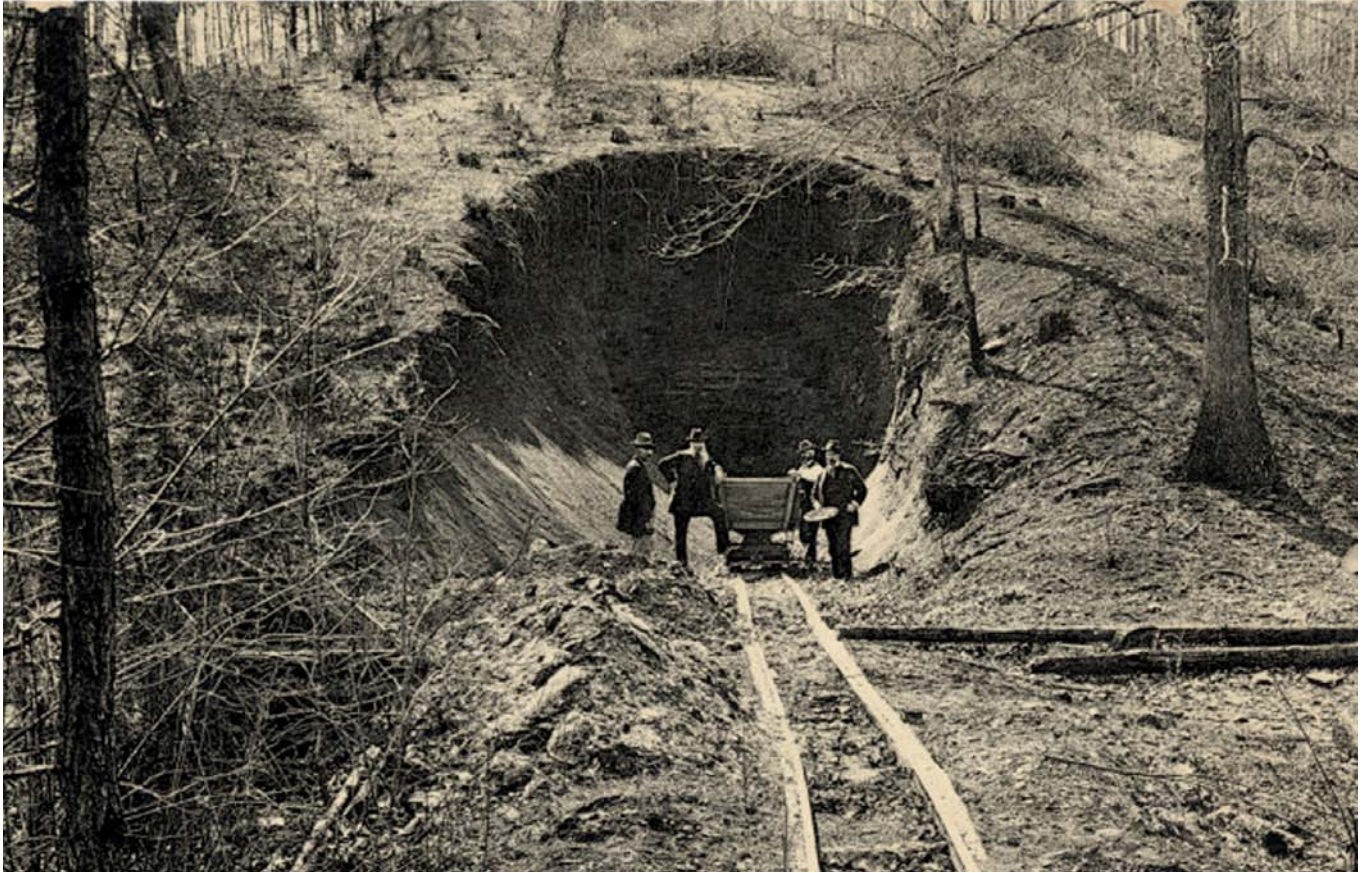
Figure 42. Adit. Note the Ore Dump Immediately Outside the Mine Opening and the Wooden Tracks. Near High Point, North Carolina. Unknown Date (Rowan County Government 2008).
