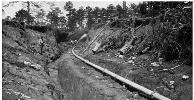
Figure 48. Water Conveyance Systems Might Leave Distinct Archaeological Traces. Parker Mine, Stanly County, North Carolina (Nitze and Wilkens 1897).
