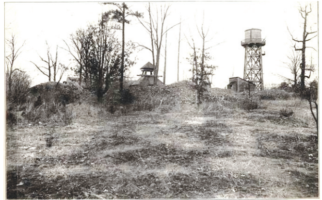
Figure 41. Mine Overburden or Ore Dumps Consist of Broken Rock Piles and are Sometimes Recognized as Unnatural Contours on Hill Sides. Howie Gold Mine, Union County, North Carolina (Howie Mining Company 1906).
