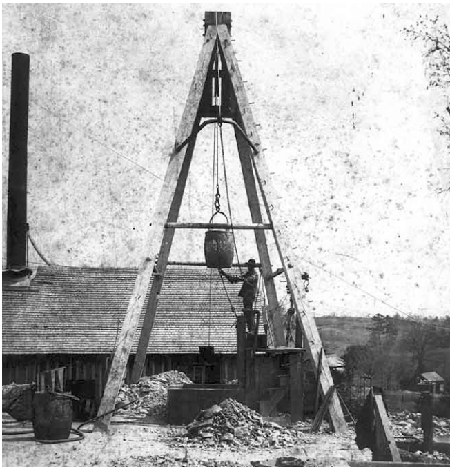
Figure 13. Headframe--Phoenix Mine, Cabarrus County, North Carolina, Late 1800s (North Carolina Office of Archives and History).
