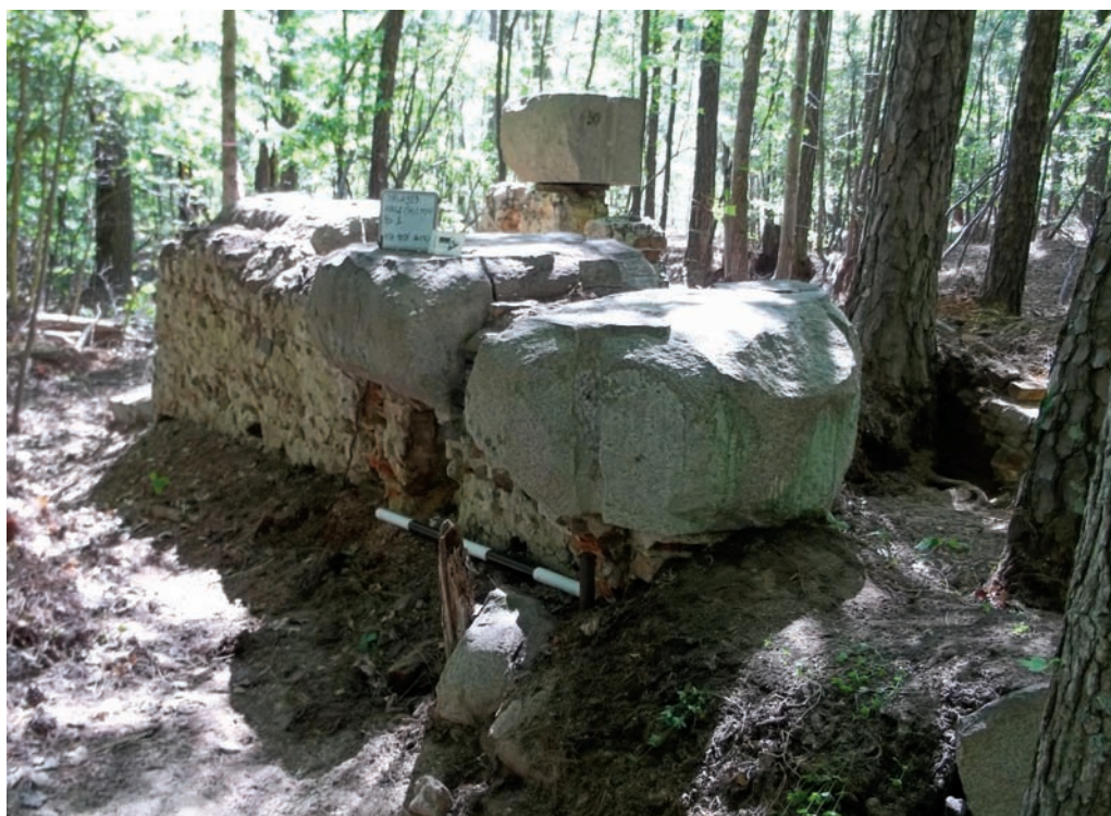
Figure 52. Masonry Equipment Mounts for the Corliss Steam Engine, Haile Gold Mine Stamp Mill (Site 38LA383), Lancaster County, South Carolina (Botwick and Swanson 2011).
