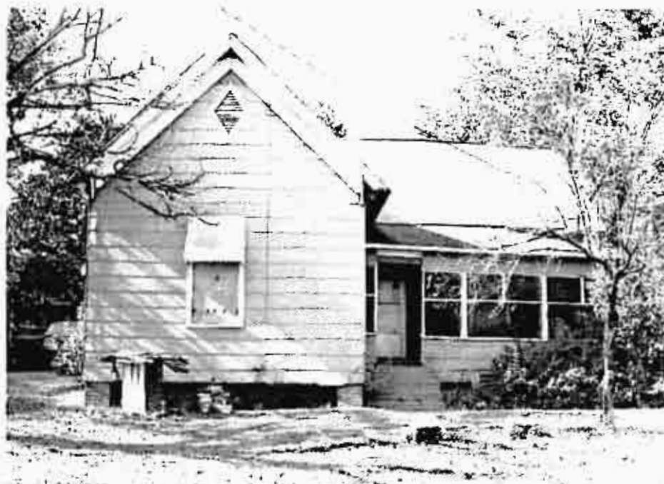
Figure 8. 224 Davis Alley, Site No. 623
