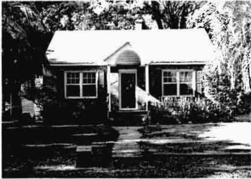
Figure 14. 1147 Palmetto Street, Site No. 460
