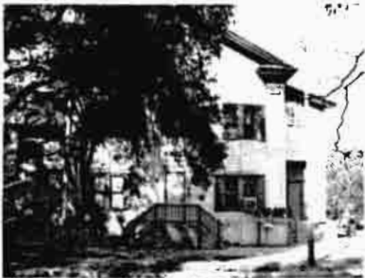
Figure 20. West End Methodist Façade
