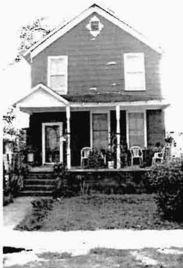
Figure 6. 1711 Front Street, Site No. 507
