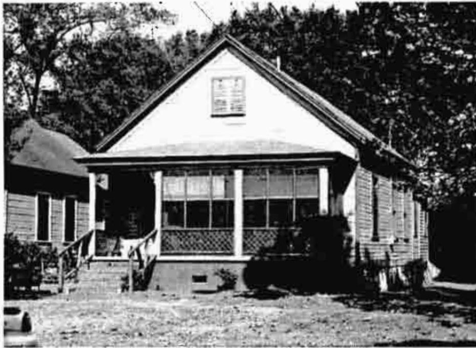
Figure 7. 1510 Front Street, Site No. 613
