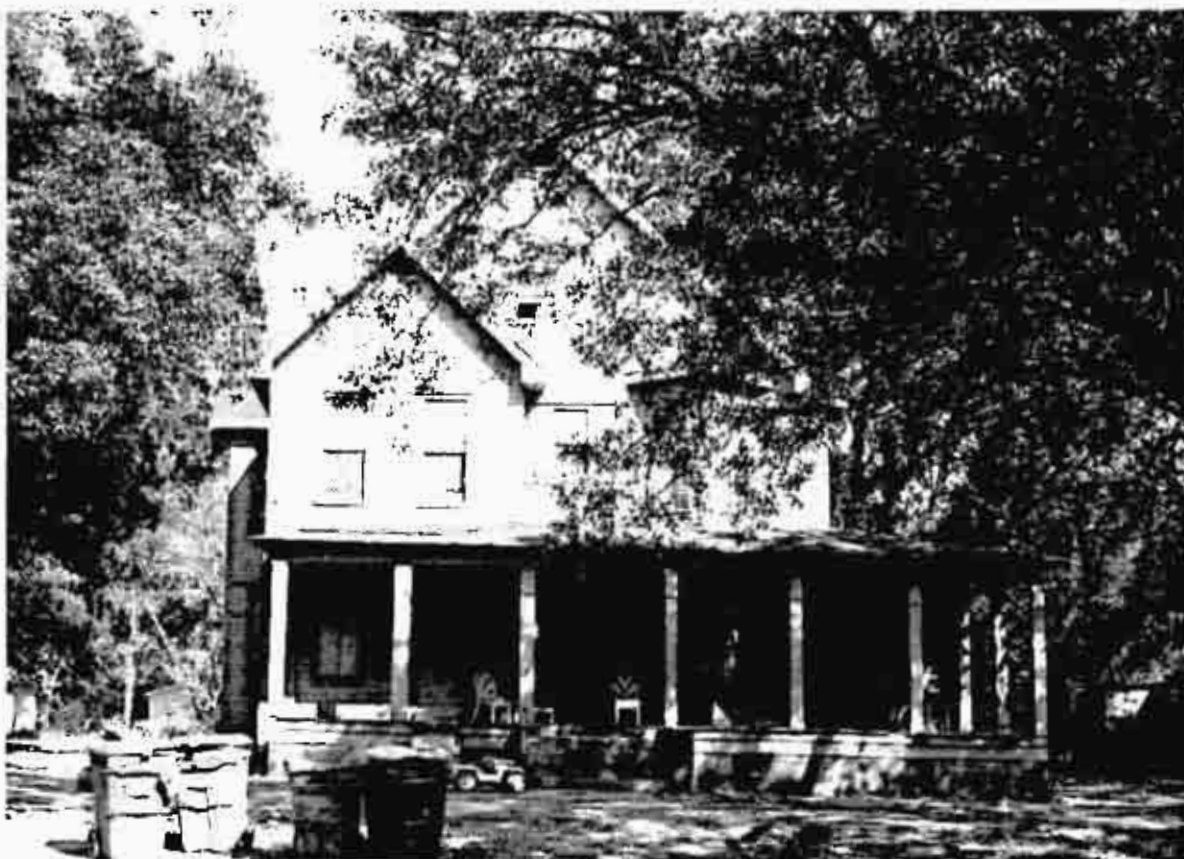
Figure 11. 1424 Winyah Street, Site No. 595
