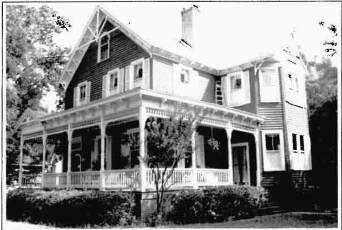
1897 Queen Anne-detailed Front-gable and Wing, 1004 Highmarket Street (Site #293)
