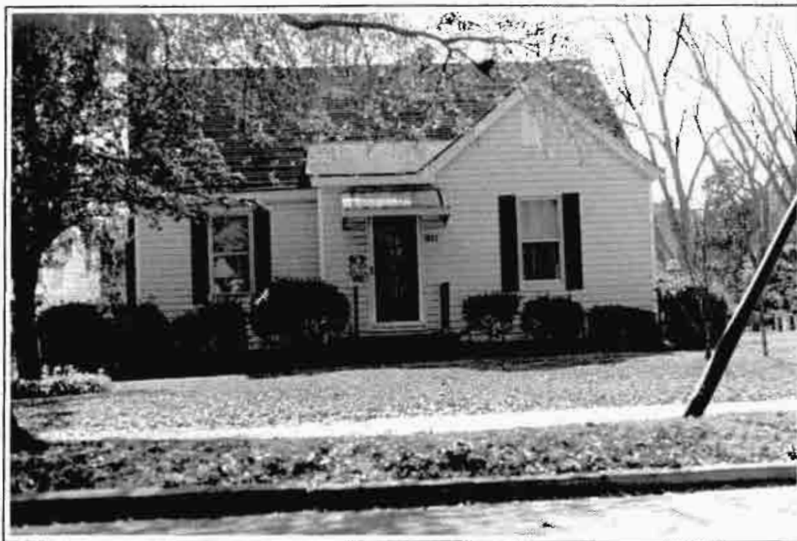
Ca. 1938 Minimal-Traditional Style, 211 Front Street (Site #398)
