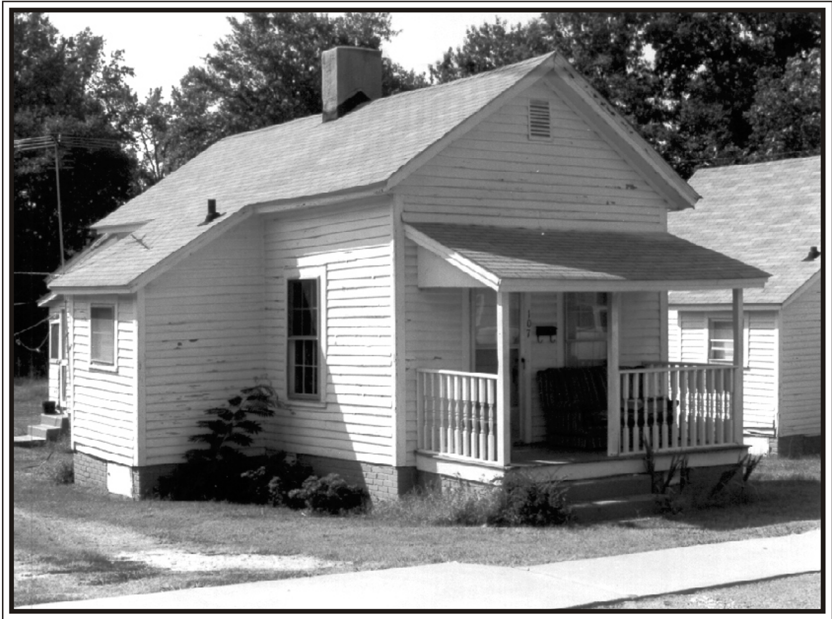
Figure 6. 107 Fourth Street, Site 177 1161, southwest oblique.
