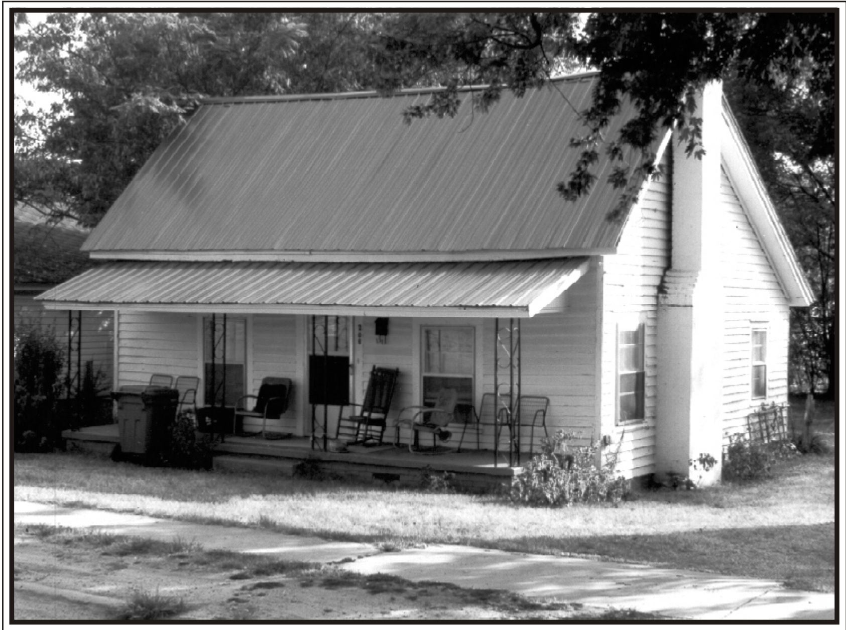
Figure 4. 206 Woodside Avenue, Site 177 1107, north oblique.
