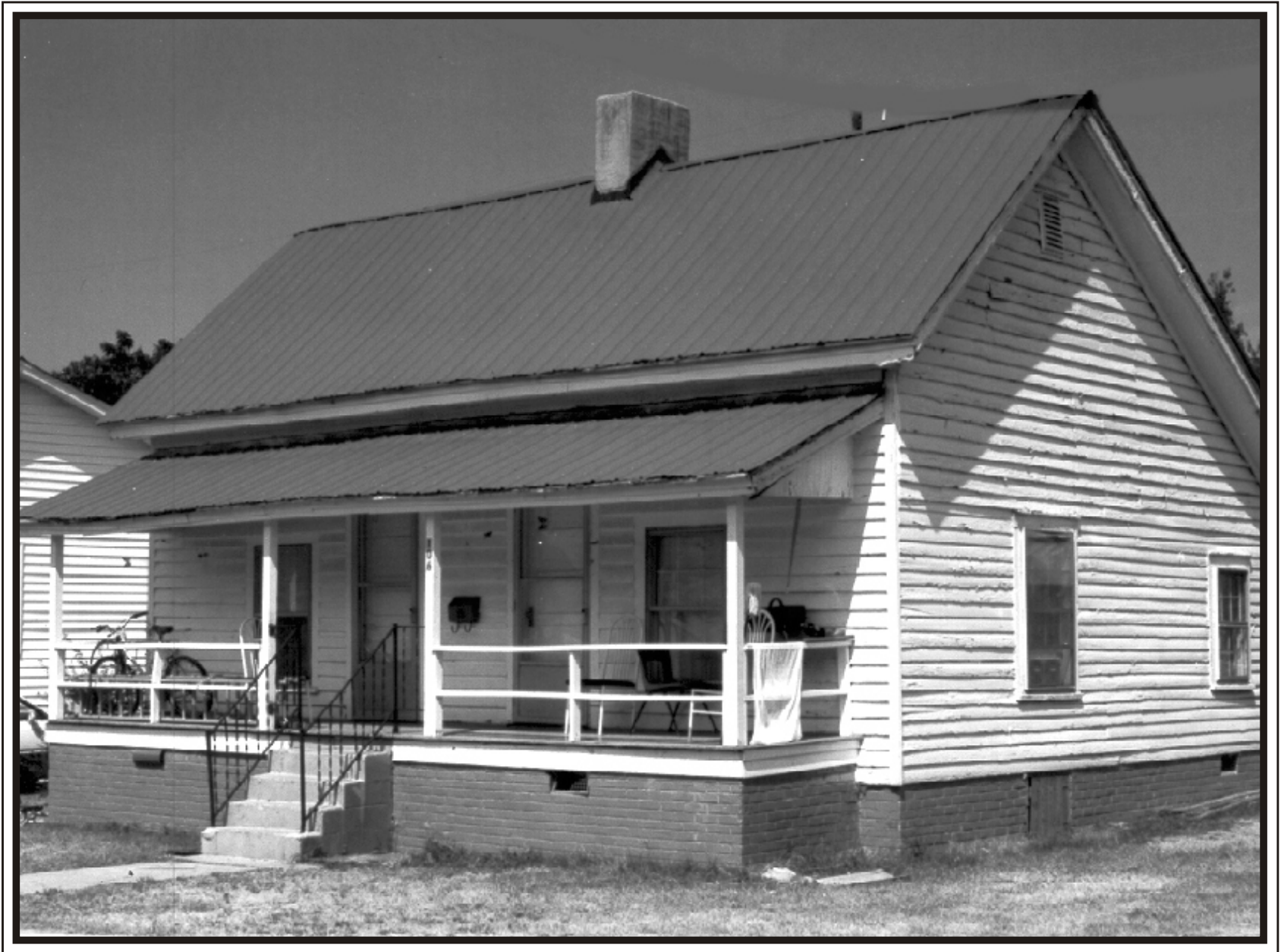
Figure 5. 106 Fourth Street, Site 177 1172, southwest oblique.
