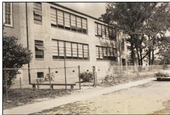
Figure 16. Chicora Elementary classroom wing. Photograph c. 1955. 69
