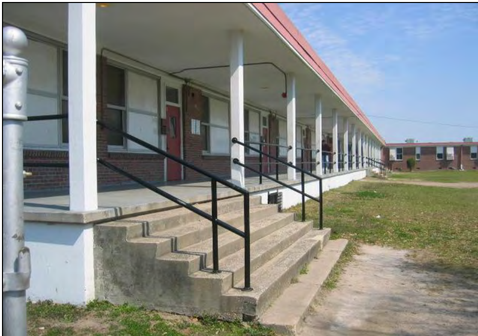
Figure 10. East Bay Elementary school, constructed c. 1955, now Sanders-Clyde Elementary school. 59
