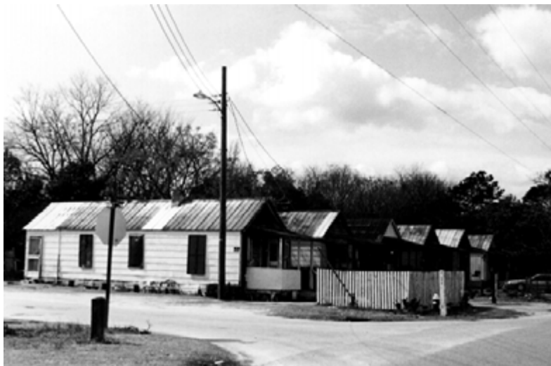
Plate 13: Shotgun Houses Built Circa 1920 Along Third Street
