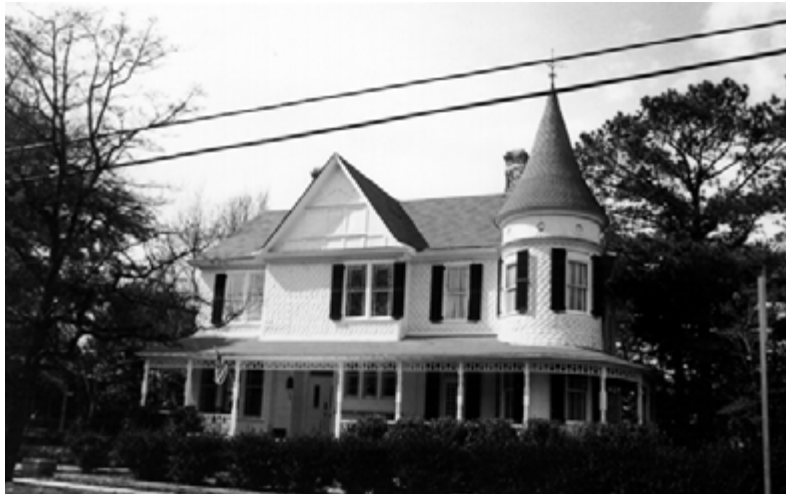
Plate 6: “Drummer’s Home” (site # 0259) at 209 Cashua Street
