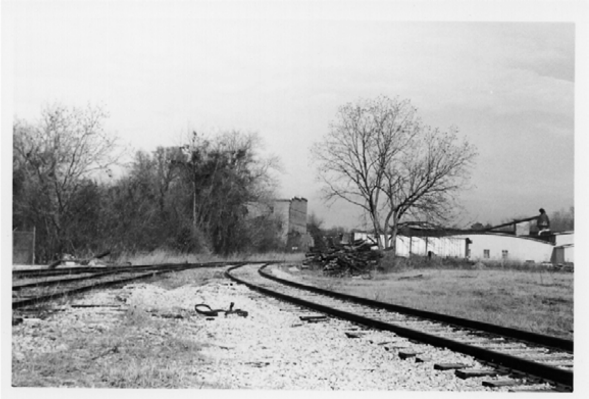
Plate 1: Railroad Tracks East of Main Street
