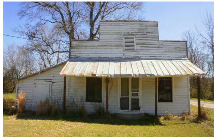
Unnamed Store with Parapet, Sumter County
