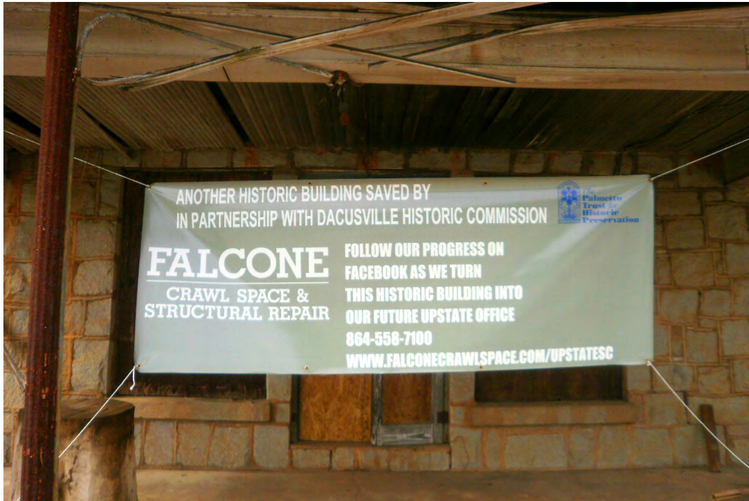
Preservation of the Hester Store is ongoing through a partnership between a private firm, the Dacusville Historic Commission and The Palmetto Trust for Historic Preservation.
