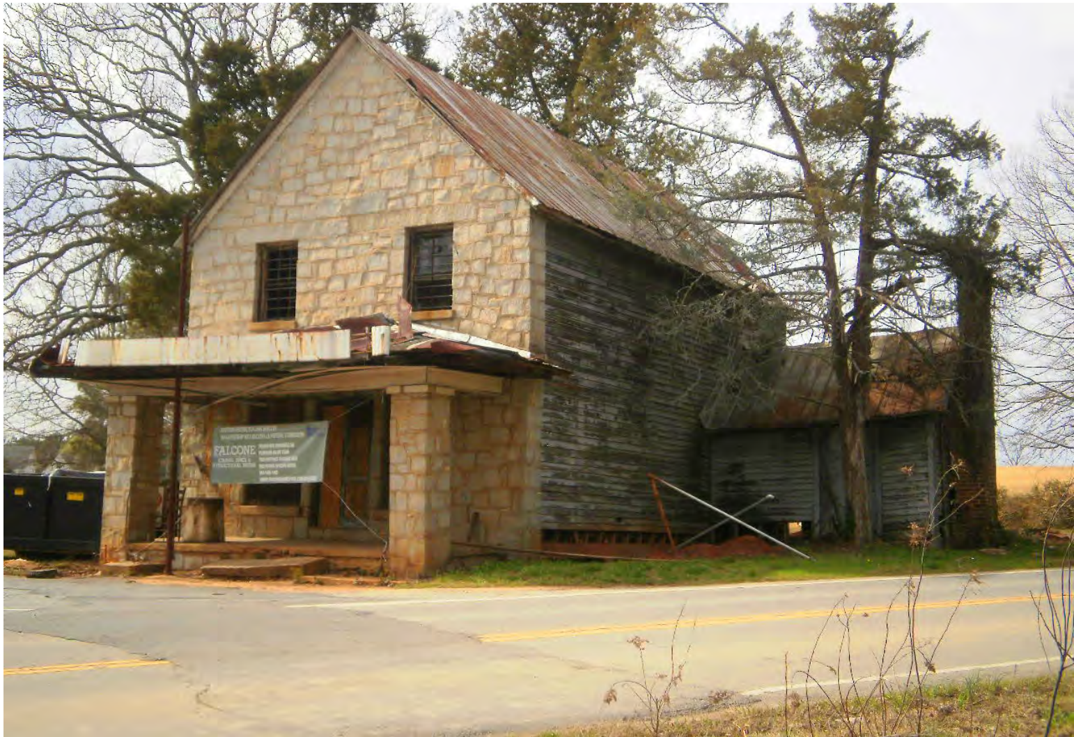
Hester's Store, Dacusville, was constructed in 1893. Originally clad in weatherboard, it was refaced with granite in the 1930s to update the appearance of the store. This alteration is historic and reflects the intent of the storeowner to further his commercial business. Such alterations do not compromise the eligibility of a store instead they convey cultural information about evolving commercial and consumer practices.
