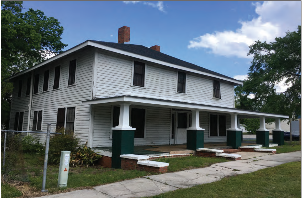
Figure 5.8 A view of the Frederickson House (0316), west oblique.
