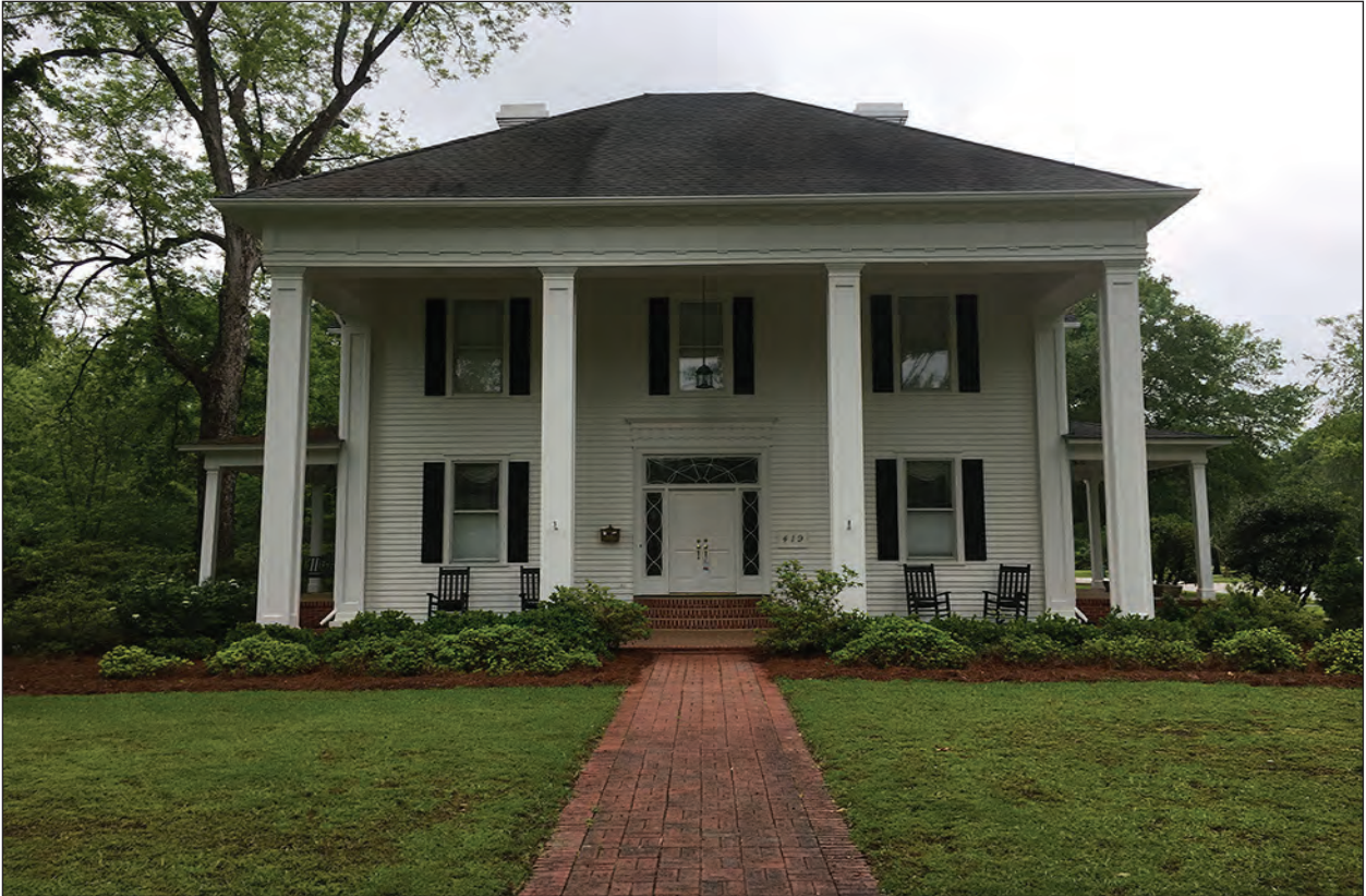
Figure 4.6 View of the First United Methodist Church Manse (0162), example of a Neoclassical style house.
