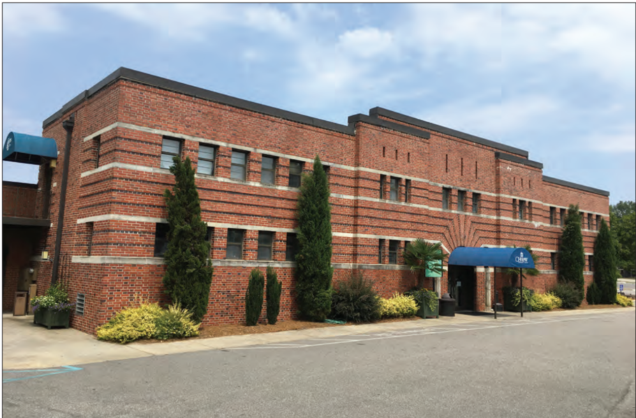
Figure 5.2 View of the Cheraw Amory building (0371), east elevation.
