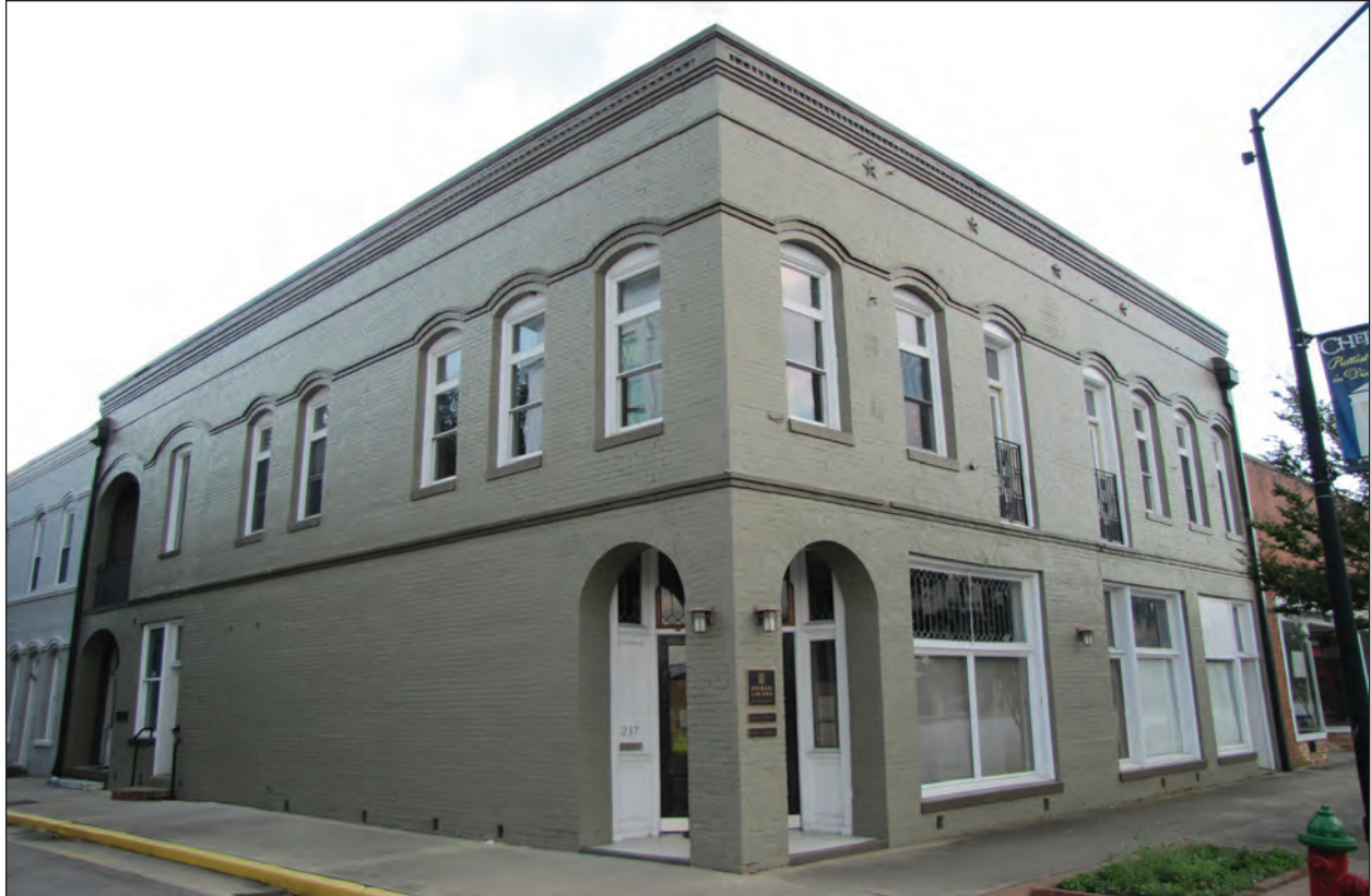
Figure 4.22 View of the Hotel Covington (0275), example of a two-part block commercial building.
