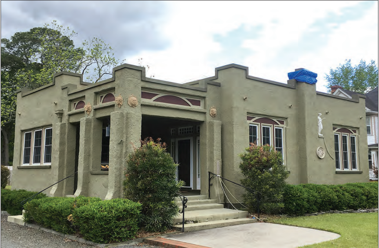
Figure 4.10 View of Crawford-Overton house (0195), example of an Art Deco house.
