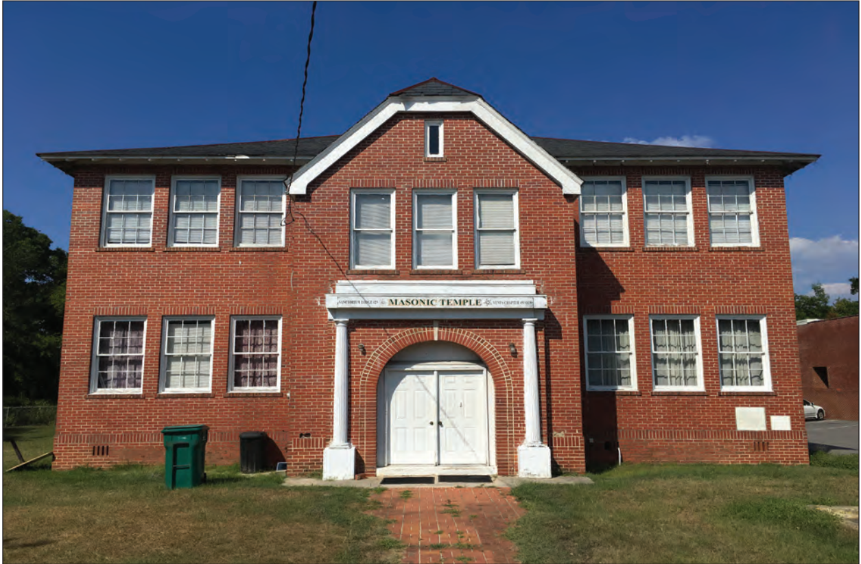
Figure 5.5 A view of the Coulter Memorial Academy Administration Building (0372), southwest elevation.
