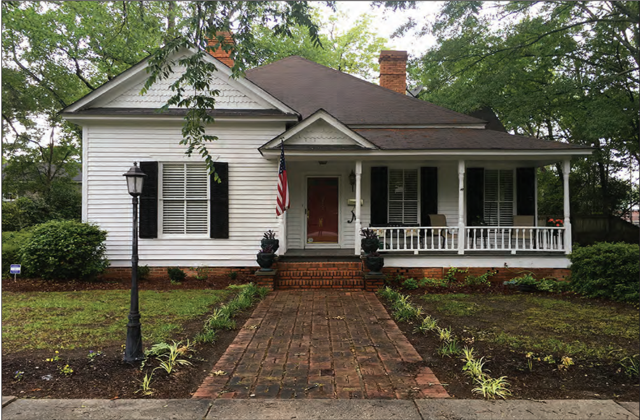
Figure 4.3 View of the Hilliard-Bundy House (0129), example of a Folk Victorian style house.
