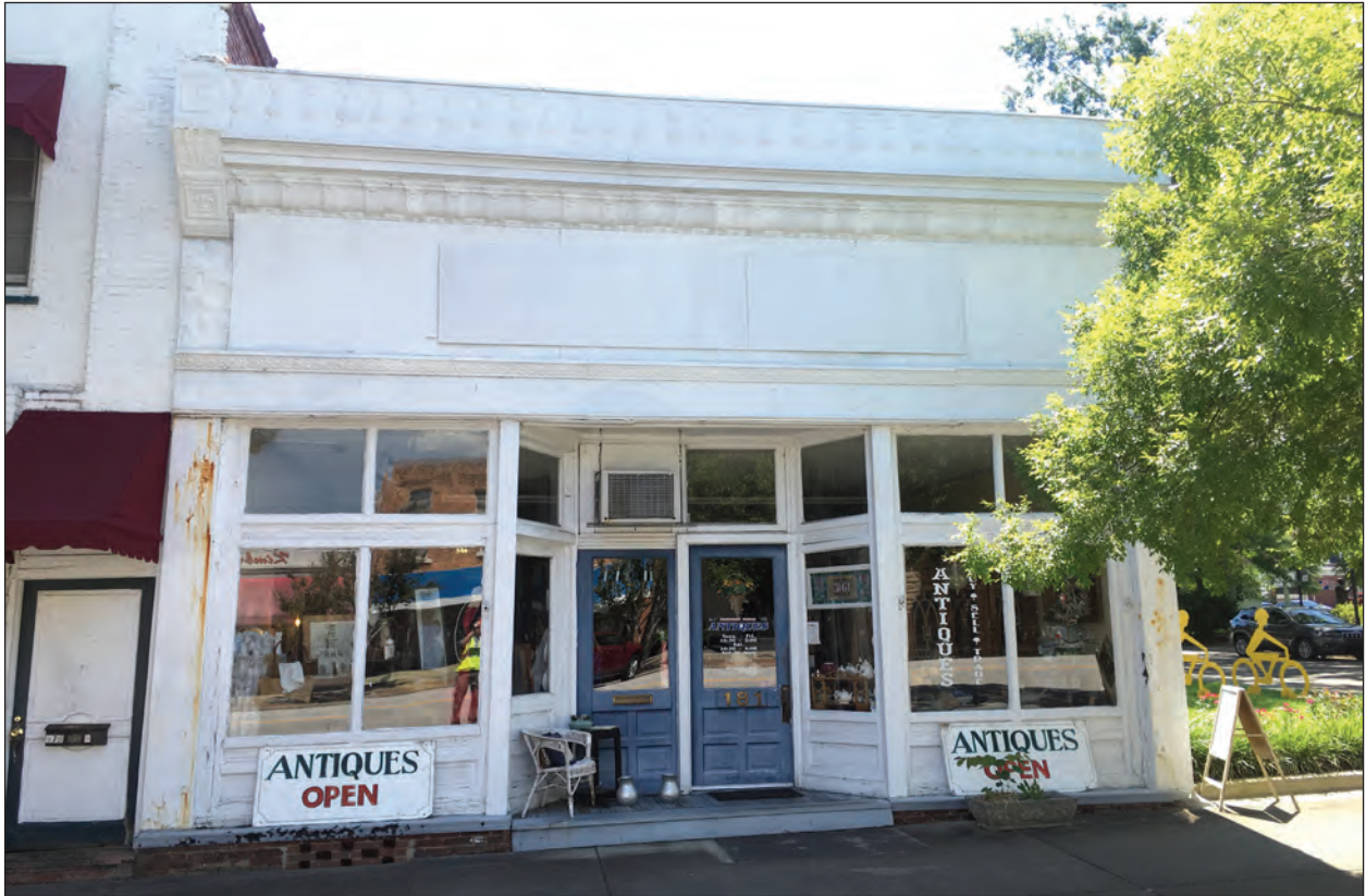
Figure 4.23 View of the Michael and Associates Building (0292), example of a one-part block commercial building.
