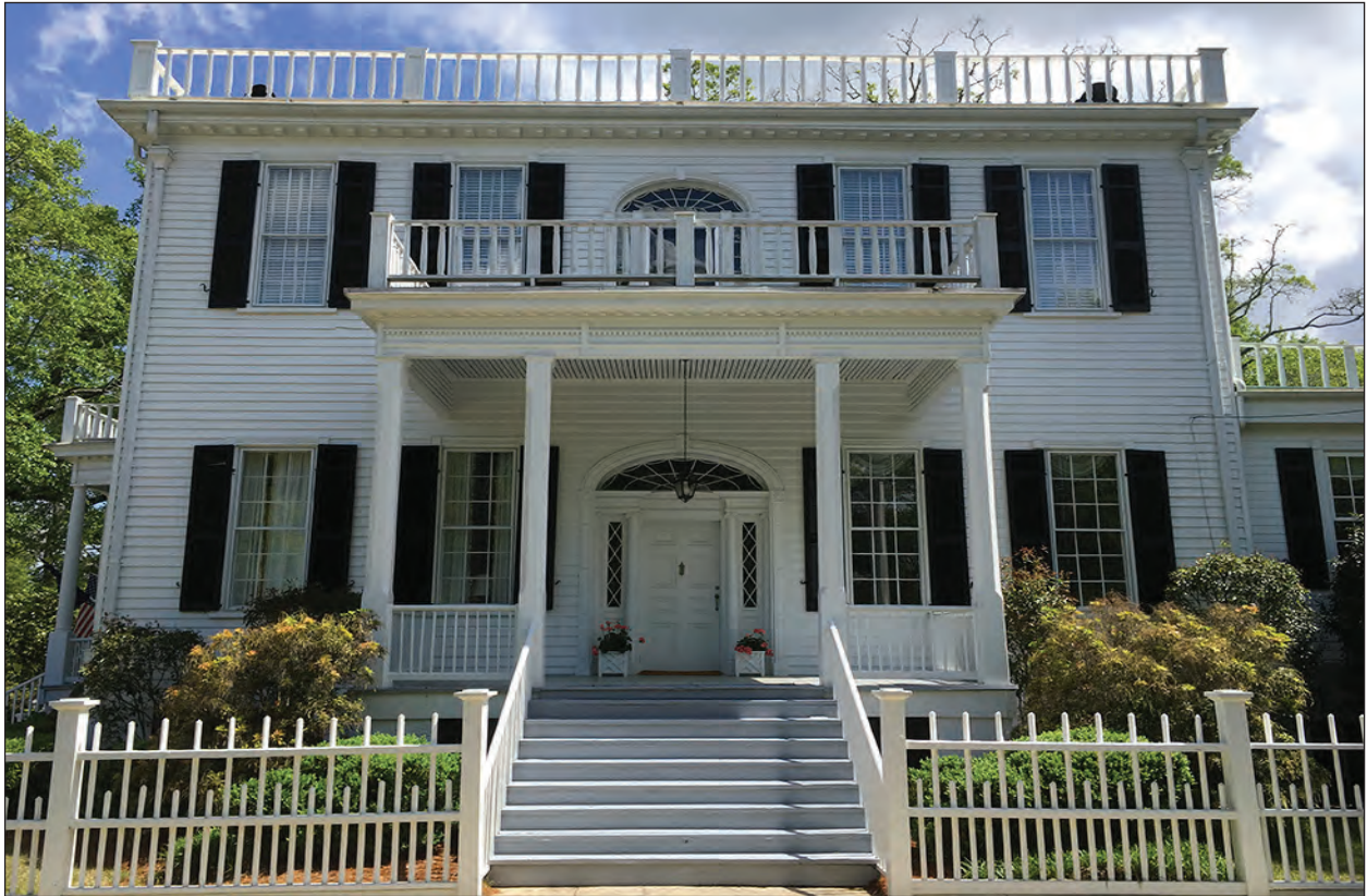
Figure 4.1 View of the Lafayette House (0232), example of the Federal style.
