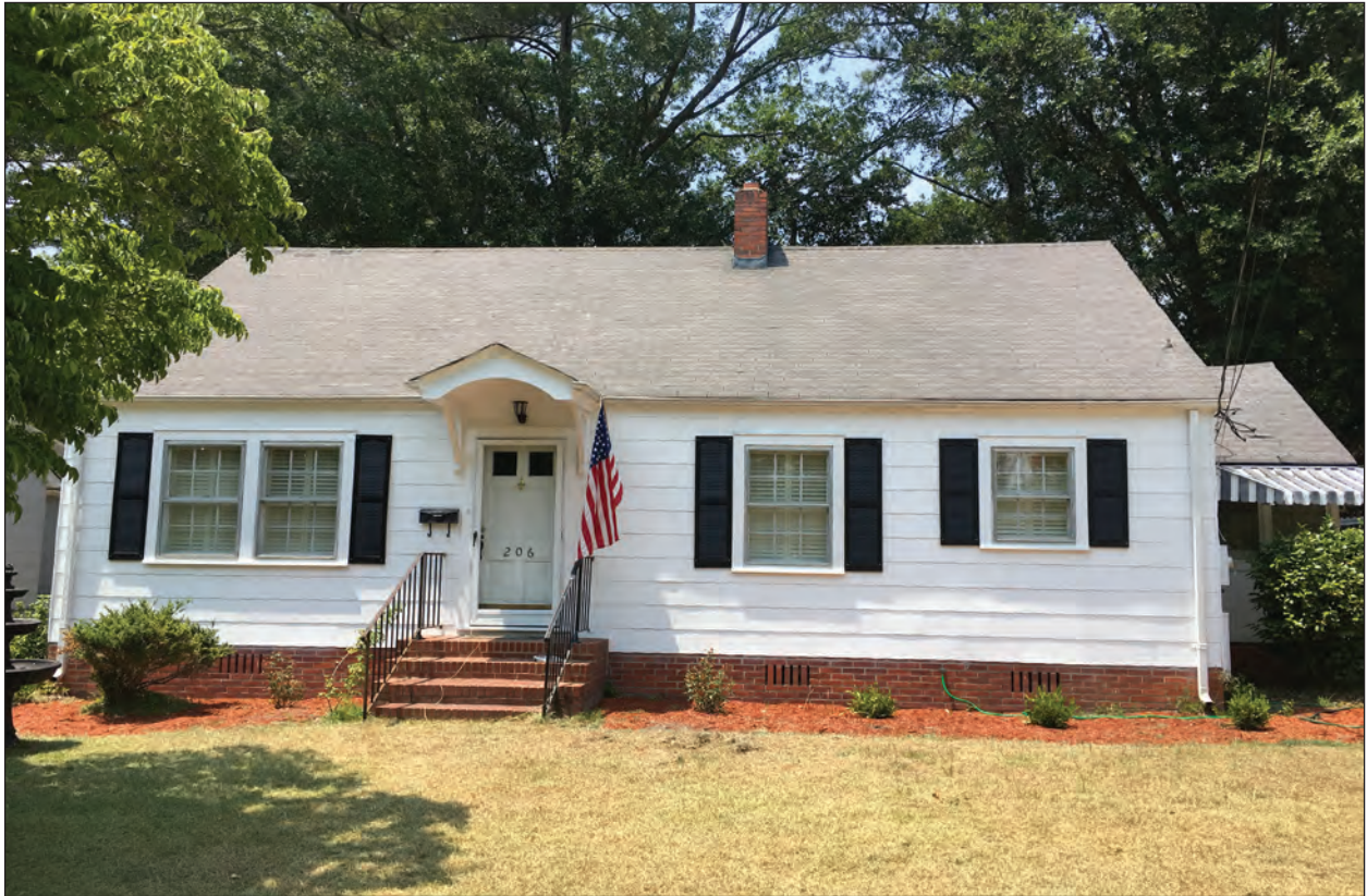
Figure 4.11 View of Resource 0682, example of a Minimal Traditional style house.
