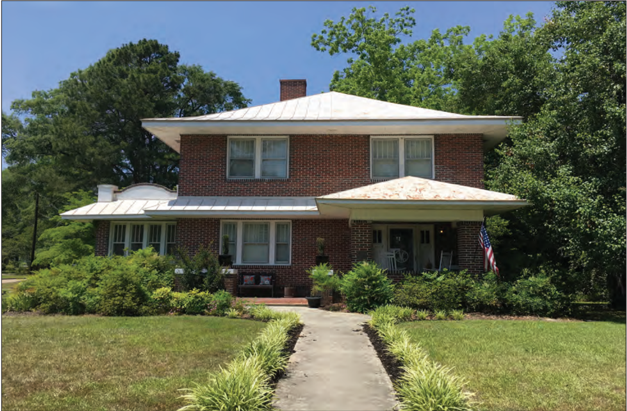
Figure 4.8 View of the Latta-McManus House (0094), example of a Prairie style house.
