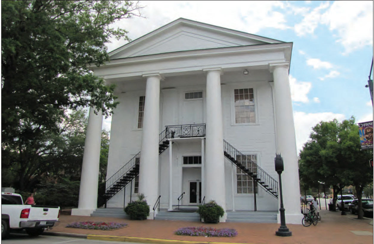
Figure 4.29 View of the Cheraw Town Hall (Resource 0284), example of a Greek Revival government building.
