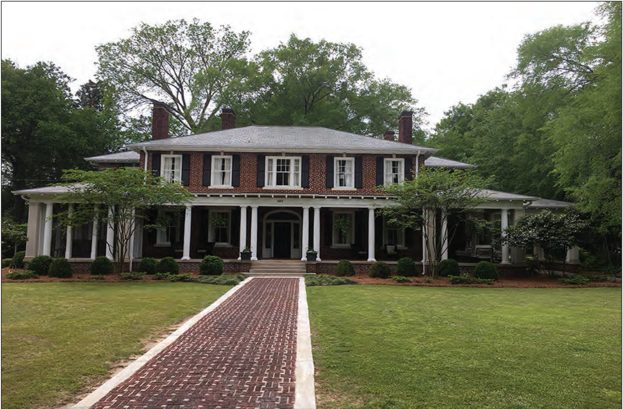
Figure 4.5 View of the Moore-Ingram House (0222), example of the Colonial Revival style.
