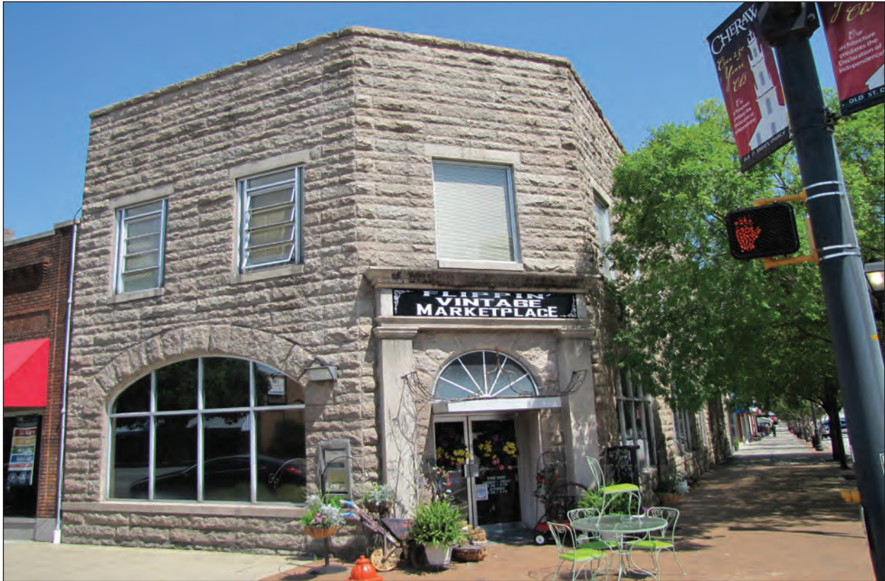
Figure 4.25 View of the South Carolina National Bank Building (0334), example of a vault commercial building.
