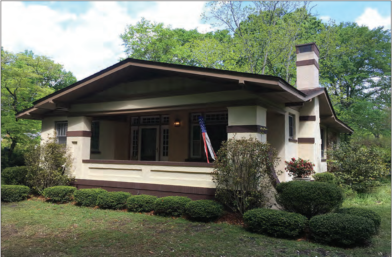
Figure 4.9 View of the Bunch-Moore house (0214), example of a Craftsman style house.
