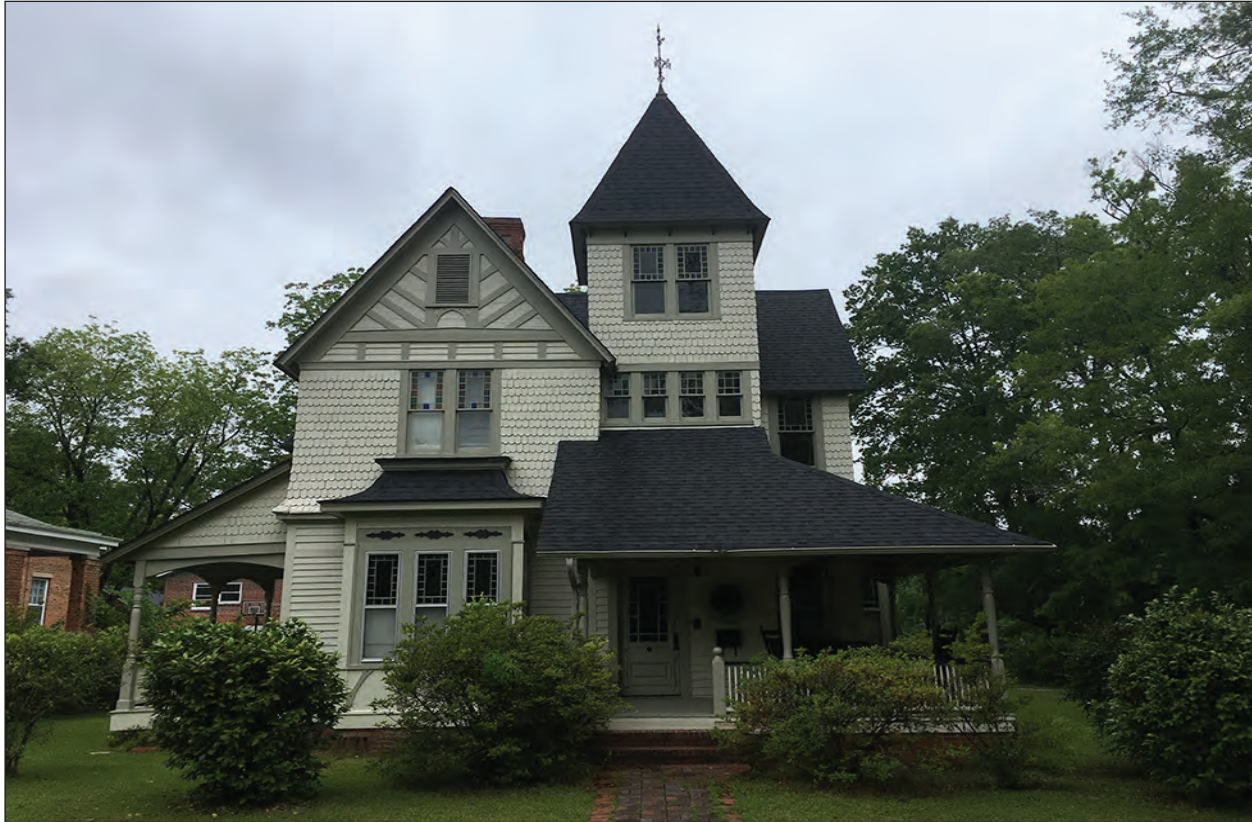
Figure 4.4 View of the Wannamaker House (0122), example of the Queen Anne style.
