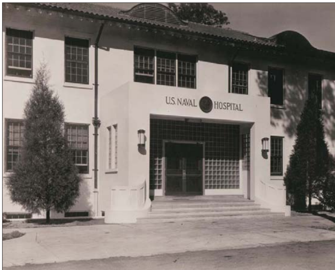
B. Main Entry of Hospital, Building NH45
