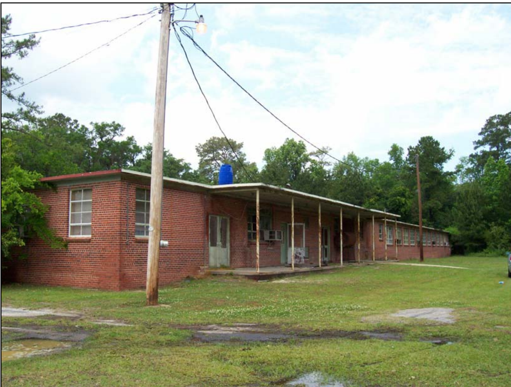
Figure 6. Rear of Bucksport Elementary School.
