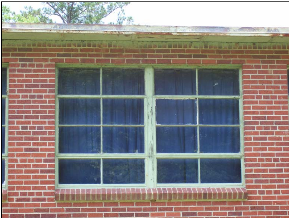
Figure 17. Window detail at Bucksport Elementary School.
