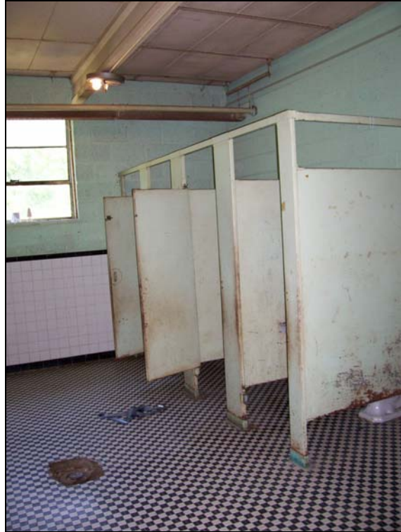
Figure 12. Girl's bathroom at Bucksport Elementary School.
