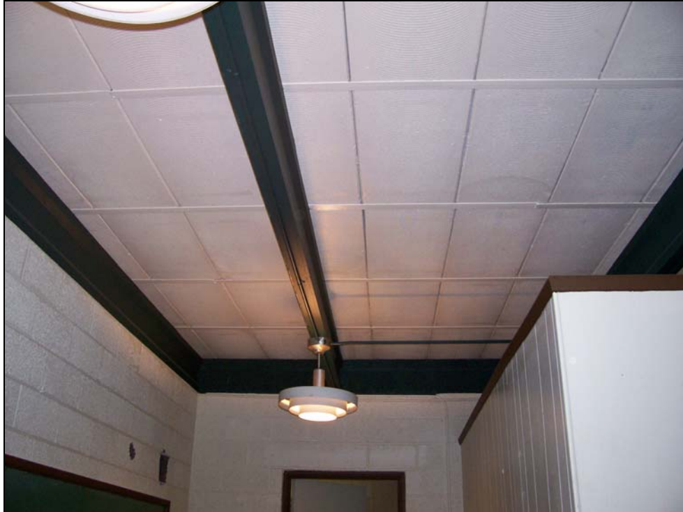
Figure 18. Incandescent light fixture at Bucksport Elementary School.
