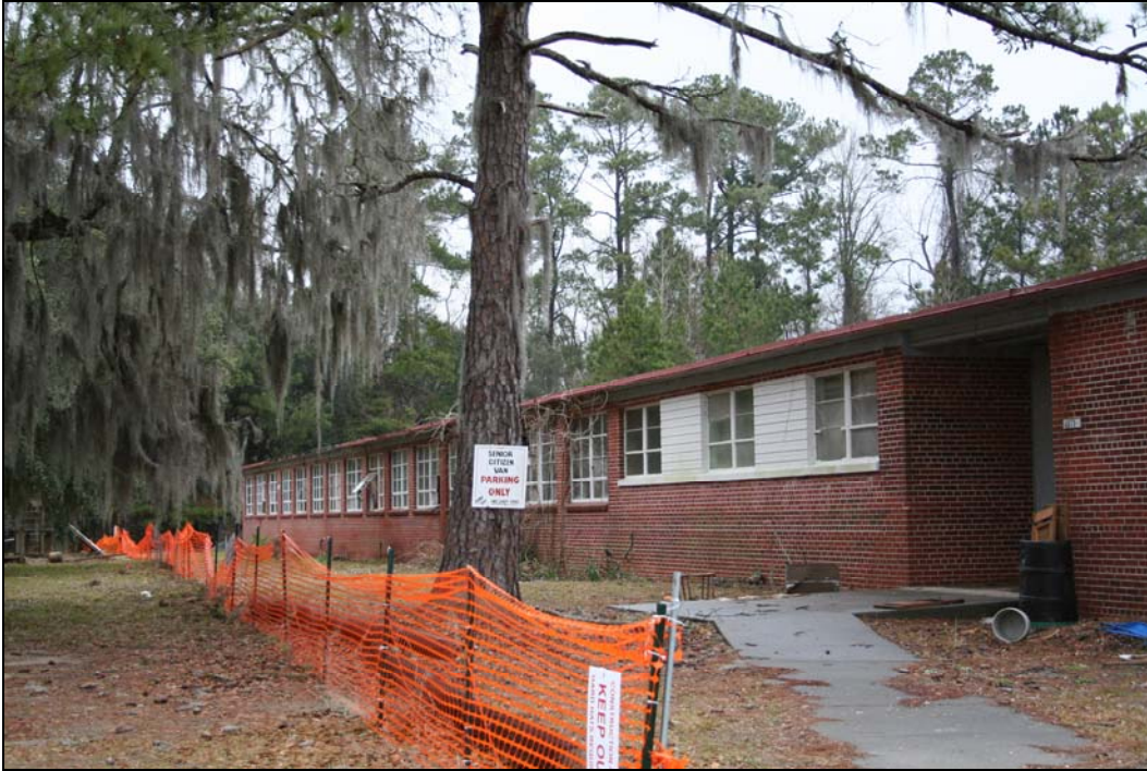
Figure 5. Front of Bucksport Elementary School.
