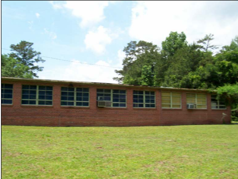
Figure 16. Bank of classroom windows at Bucksport Elementary School.
