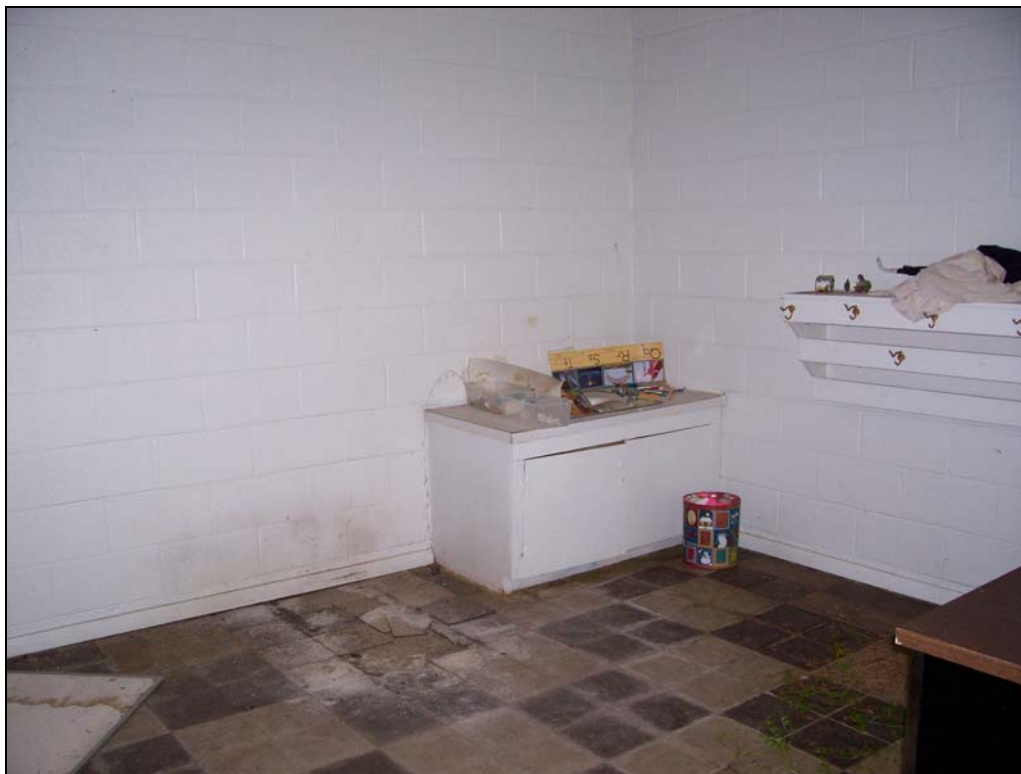
Figure 8. Classroom at Bucksport Elementary School, with sink and coat hooks.
