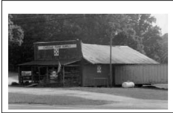
Figure 4. Cheddar Farm Supply, Site 1108.
