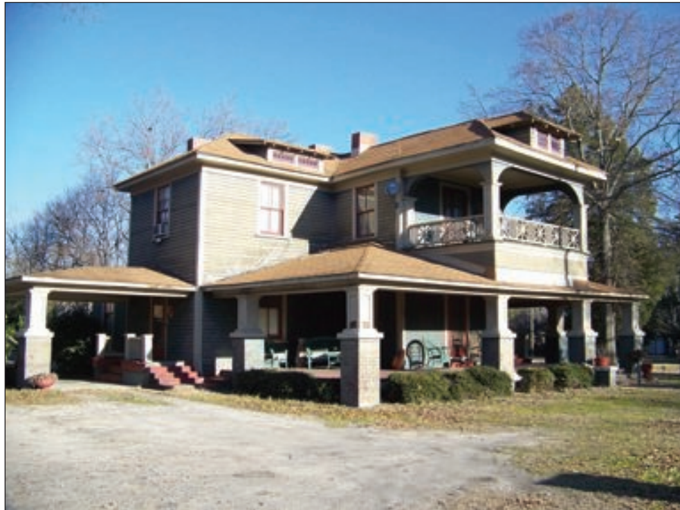
Figure 5.9 Resource 2039, looking southeast (top); and Resource 2087.00, looking southwest (bottom).
