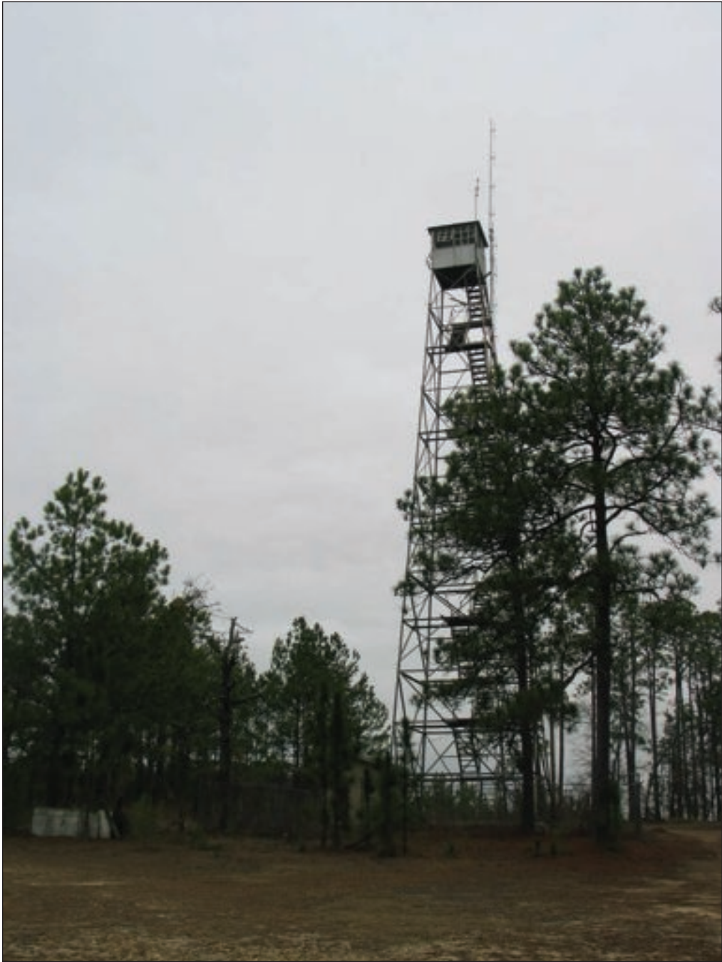
Figure 5.10 View of Resource 2364, looking south.
