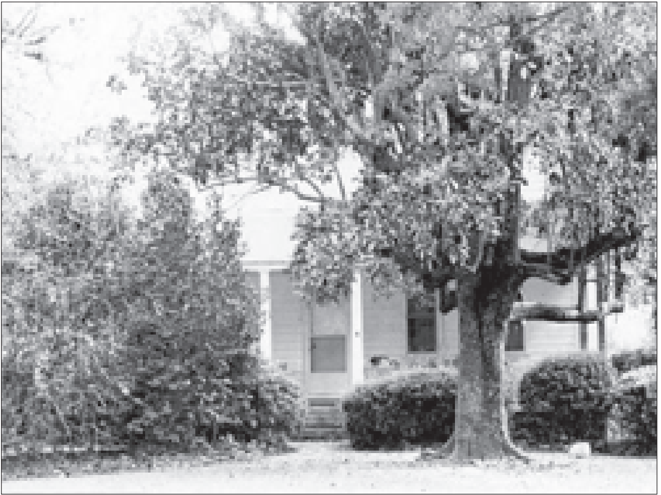
Figure 3.6 View of the Robertson-Easterling-McLaurin House (courtesy of SCDAH).
