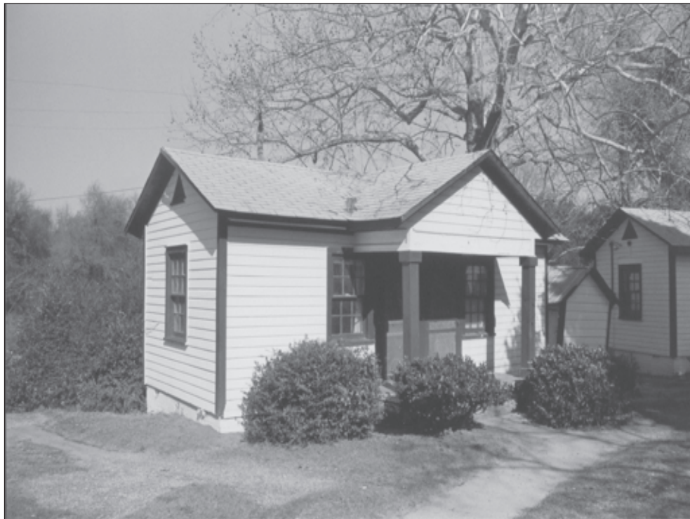
Figure 5.6 Resource 1019.06, looking southeast (top); and Resource 1019.08, looking south (bottom).
