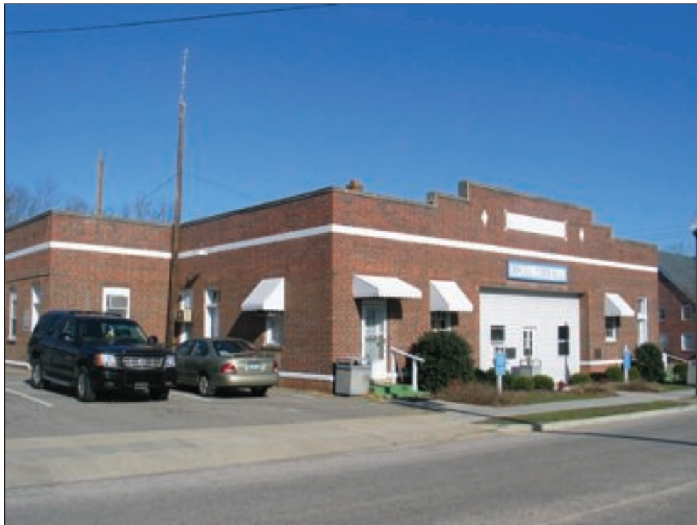
Figure 4.11 Resource 1665, the Fletcher Memorial School, an example of the Neoclassical style (top); and Resource 1973, McColl Town Hall (bottom).
