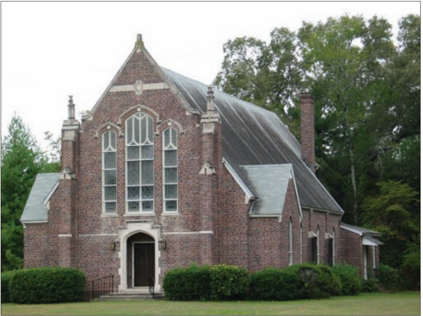
Figure 4.10 Resource 1667, Pine Grove United Methodist Church, an example of the Gothic Revival style.
