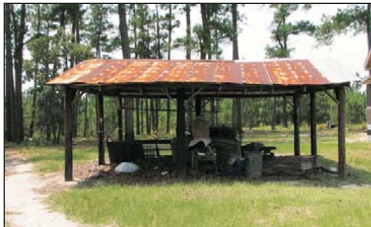
20B. Open Shed (Site U/67/0587.01)
