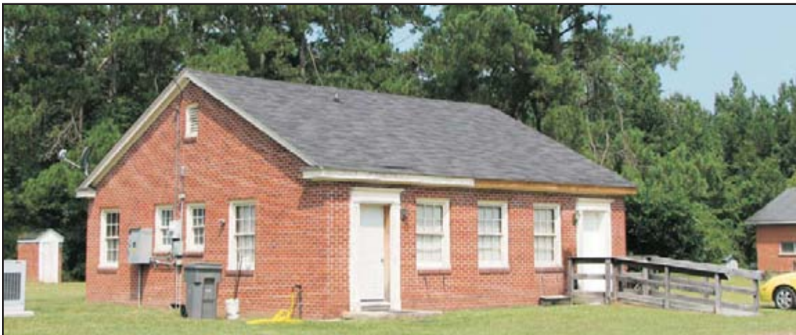
26B. Minimal Traditional (Site U/67/0692) - Marion County EMS, Britton's Neck Substation
