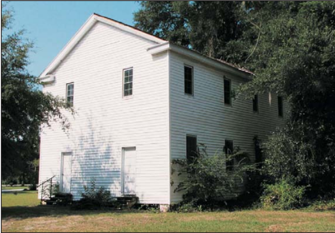
26A. Front Gable (Site U/67/1018) - Little Pee Dee Masonic Lodge
