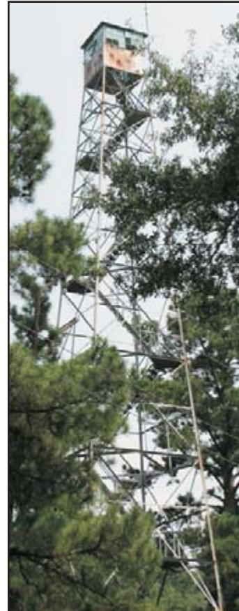
29B. Lookout Tower (Site U/67/0597)
