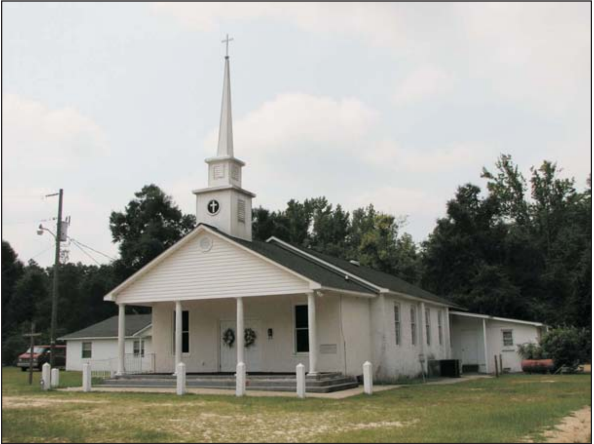
22A. Front Gable with Steeple (Site U/67/0671)
