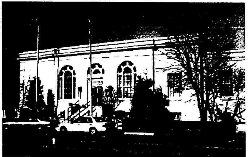
Figure 86: Renaissance style, U.S. Post Office, 542 DeKalb Street, (sited 0080).
