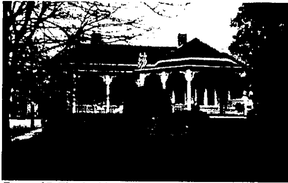
Figure 37. This building, located at 1209 Lyttleton Street, was constructed about 1886 by Jake Herschberger, a merchant who came to Camden from Germany. Herschberger later changed his name to Hirsch and with his brother, Gus, founded the Hirsch Brothers Department Store on Broad Street.
