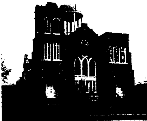
Figure 90. Late Gothic Revival style, Trinity Methodist Church, 704 DeKalb Street (site 0784).
