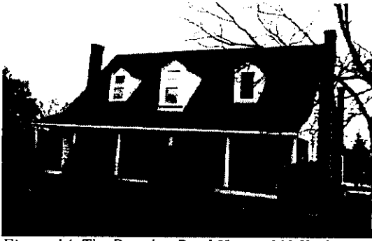
Figure 14. The Douglas-Reed House, 312 York Street (site 0445) is typical of the surviving small early nineteenth century buildings. It was built in 1812 as a three-room, one-story dwelling and was enlarged by subsequent owners.
