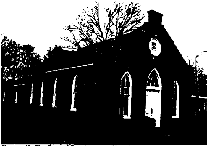
Figure 48. The Second Presbyterian Church congregation was established in the late nineteenth century by a group of ex-slaves. The cornerstone of the church, which is located at 816 Market Street (site 0460) indicates that work was begun on the building in 1897. It was not until 1904, however, that the church was finally dedicated.
