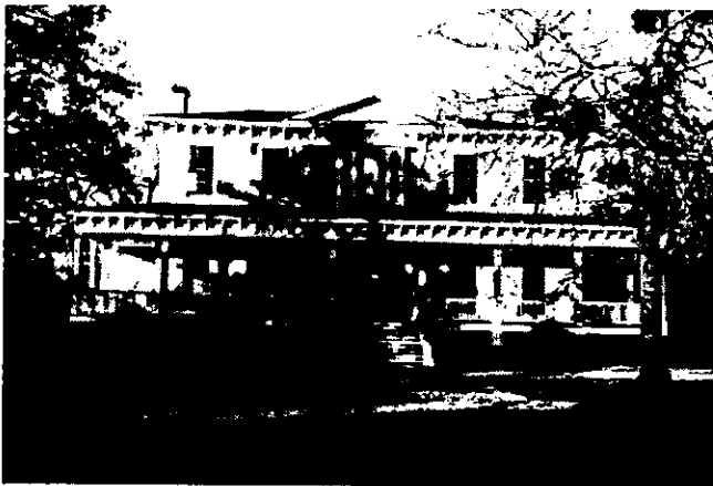
Figure 92. Italianate style, Hobkirk Inn, 1919 Lytleton Street (site 0355).
