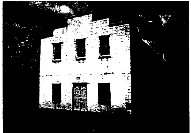
Figure 61. Haddoth Lodge No. 250, F&AM, 714 York Street (site 0784).
