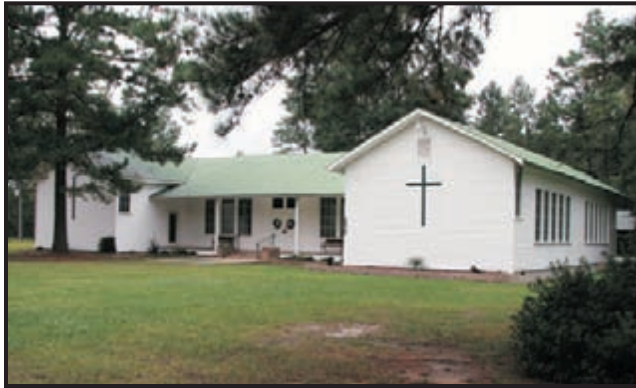
32A. Modern Vinyl and New Windows Replacing Original Materials on Historic Buildings, Such as This Rosenwald School (Site 2012)
