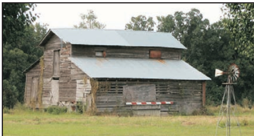
14E. Transverse Barn with Enclosed Attached Sheds (Site 3429.01)
