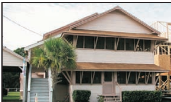
13F. Typical Two Story, Front Gable Beach Cottage With Partially Enclosed Porches (Site 2299)
