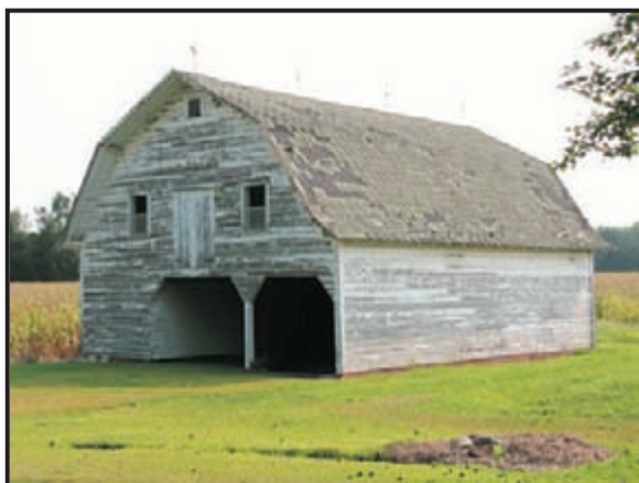
14C. Typical Large Barn and Garage with Gambrel Roof (Site 1625.04)
