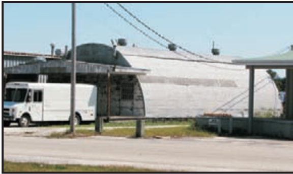
22C. Quonset Hut Metal Building (Site 2818)
