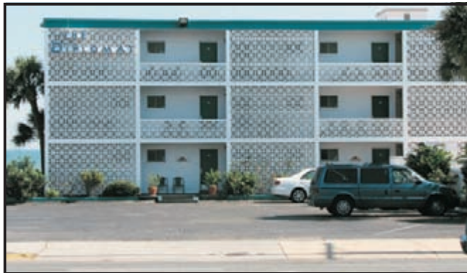
32C. Loss Mid-Century Buildings and Designs, Such as the Use of Decorative Concrete Block as Screening and Building Material (Site 2914)
