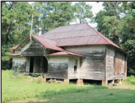
23C. Rural School with Square Shape and Hip Roof (Site 1629)
