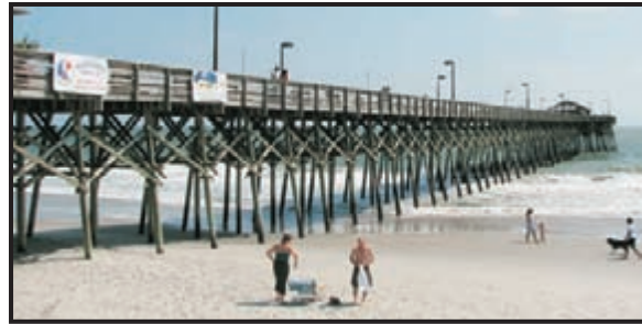
22B. Typical Wood Pier (Site 3493)
