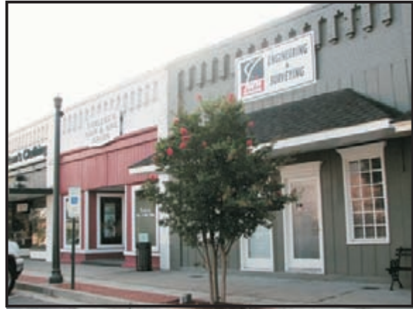
16B. Typical Multi-Bayed, One Part Commercial Block With Decorative Cornice, Altered (Site 1662)
