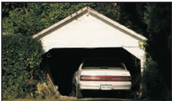
22G. Typical Single Bay Garage (Site 3154.01)
