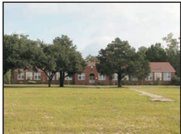
17D. Good Example of Rural Brick School (Site 2153)
