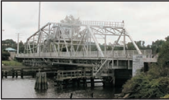
22A. Typical Steel Truss Bridge (Site 0326)
