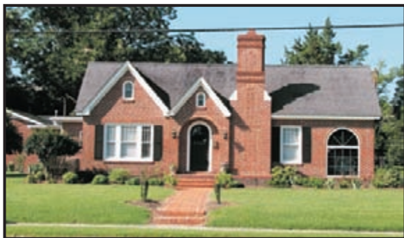
13A. Typical Masonry Minimal Traditional Type (Site 1816)
