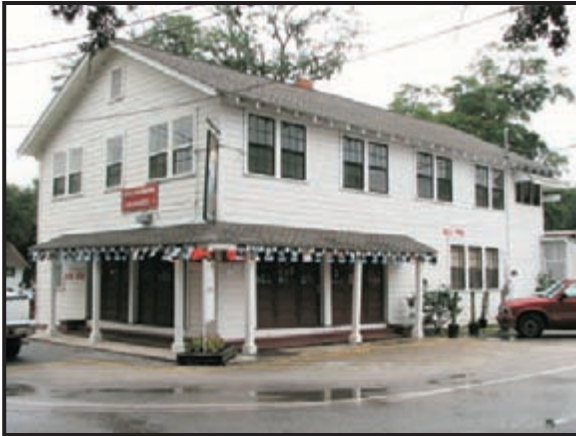
15A. Urban, Wood Frame Two Story Commercial Building (Site 0044)
