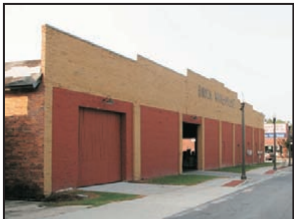
15D. Multi-Bayed Brick Warehouse (Site 1664)
