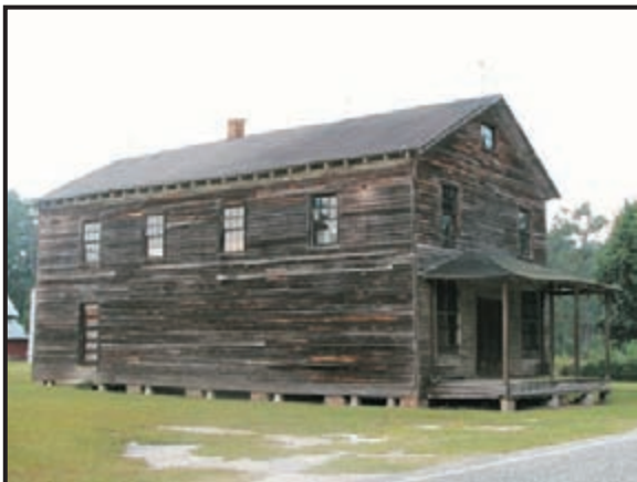
15C. Two Story, Front Gabled Wood Frame Type (Site 0253)
