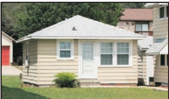
13G. Typical Example of Domestic Servants Quarters Adj. to Beach Cottage (Site 2354.01)
