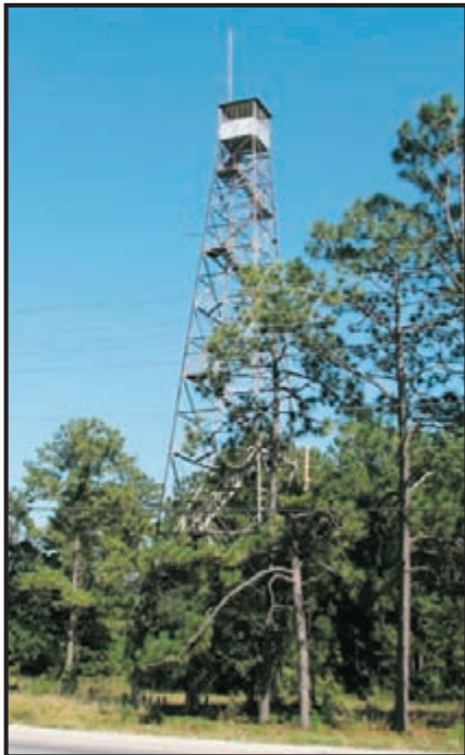
22E. Typical Metal Lookout Tower (Site 3068)
