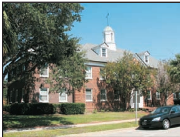
20B. Example of Civic Hipped Roof Type with Additions (Site 2754)
