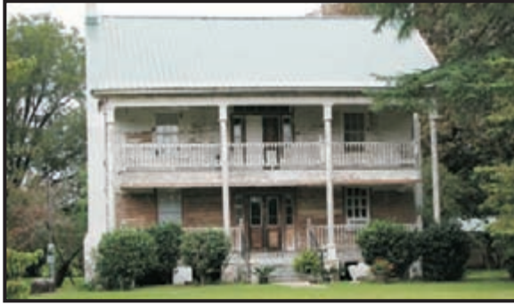
12B. Typical I-House with Two-Story Full Length Porch (Site 0288)
