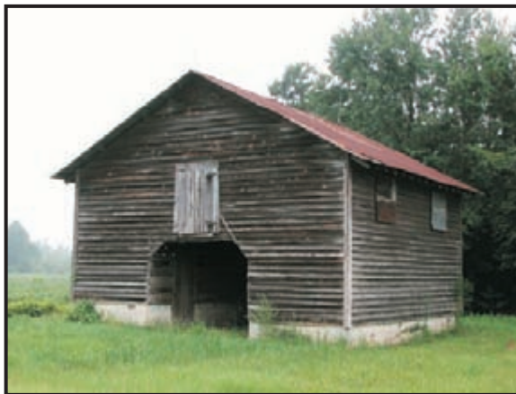
14B. Typical Transverse Double Crib Barn (Site 2002)
