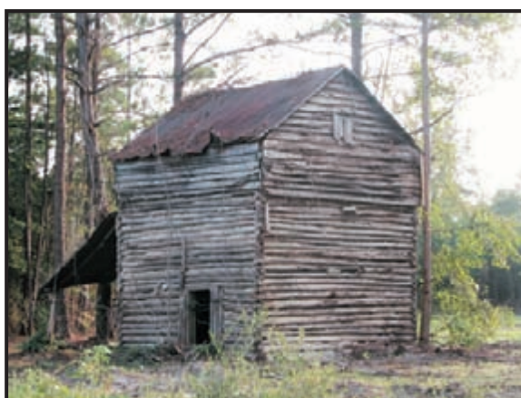
14D. Typical Saddle - Notched Log Tobacco Barn (Site 2142)
