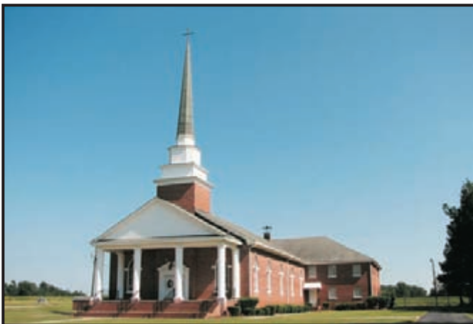
18E. Good Example of Rural, Greek Revival Type with Prominent Door Surround, Steeple and Porch (Site 3478)
