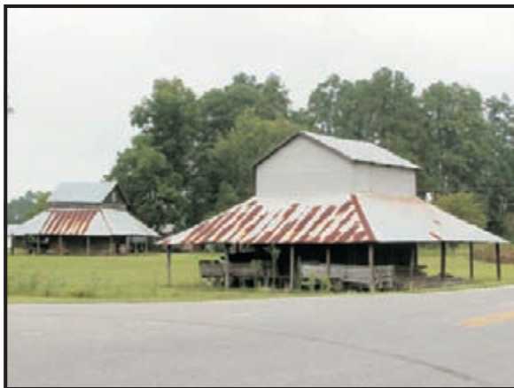
14A. Typical Tobacco Barns with Asphalt Roll Covering (Site 0343)
