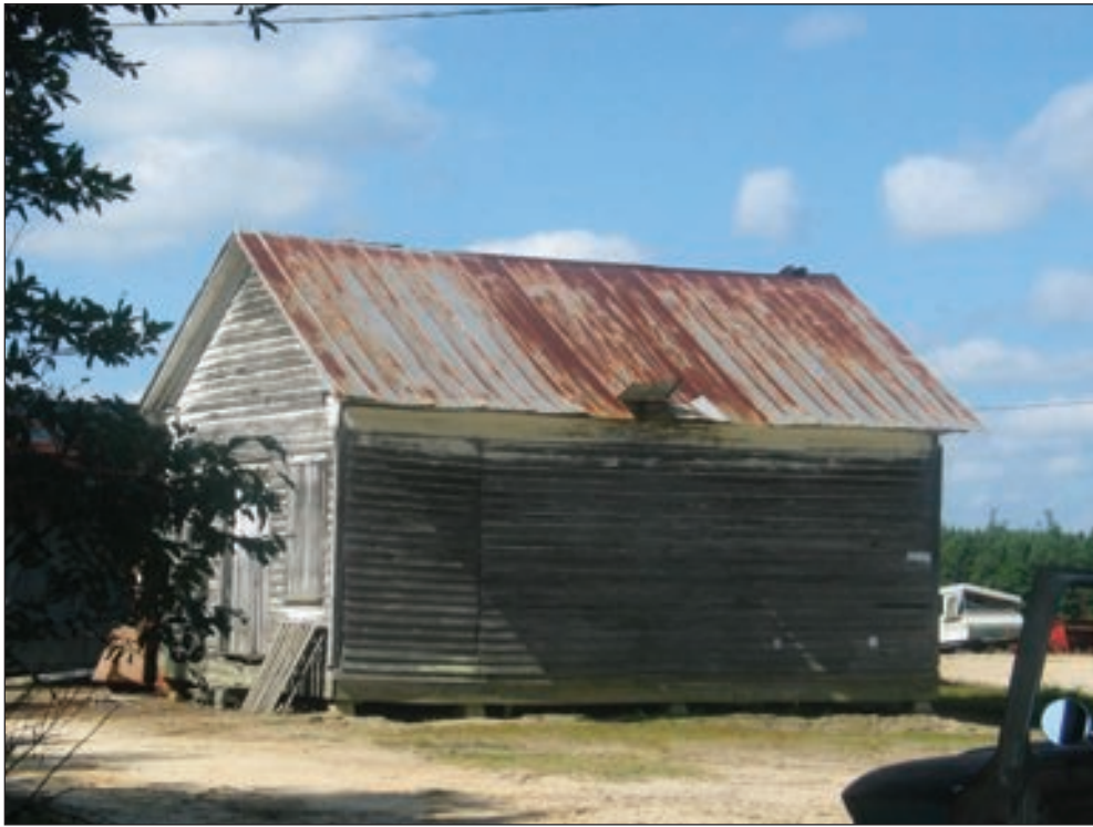
Figure 5.23 Resource 554.04, unidentified barn, view looking northeast.
