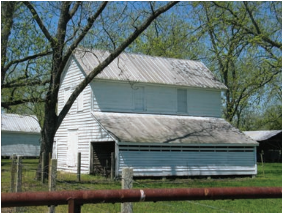
Figure 5.27 Resource 714.02, unidentified horse barn, view looking northeast.
