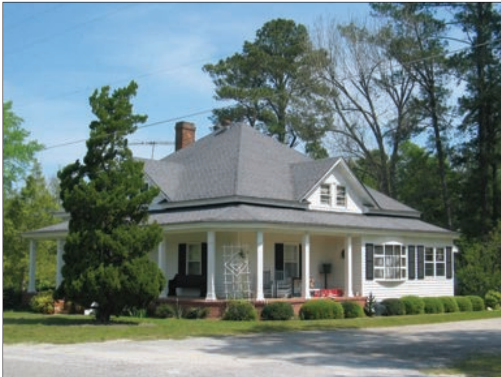
Figure 5.28 Resource 746, Kemper School, view looking south.
