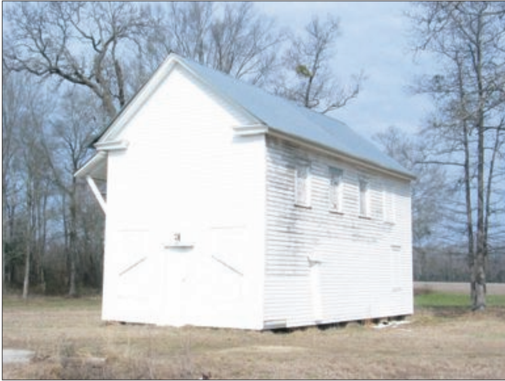
Figure 5.36 Resource 770.01, unidentified agricultural building, view looking south.
