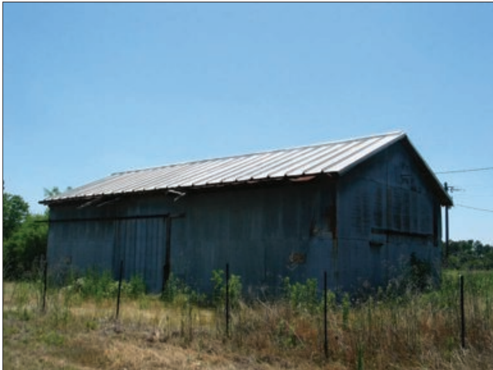
Figure 5.2 Resource 264.01, McCormick Gin/Longhorn Farm storage building, view looking north.
