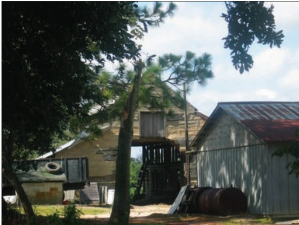
Figure 5.22 Resource 554.03, unidentified outbuilding, view looking northeast.
