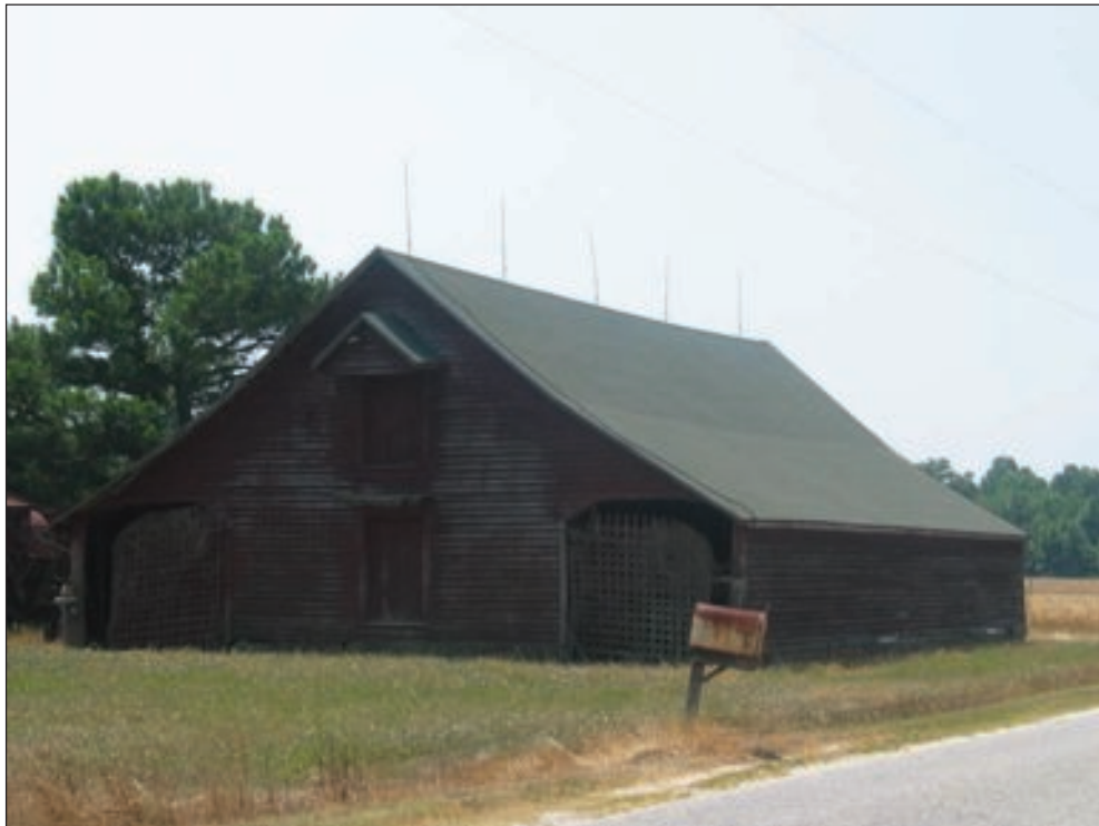
Figure 5.13 Resource 440.03, D.C. Rodgers Home (barn), view looking northeast.
