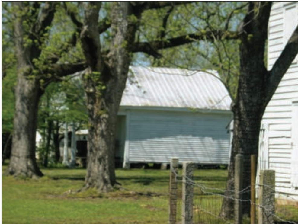
Figure 5.26 Resource 714.01, unidentified barn, view looking northeast.
