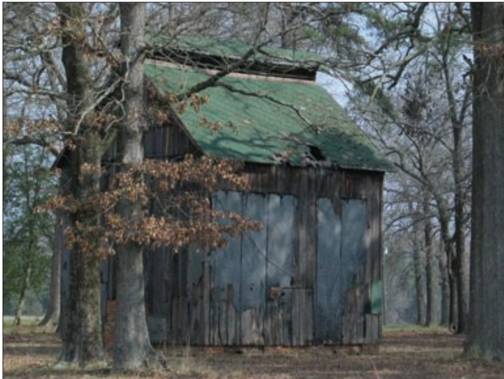
Figure 5.37 Resource 770.02, unidentified barn, view looking west.
