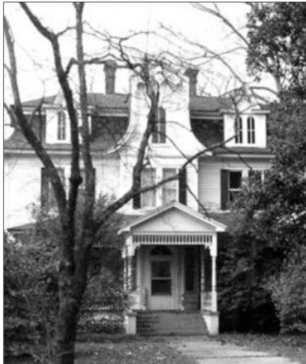
Figure 3.18 View of the left oblique of the McMillan House (courtesy of SCDAH).
