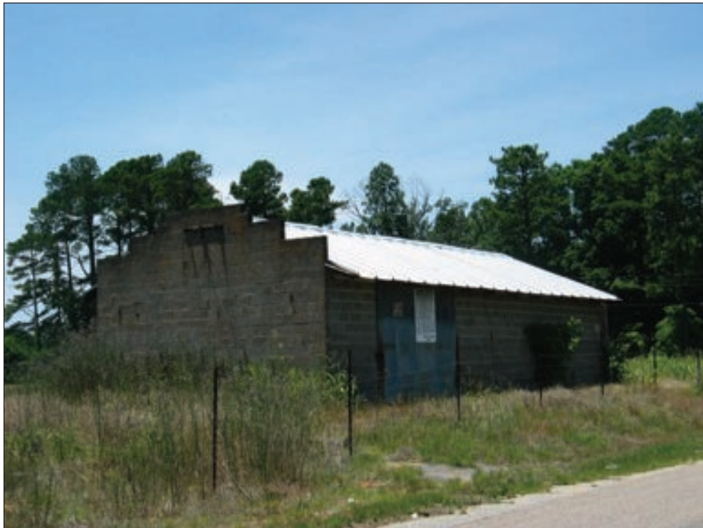
Figure 5.4 Resource 264.03, McCormick Gin/Longhorn Farm warehouse building, view looking east.
