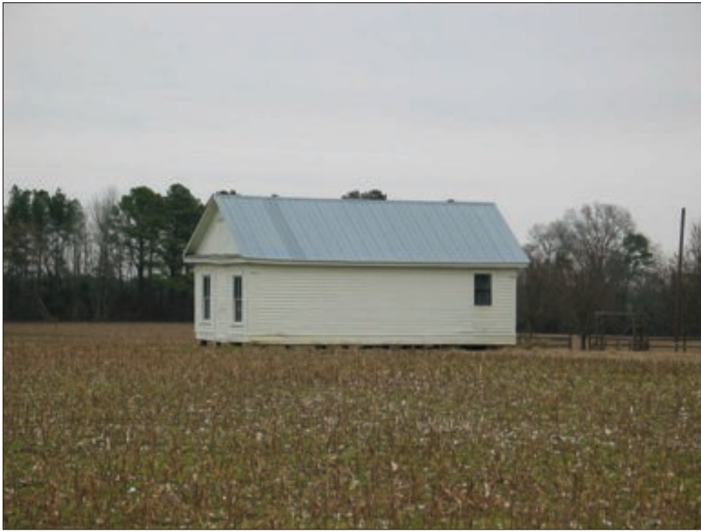
Figure 5.34 Resource 755.02, Elias Alford House (school), view looking west.
