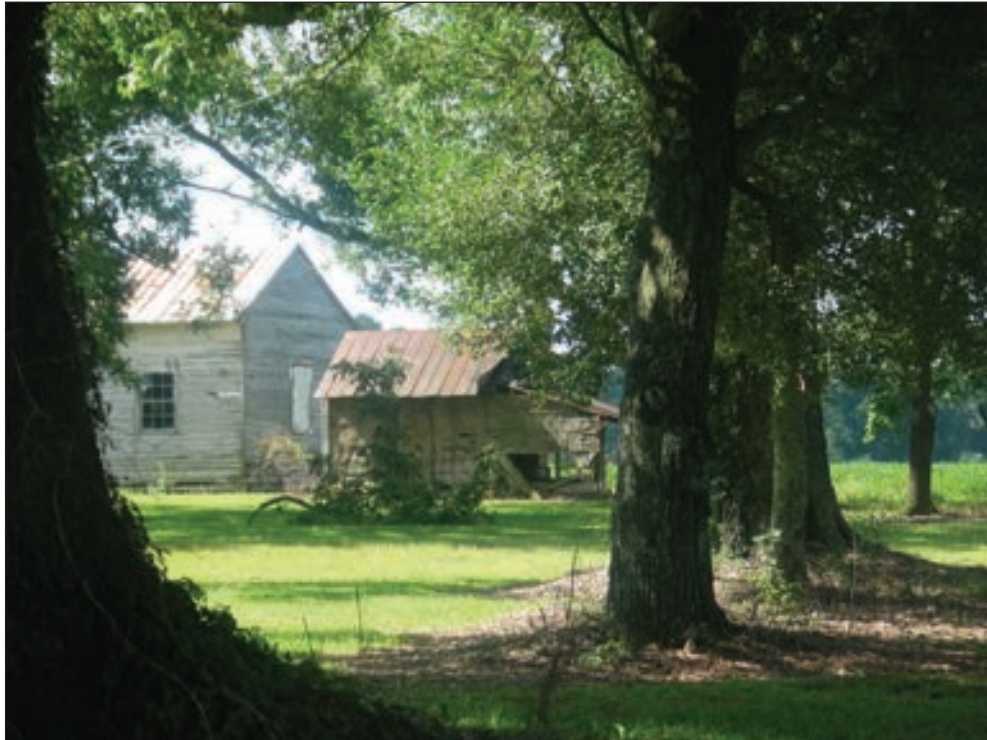
Figure 5.20 Resource 554.01, unidentified outbuilding, view looking north.
