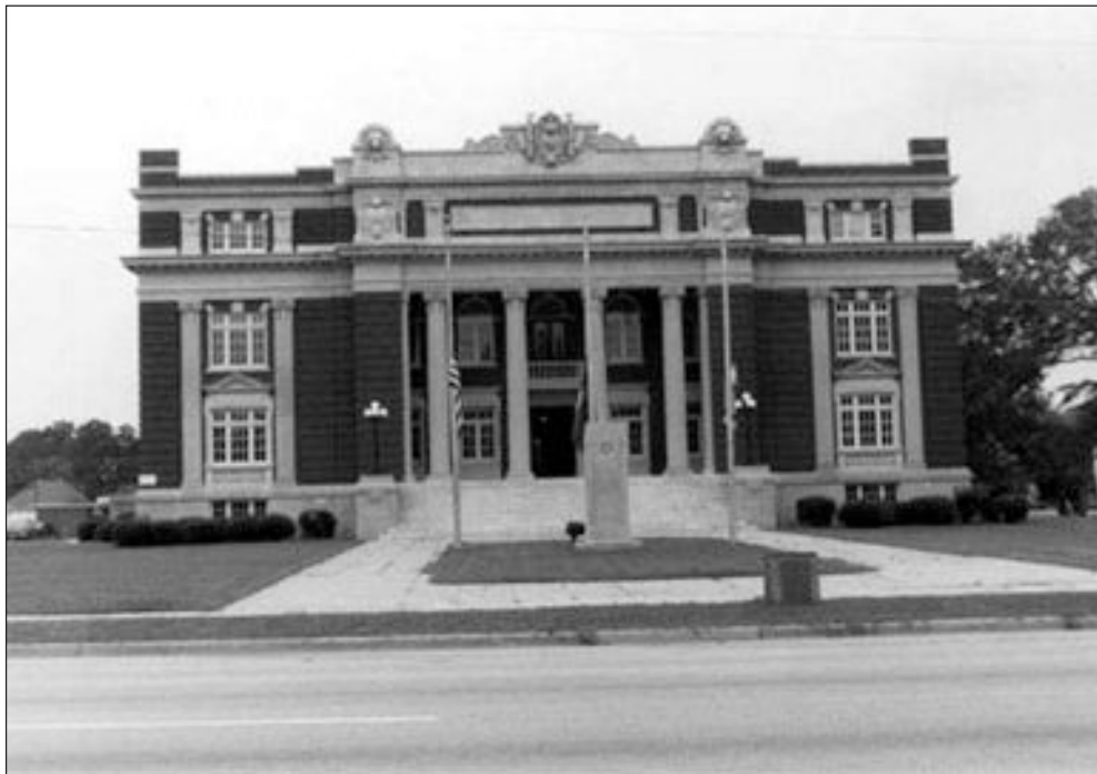
Figure 3.14 View of Dillon County Courthouse (courtesy of SCDAH).
