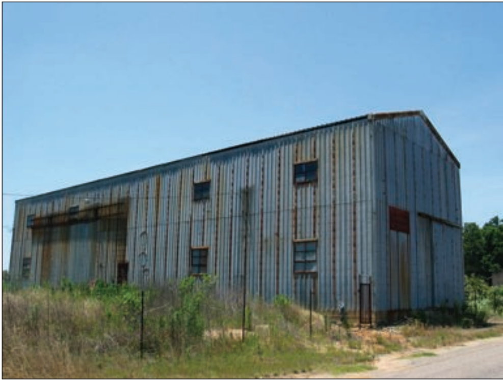
Figure 5.1 Resource 264, McCormick Gin/Longhorn Farm commercial building, view looking east.
