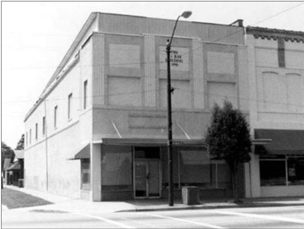
Figure 3.2 View of the McRae Building, 201 West Main Street (courtesy of SCDAH).
