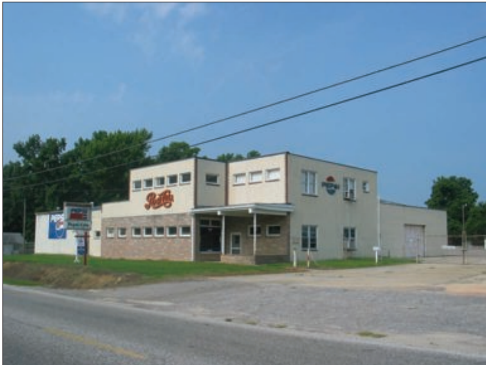
Figure 5.18 Resource 504, Pepsi-Cola Bottling Company Building, view looking northeast.
