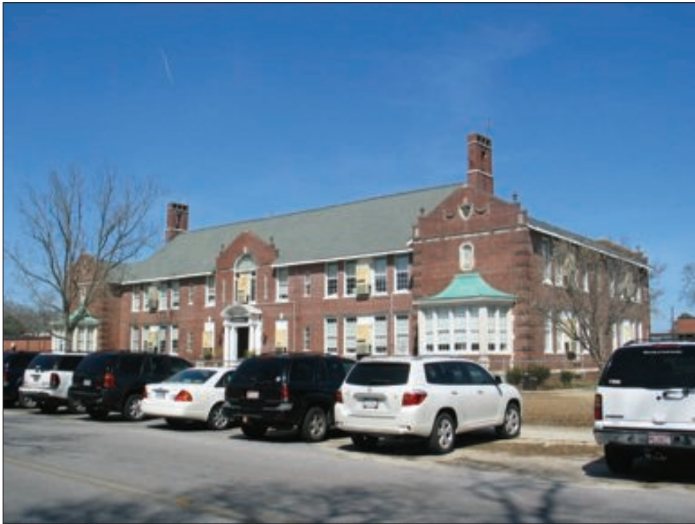
Figure 5.47 Resource 1282, East Elementary School, view looking south.
