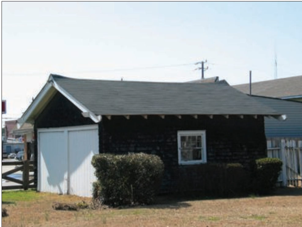
Figure 5.46 Resource 1110.01, unidentified garage, view looking northeast.
