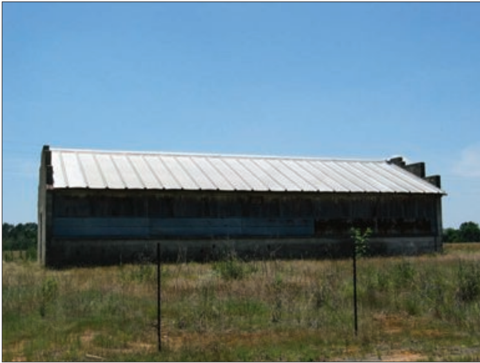
Figure 5.3 Resource 264.02, McCormick Gin/Longhorn Farm commercial building, view looking north.
