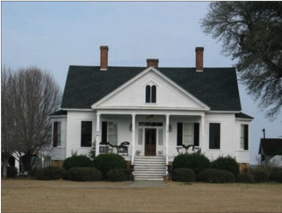
Figure 5.38 Resource 773, unidentified residence, view looking southwest.
