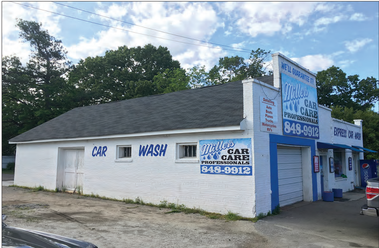
Figure 4.19 View of Resource 1316, example of a freestanding commercial building.
