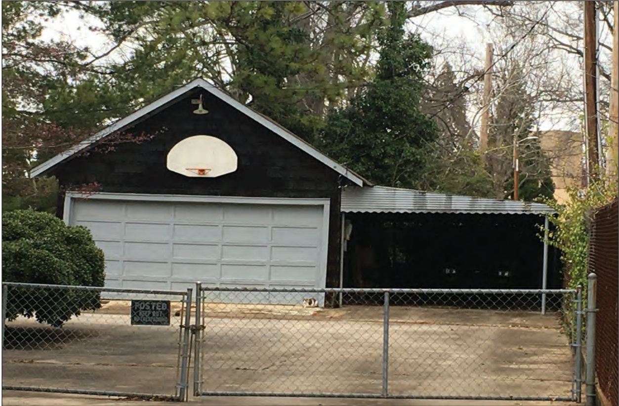
Figure 5.5 View of Resource 4008.01, south elevation.
