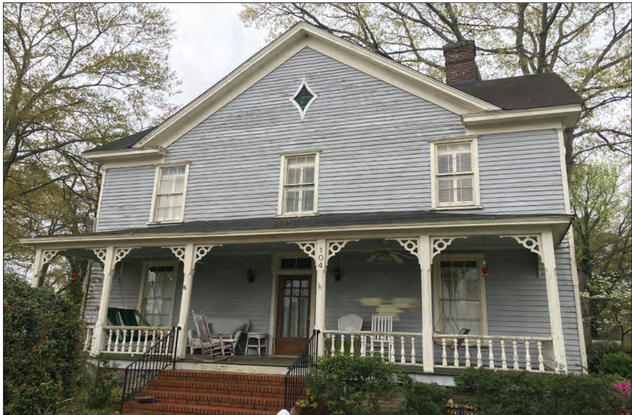
Figure 5.12 View of Resource 4421, north elevation.
