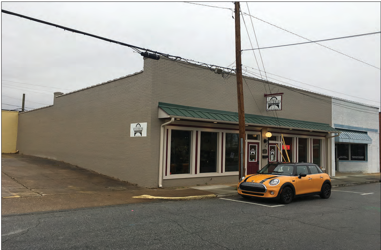
Figure 4.18 View of Resources 4002 and 4003, examples of a block of commercial buildings.
