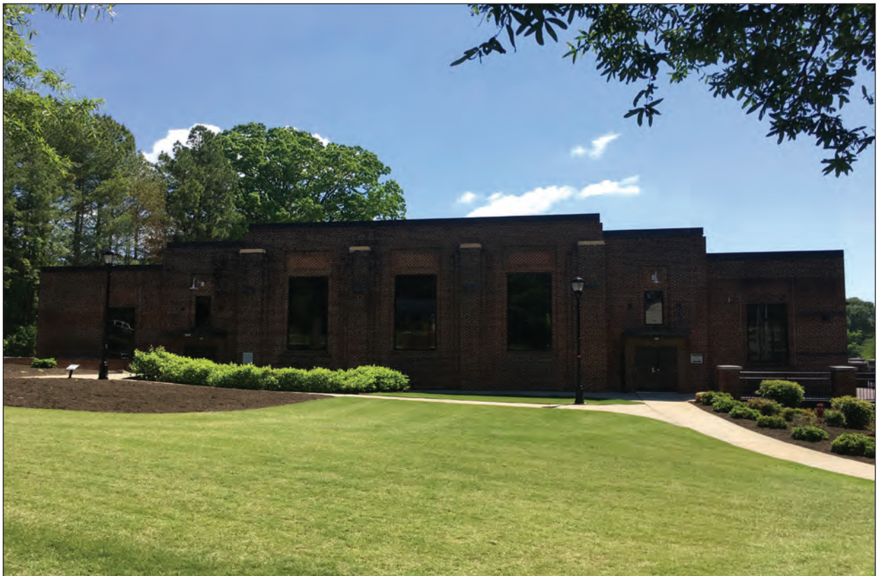
Figure 5.13 View of Resource 4634, northwest elevation.
