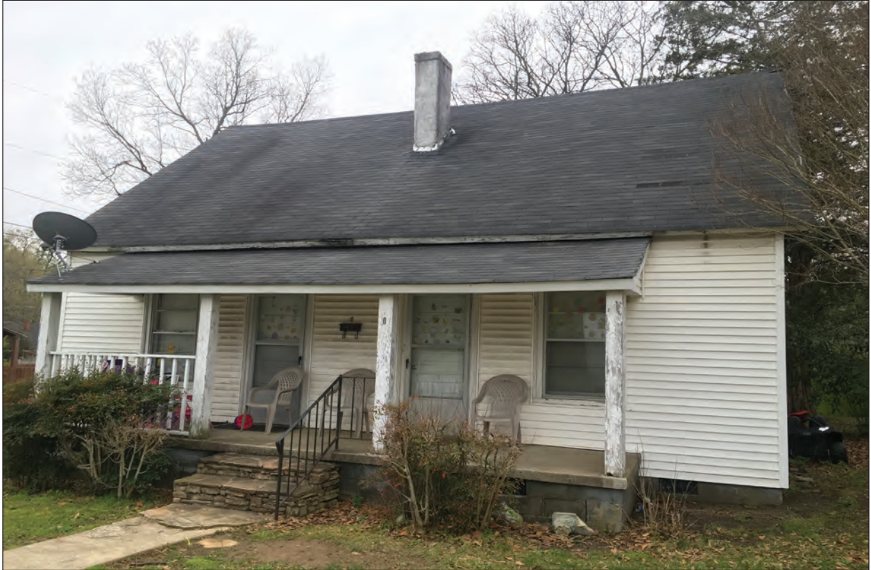
Figure 5.26 View of Resource 4239, mill house, northeast elevation.
