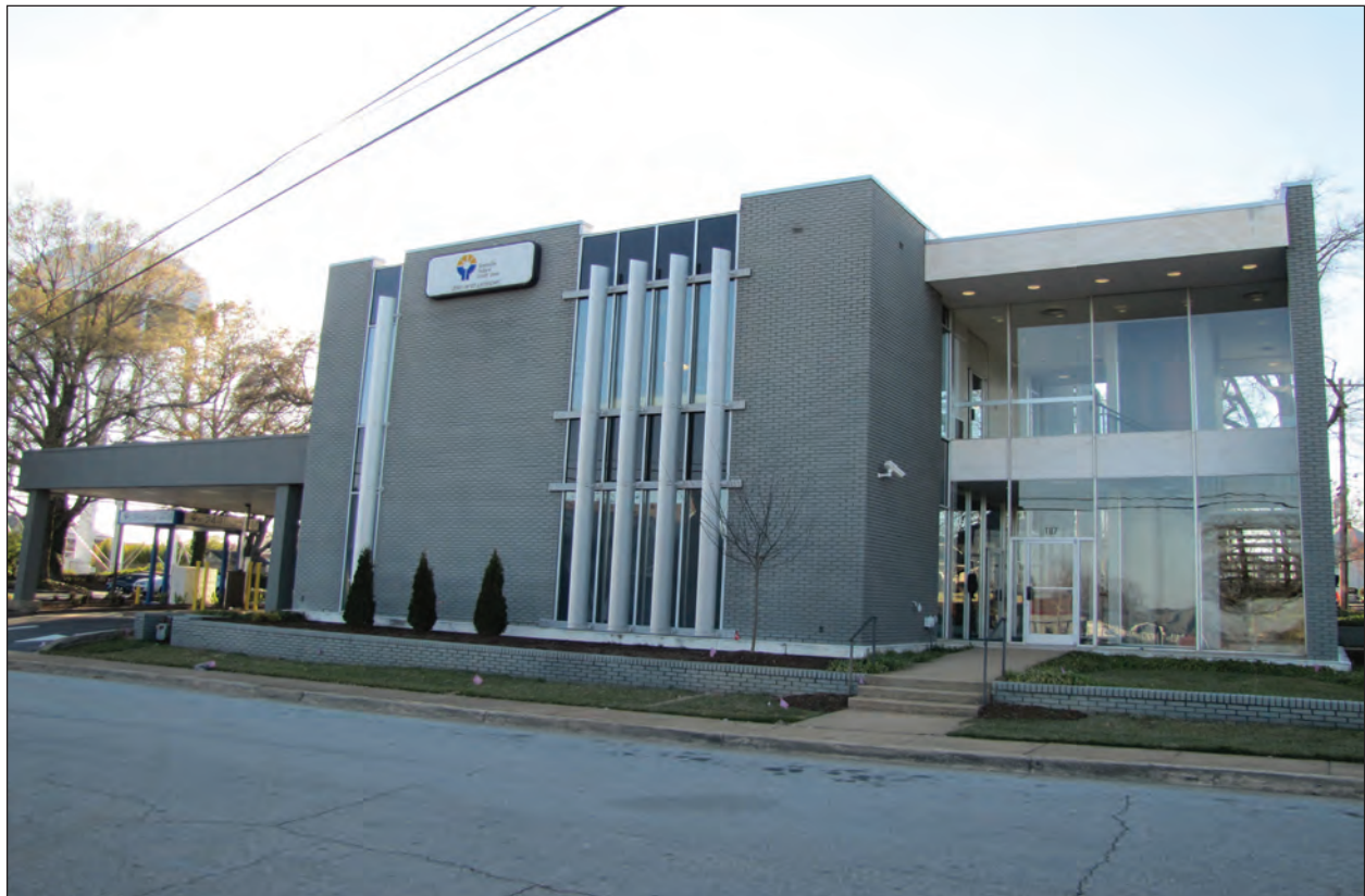
Figure 5.9 View of Resource 4084, southeast elevation.
