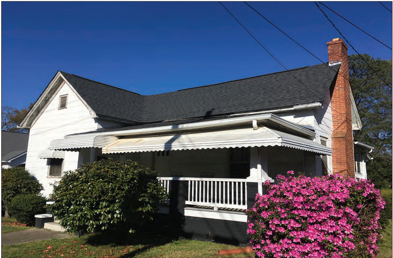
Figure 4.14 View of Resource 4356, example of a gable-front and wing house.
