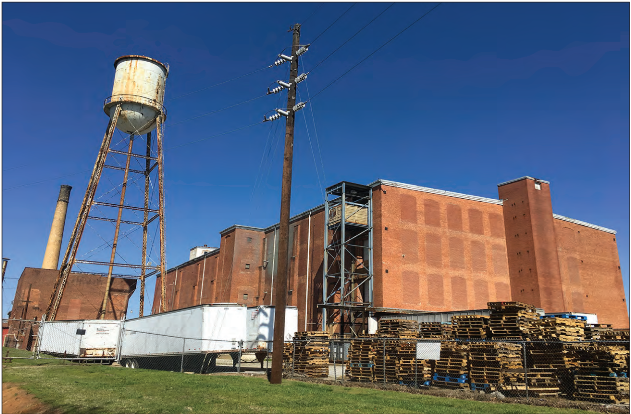
Figure 4.27 View of Resource 4365, Greer Mill complex, example of a manufacturing resource.
