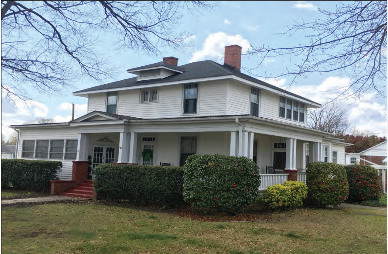
Figure 5.25 View of Resource 4155, superintendent house, northeast oblique.
