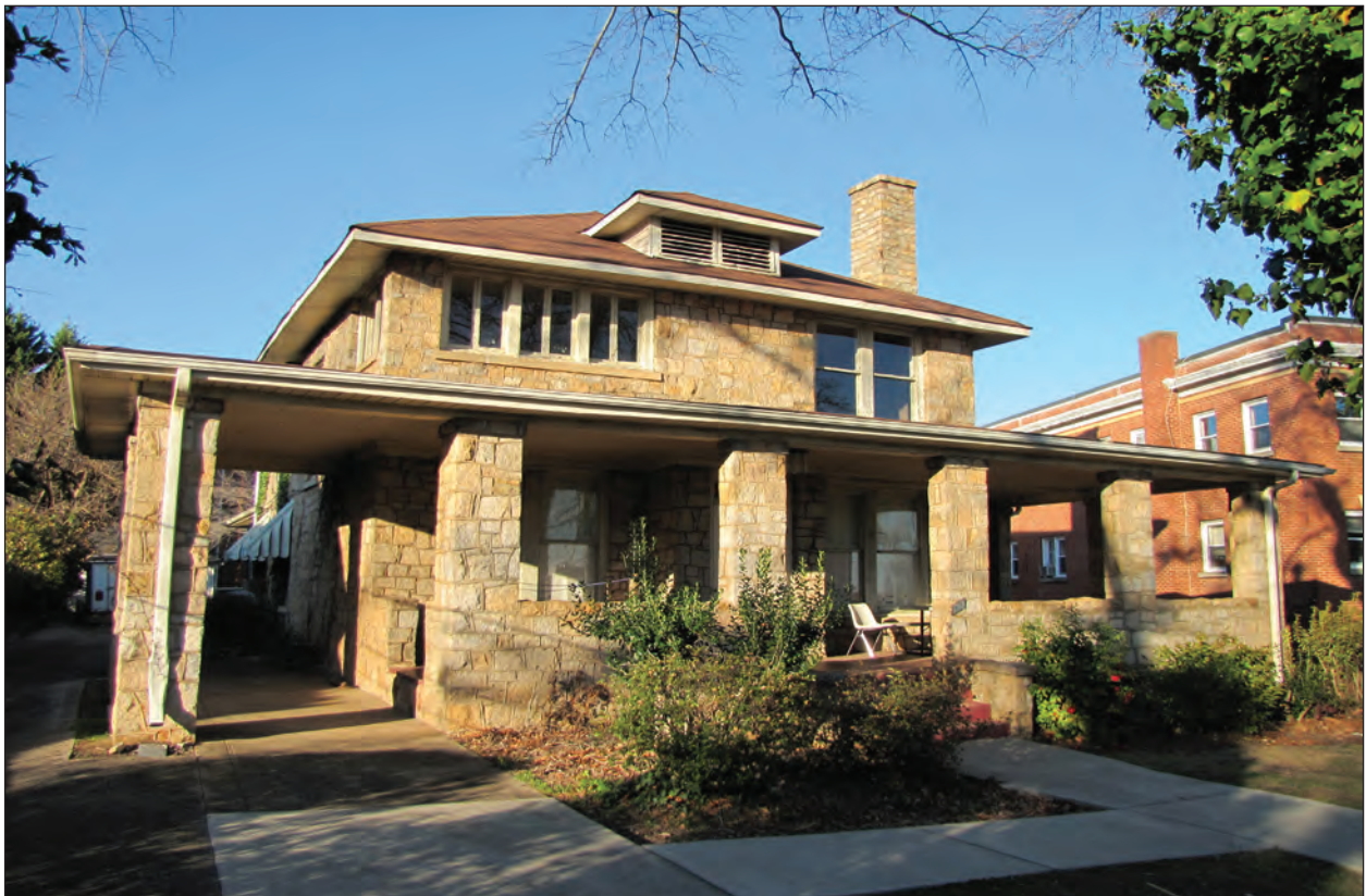
Figure 5.10 View of Resource 4085, southwest elevation..
