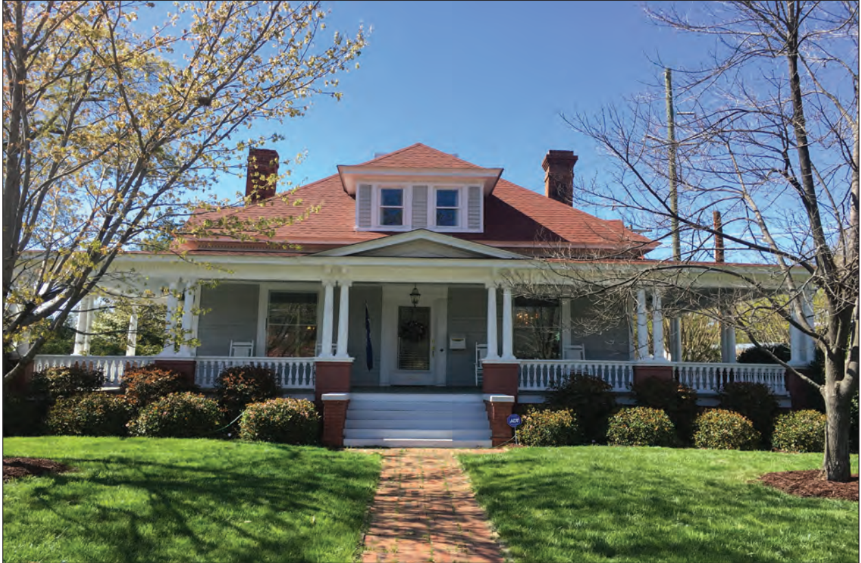
Figure 5.21 View of Resource 4343, southeast elevation.
