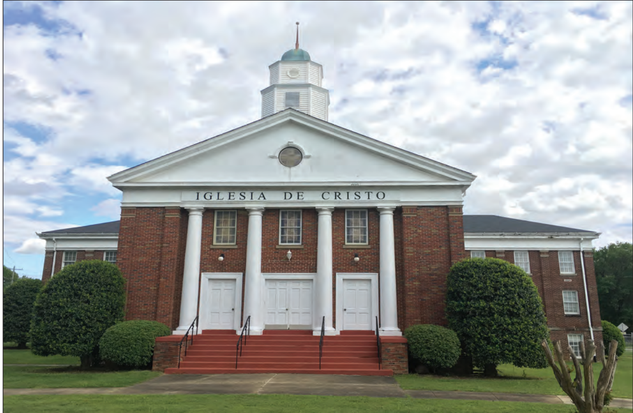
Figure 5.2 View of Resource 1315, northwest elevation.
