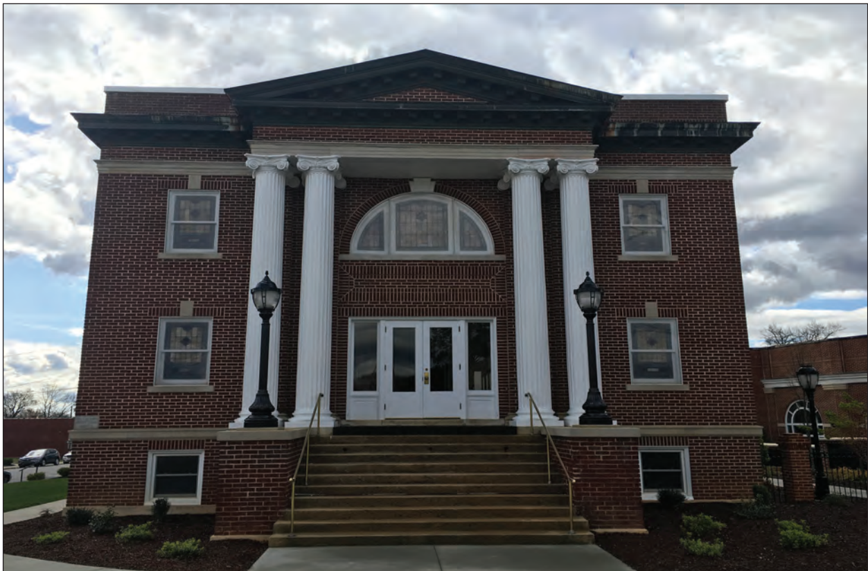
Figure 5.3 View of Resource 4006, north elevation.
