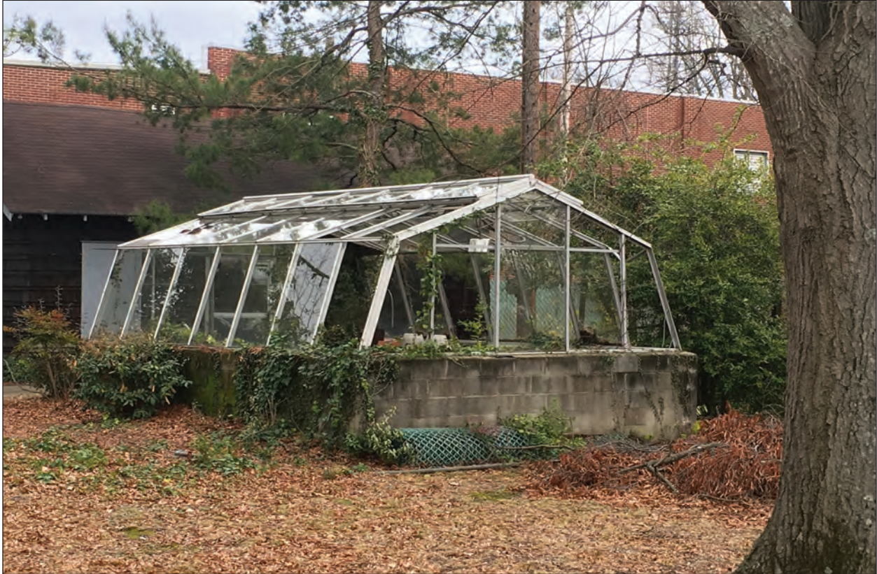
Figure 5.6 View of Resource 4008.02, northwest oblique.
