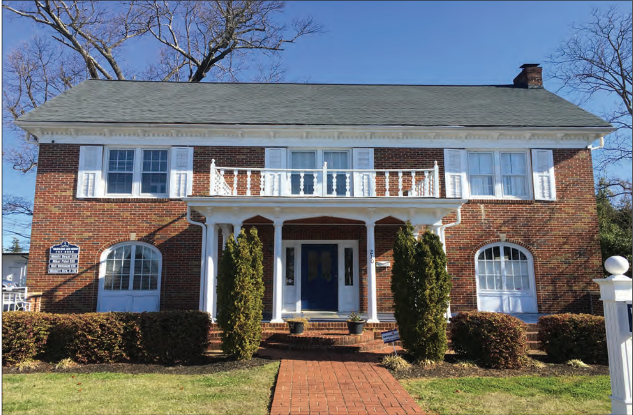
Figure 5.19 View of Resource 4060, southwest elevation.
