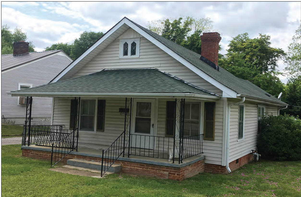
Figure 4.12 View of Resource 1218, example of a front-gable house.
