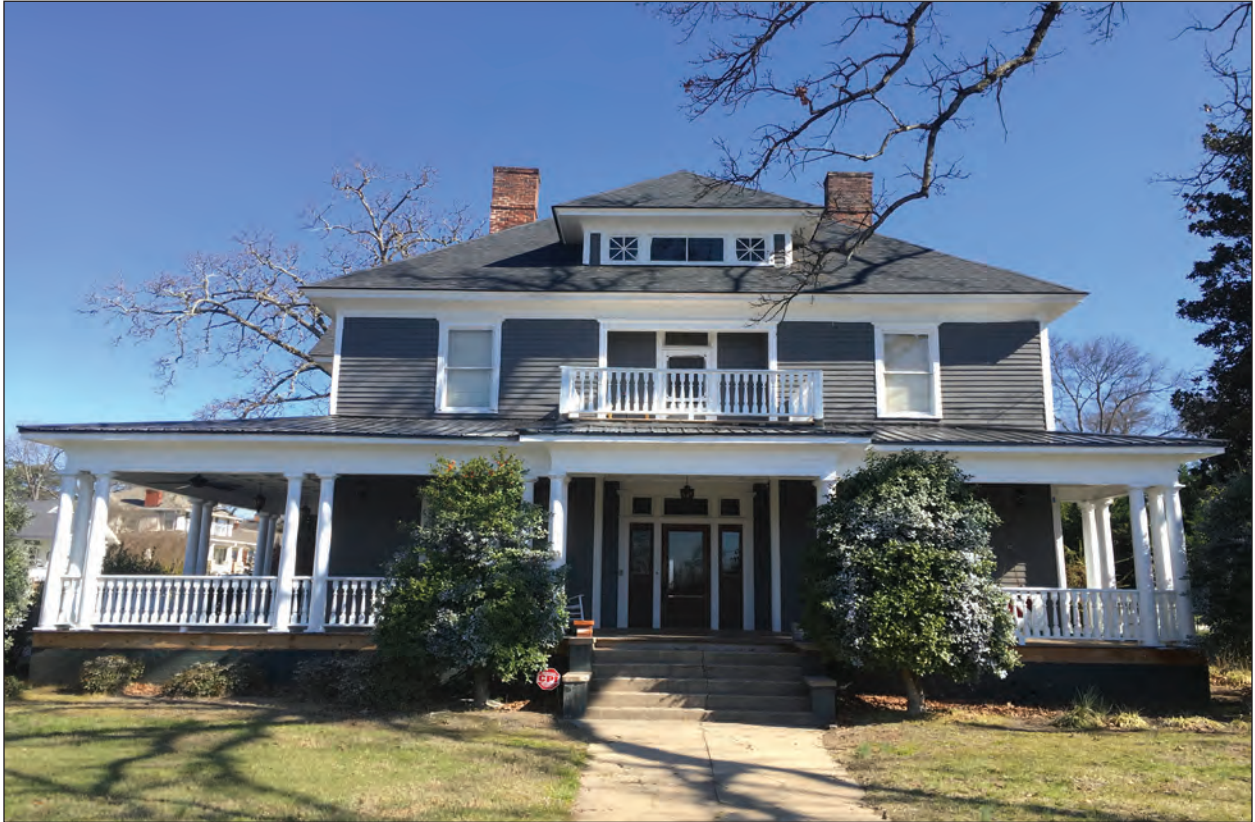
Figure 5.20 View of Resource 4061, southwest elevation.
