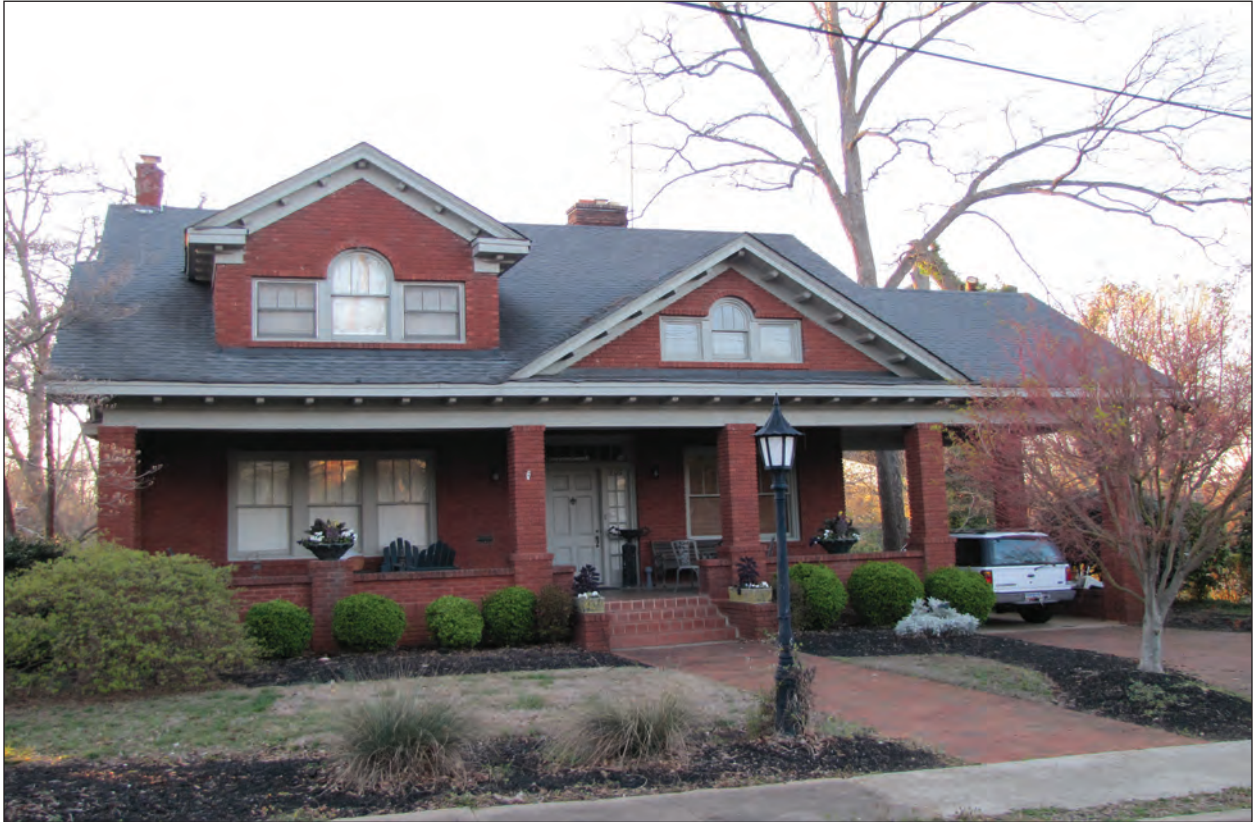
Figure 5.16 View of Resource 4042, southeast elevation.
