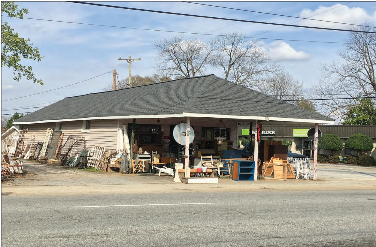
Figure 4.26 View of Resource 4130, example of a folk form transportation building.
