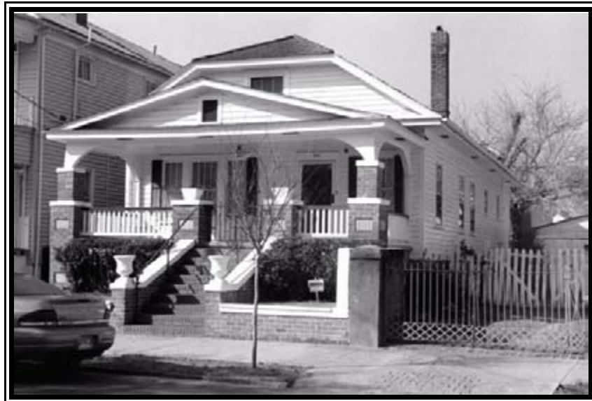
Figure 62. 541 Rutledge Avenue (Resource 2249), northeast elevation.
