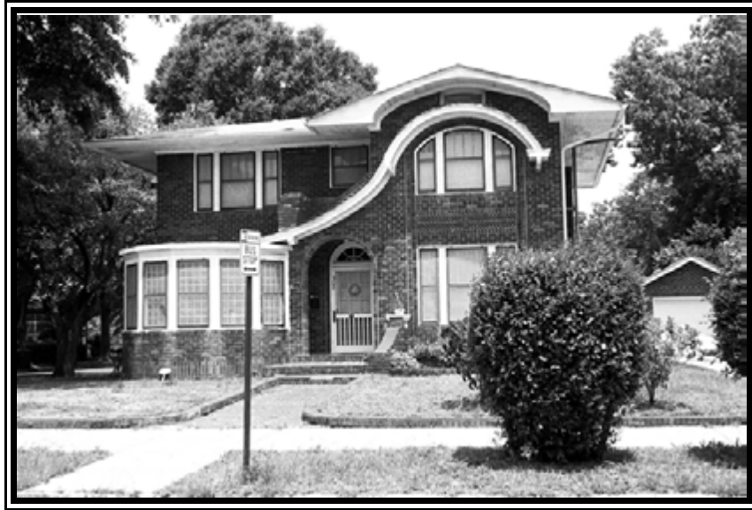
Figure 83. 308 Grove Street (Resource 4091), south elevation.
