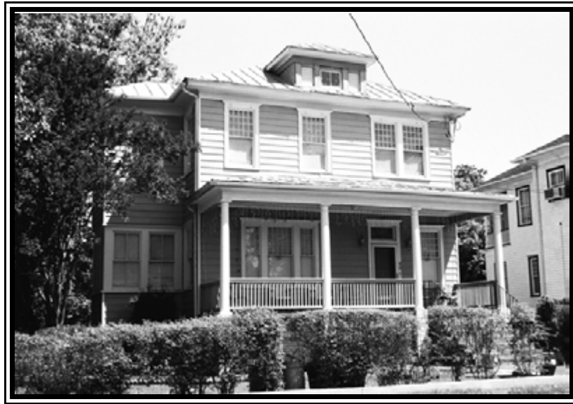
Figure 79. 60 Poplar Street (Resource 3154), southwest elevation.
