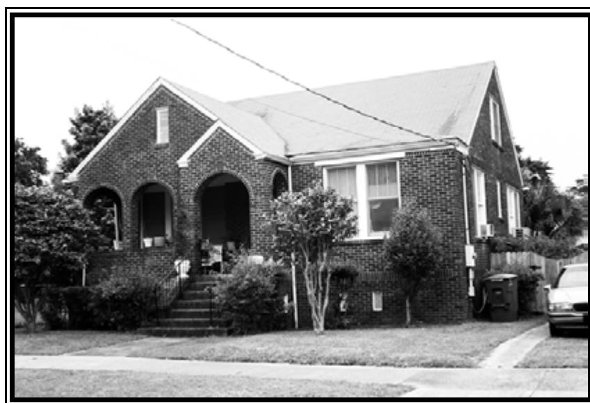
Figure 47. Resource 3566, southwest elevation, an example of the Minimal Traditional style.
