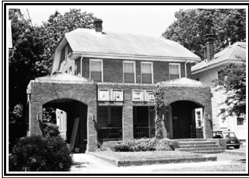
Figure 77. 809 Rutledge Avenue (Resource 3062), southeast elevation.
