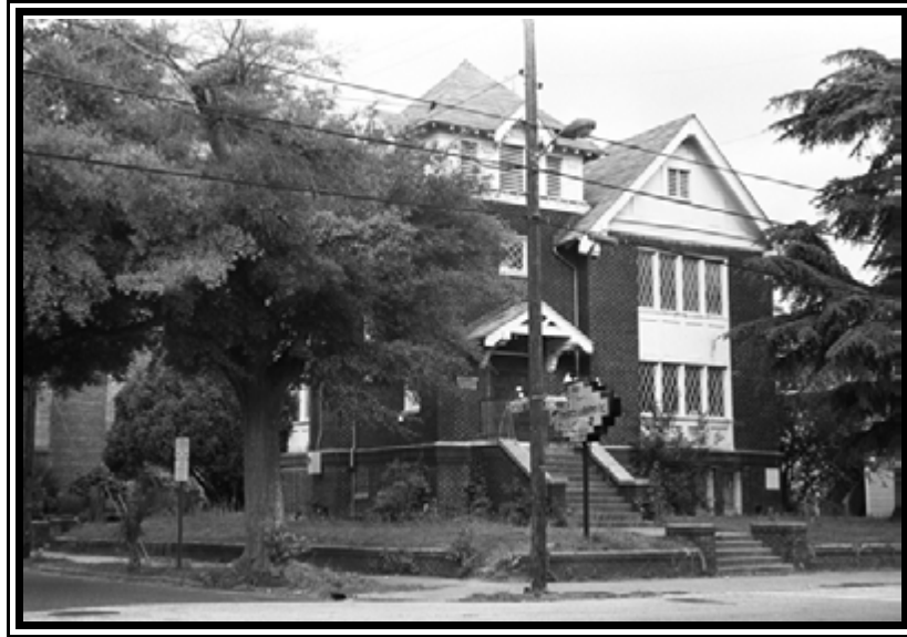
Figure 75. 981 King Street (Resource 2967), southeast elevation.
