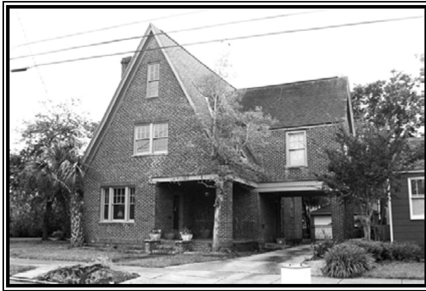
Figure 82. 187 Grove Street (Resource 3932), northeast elevation.
