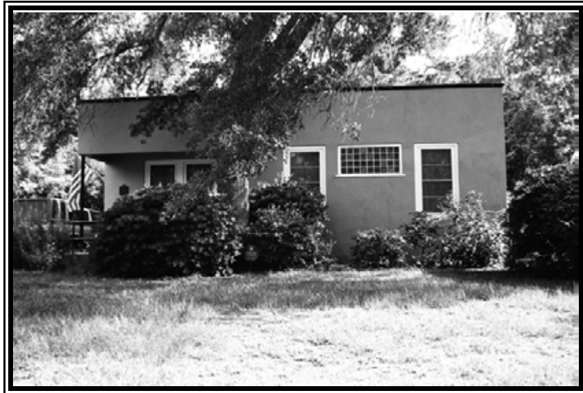
Figure 46. Resource 3503, south elevation, and example of the International style.
