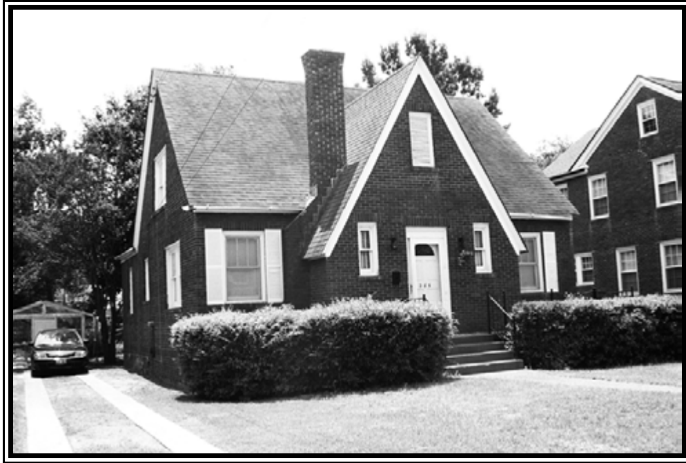
Figure 39. Resource 4098, northwest elevation, showing elements of the Tudor Revival style.
