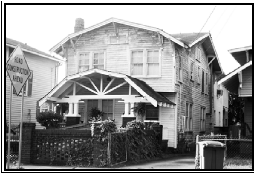
Figure 80. 31 Cypress Street (Resource 3212), northwest elevation.
