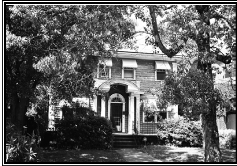
Figure 76. 807 Rutledge Avenue (Resource 3061), east elevation.
