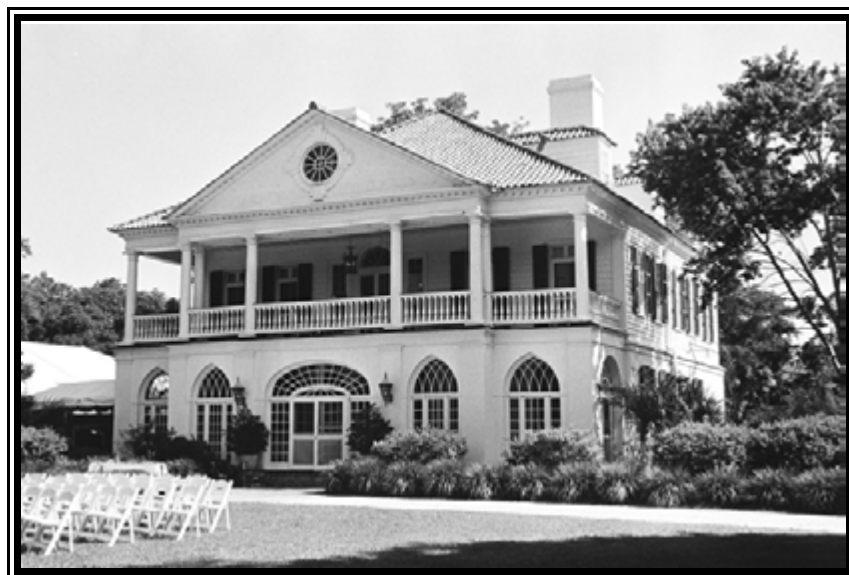
Figure 30. Lowndes Grove (Resource 0073.00), southeast elevation, an example of the Federal style.
