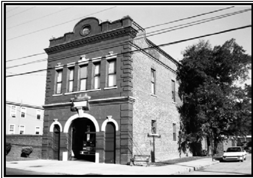
Figure 51. Engine Number 8 Building (Resource 2888), southeast elevation.
