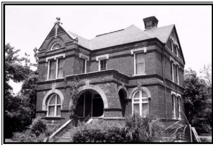
Figure 34. Enston Home Cottage #1 (Resource 0075.01), northeast elevation, an example of the Romanesque Revival style.
