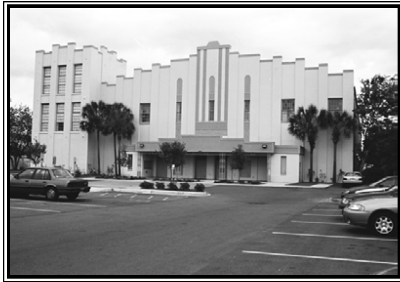
Figure 53. County Hall (Resource 2964), southwest elevation.
