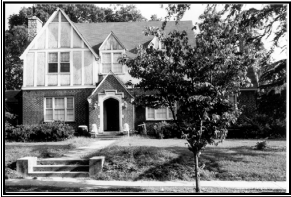
Figure 19. An example of Tudor Revival style, site 0375, 900 East Main St.
