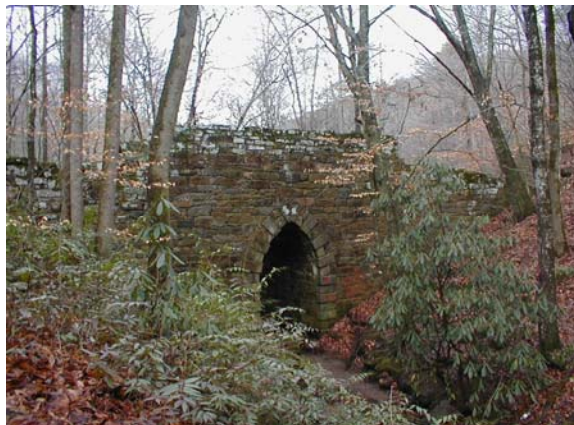
Poinsett Bridge, Greenville County, Heritage Trust site.
