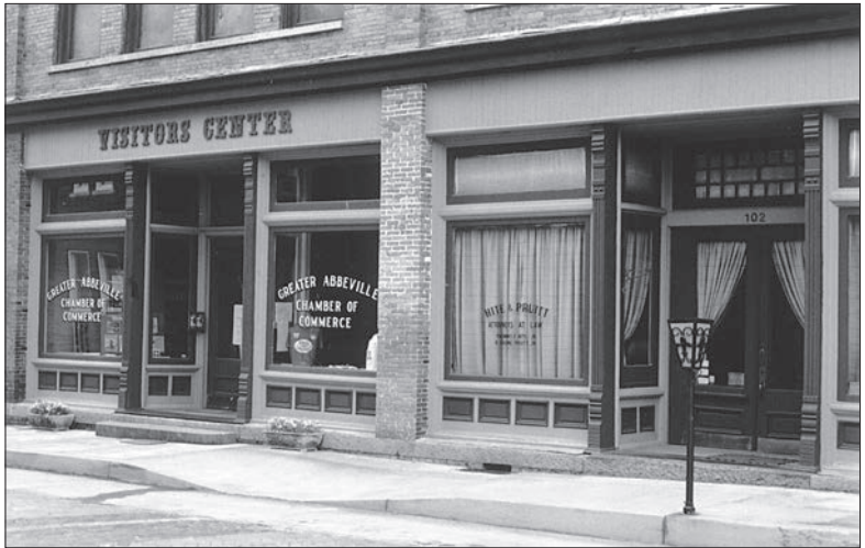
LEFT: This wood storefront has all the classic elements: a paneled bulkhead, large paired and glazed entrance doors, large display windows, and transoms over the display windows. Note that the storeroom ceiling is so high there is room for an unusual double transom over the entrance doors. RIGHT: These late-19th century storefronts combine stone, wood, cast iron, and glass in a lively and visually interesting composition. In these examples, large signboards are placed above the storefronts and below an intermediate cornice.
