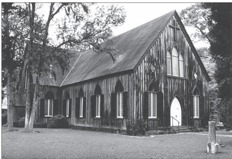
In South Carolina most Gothic Revival buildings were churches like the Church of the Cross, in Bluffton, Beaufort County.
