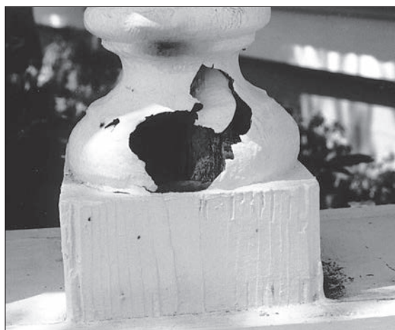
CLOCKWISE LEFT TO RIGHT: Proper surface preparation is essential to a successful paint job on a wood-sided building. Sometimes it is necessary to remove earlier paint layers if the build-up is so great that it cannot provide a sound surface for the new paint. / This is a close-up view of severe termite damage. The tunnels they eat through the wood are clearly visible, as is the waste material, known as frass, that they leave behind. / Termite damage often is not visible on the surface of the wood element. This baluster has lost all its physical integrity, having been eaten away from within. The damage was not apparent, however, until a tool pressed against the surface broke through the thin shell of paint and wood that the termites left behind.
