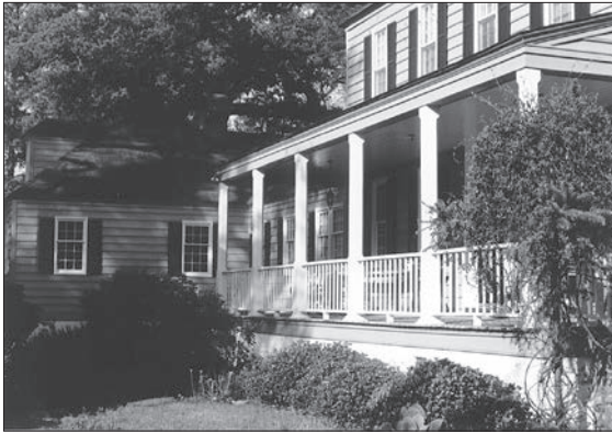
LEFT: Additions should be located so that they do not interfere with the original form and setting of the main building. Materials, details, and overall form should also be compatible with the historic building. RIGHT: The design of these incompatible doors and windows was not based on the design of the historic building.
