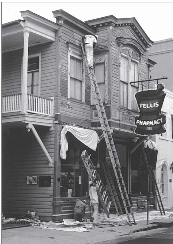
CLOCKWISE LEFT TO RIGHT: Proper surface preparation is essential to a successful paint job on a wood-sided building. Sometimes it is necessary to remove earlier paint layers if the build-up is so great that it cannot provide a sound surface for the new paint. / This is a close-up view of severe termite damage. The tunnels they eat through the wood are clearly visible, as is the waste material, known as frass, that they leave behind. / Termite damage often is not visible on the surface of the wood element. This baluster has lost all its physical integrity, having been eaten away from within. The damage was not apparent, however, until a tool pressed against the surface broke through the thin shell of paint and wood that the termites left behind.
