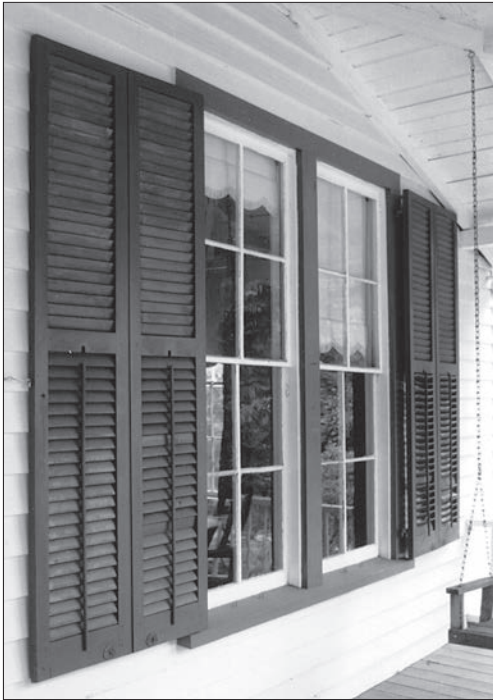
LEFT: Working shutters and a sheltering porch roof can significantly cut down on summer heat gain in a house. The shutters have louvers to provide air flow while they are closed, and the porch keeps the sun from shining directly into the interior. ABOVE: Plugs like these are evidence that insulation has been pumped or blown into a cavity wall, probably without a proper vapor barrier. The potential for trapping moisture in the insulation is very high in such cases and can lead to serious dry rot damage to the structure.
