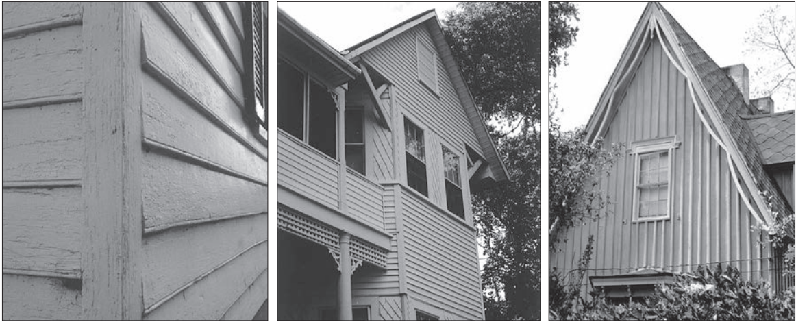
LEFT TO RIGHT: Historic wood siding can have a great deal of character and visual quality, as can be seen in this example of beaded-edge beveled siding. / Late 19th century buildings often combined various kinds of wood siding. This example has both beveled and shingle siding, and in addition has decorative elements such as latticework, columns, and brackets. / Board-and-batten siding was very popular in the 19th century, especially in mid-century examples of the Gothic Revival style. Battens sometimes were rectangular, but often they were beveled or profiled. Note the unusual open bargeboard treatment of this board-and-batten house.
