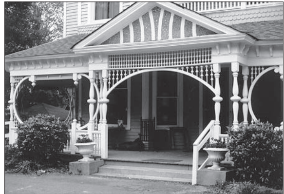
LEFT: Wood elements were the earliest kind of ornamentation and are still the most common on South Carolina buildings. This building combines an accentuated pediment, window trim, small cornice brackets, and drop finials — all of wood — in a pleasing overall composition. RIGHT: Many late-19th century buildings had elaborate ornamentation made of wood, as in this excellent example. Retention, repair, and regular maintenance of such elements is extremely important in preserving a building's character.
