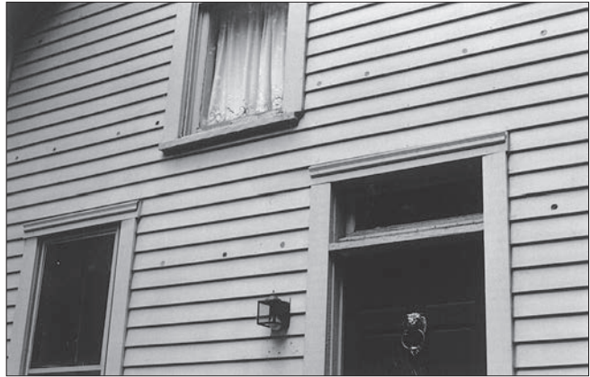
LEFT: Working shutters and a sheltering porch roof can significantly cut down on summer heat gain in a house. The shutters have louvers to provide air flow while they are closed, and the porch keeps the sun from shining directly into the interior. ABOVE: Plugs like these are evidence that insulation has been pumped or blown into a cavity wall, probably without a proper vapor barrier. The potential for trapping moisture in the insulation is very high in such cases and can lead to serious dry rot damage to the structure.
