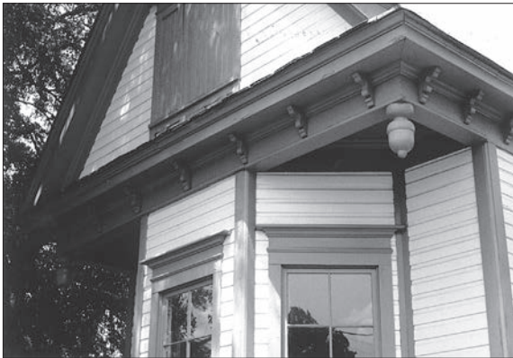
LEFT: Wood elements were the earliest kind of ornamentation and are still the most common on South Carolina buildings. This building combines an accentuated pediment, window trim, small cornice brackets, and drop finials — all of wood — in a pleasing overall composition. RIGHT: Many late-19th century buildings had elaborate ornamentation made of wood, as in this excellent example. Retention, repair, and regular maintenance of such elements is extremely important in preserving a building's character.
