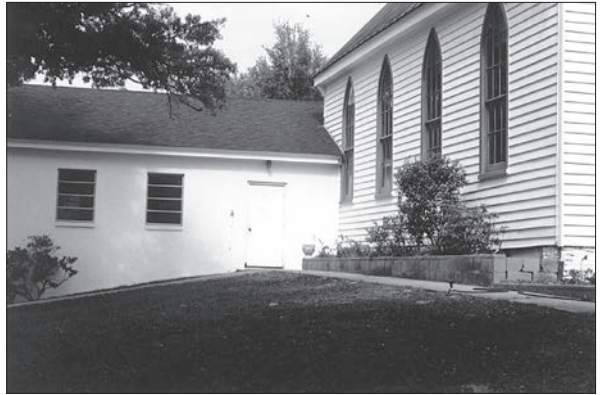
LEFT: Additions should be located so that they do not interfere with the original form and setting of the main building. Materials, details, and overall form should also be compatible with the historic building. RIGHT: The design of these incompatible doors and windows was not based on the design of the historic building.
