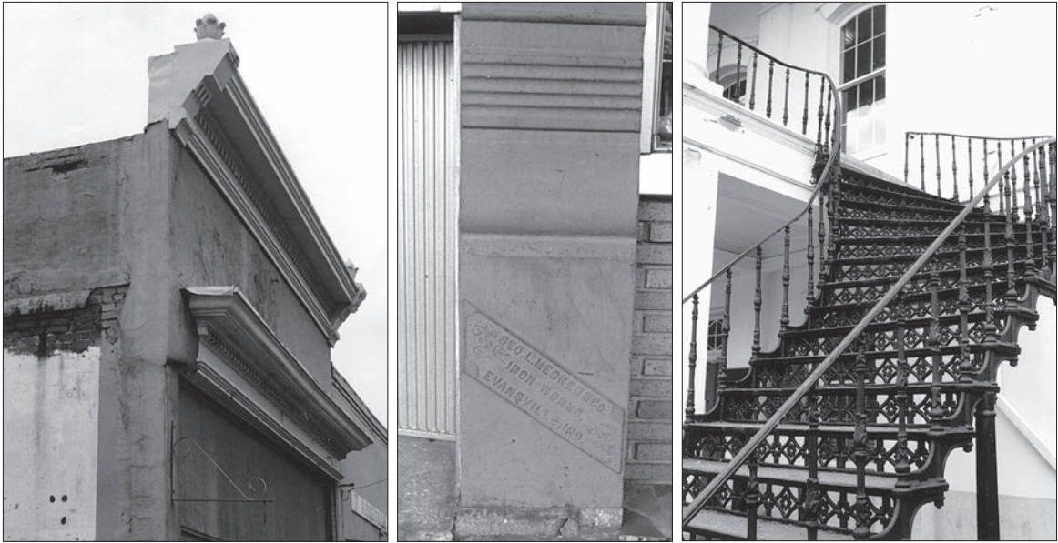
LEFT TO RIGHT: A very popular use of architectural metal was on commercial buildings, where pressed sheet metal was widely used to form building and storefront cornices. Note how much character this simple treatment gives to a fairly modest commercial structure. / Cast iron storefronts were readily available in the late 19th and early 20th centuries. George L. Mesher & Co. of Evansville, Indiana, shipped thousands of such fronts all over the United States. They could be bought by the running foot to fit any building and assembled like large kits. / Another kind of architectural metal common in South Carolina is cast iron in the form of stairs, railings, and fences. This well-designed and well-preserved example shows the level of detail that could be achieved with this material.
