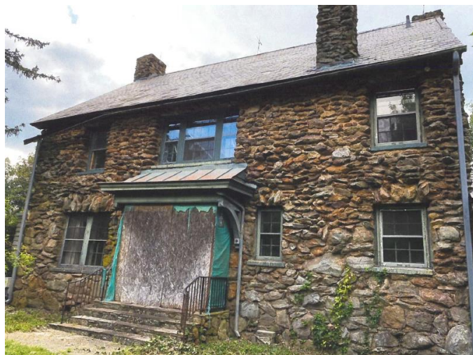
Pre-rehabilitation photograph of the residence. Image courtesy of Preservation South, Inc.
