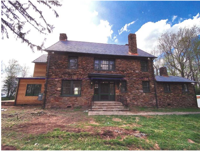
Post-rehabilitation photograph of the residence. Image courtesy of Preservation South, Inc.
